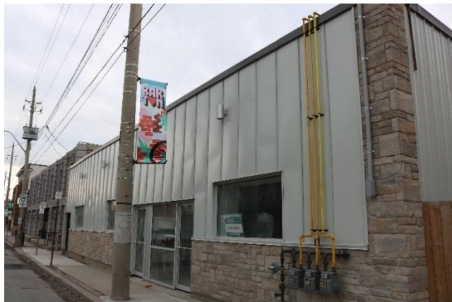
440 Barton Street East, Hamilton-After Renovations (Source: CDSB Section)
