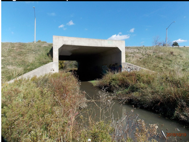
Figure 21: Example of a Culvert
