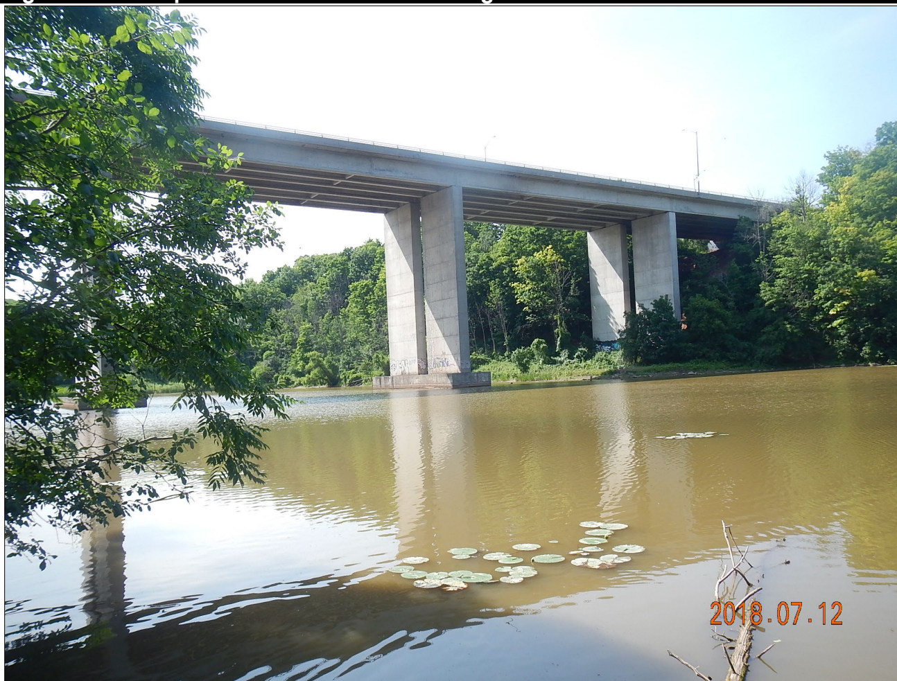
Figure 19: Example of an I-Beam / Girder Bridge on York Blvd
