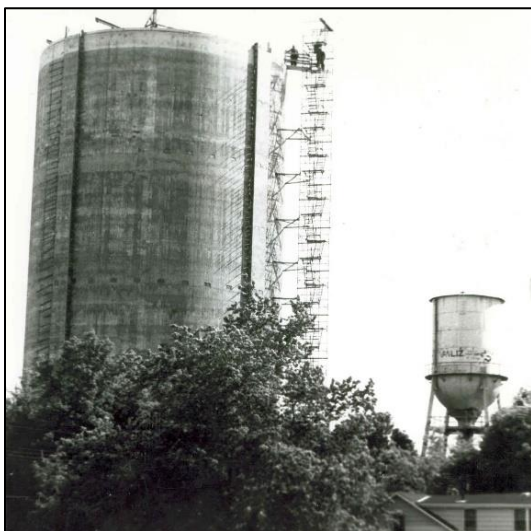
Figure 47: New water tower under construction, c. 1977 (Flamborough Archives, BW 1508)
