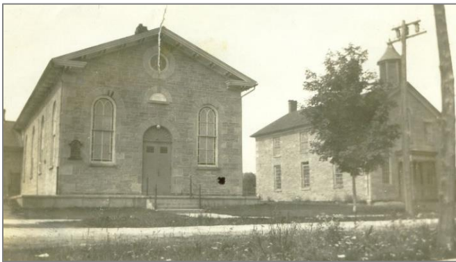
Figure 16: Methodist Church (left) and East Flamborough Township Hall (right) on Mill Street North circa 1915-1920 (Flamborough Archives, BW406)
