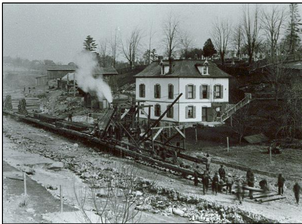
Figure 32: Railway under construction by Canadian Pacific Railway north of Dundas Street Bridge circa 1911 (Flamborough Archives, BW 94, Will Reid Collection)
