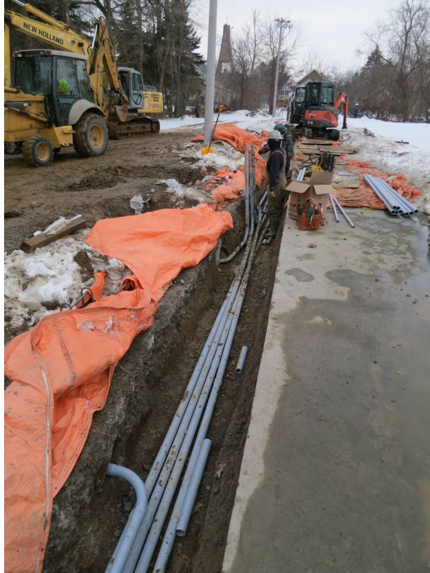
60 - March 1st. Installing electrical conduits on the south side of the courts.
