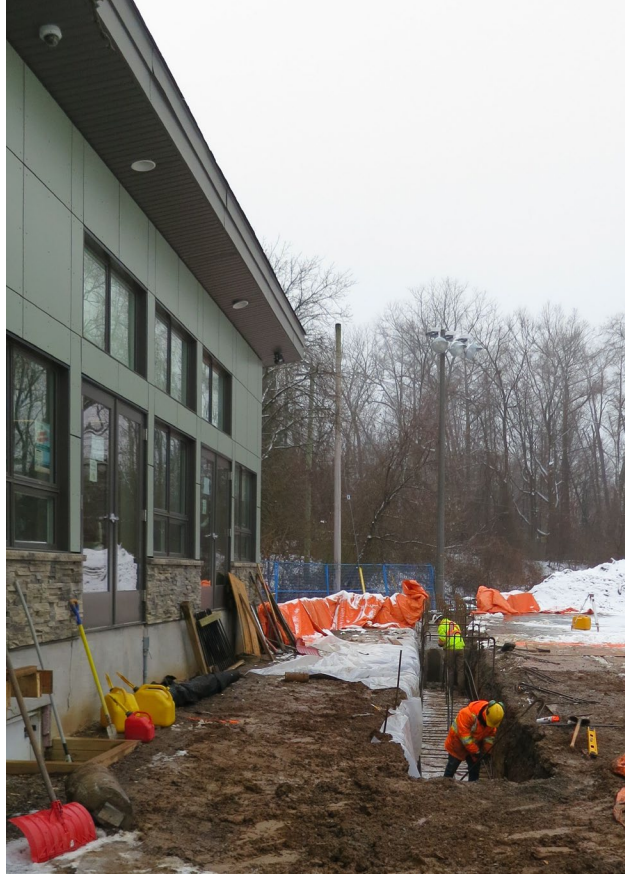
40 - Dec. 29th. Installation of the reinforcing steel for the foundation of the deck wall. Please note the polyethylene sheet. This sheet is to provide a "slip-plane" to prevent frost adhesion between the soil and the foundation wall concrete.
