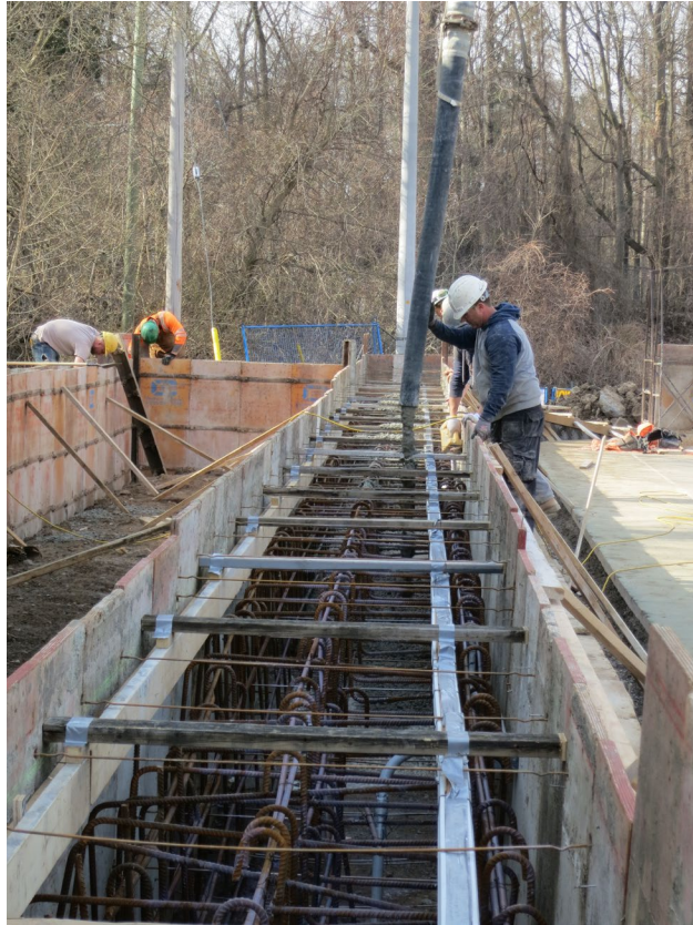
87 - April 13th. Construction of the deck wall.
