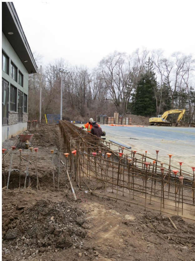
79 - April 1st. Deck wall ready for forming and the electricians are installing conduits for the electrical outlets in the wall facing the court. The Dome is attached to the top of the deck wall and also on top of the two transition walls on either side of the deck wall.
