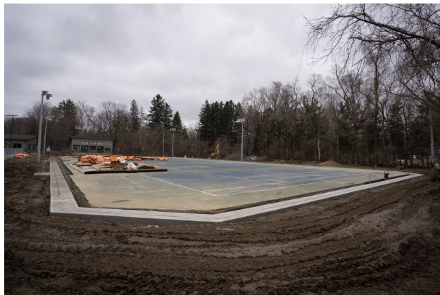
75 - March 28th, Overall view of the courts with the grade beam almost completed on three sides. The last section on the north side was poured this morning. Tomorrow, Tuesday March 29th, Demik will start the construction of the deck walls.
