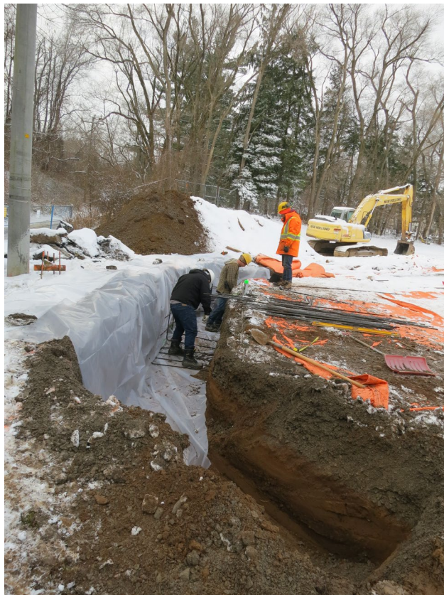
33 - December 20th. Construction of the grade beam at the South/East corner of the courts.
