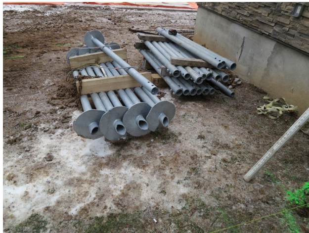
36 - Dec.22nd. A total of 11 helical piles (screw piles) were necessary on the south side of the club house. Based on the site specific ground conditions, each pile ended up approximately 21 ft. long.
