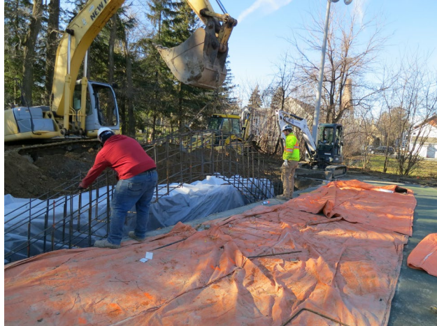
32 - December 17th. No, they are not building an "archway". The lowering of reinforcing steel into the trench and the concrete was poured this afternoon.
