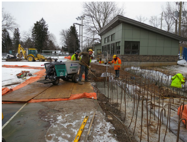
38 - Dec. 23rd. The pouring of concrete for the continuation of the foundation for the deck wall. The Dome fabric will be attached to the top of the wall . The deck will be a concrete one (fire regulation).
