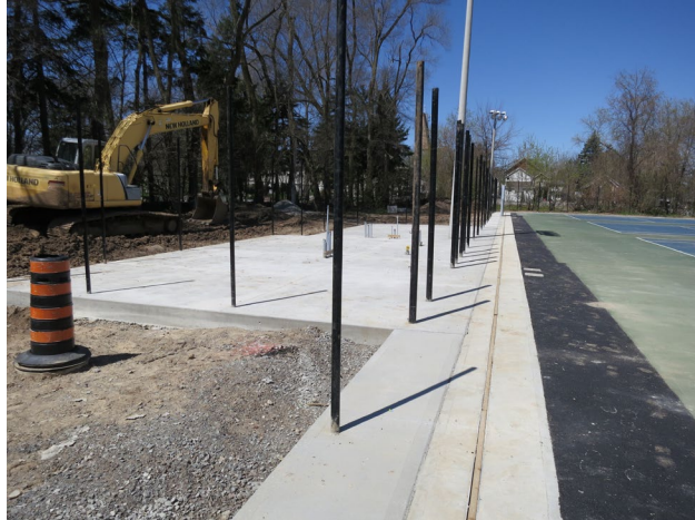
106 - 1st. week of May. Mechanical and storage shed pad. Court fence being installed.
