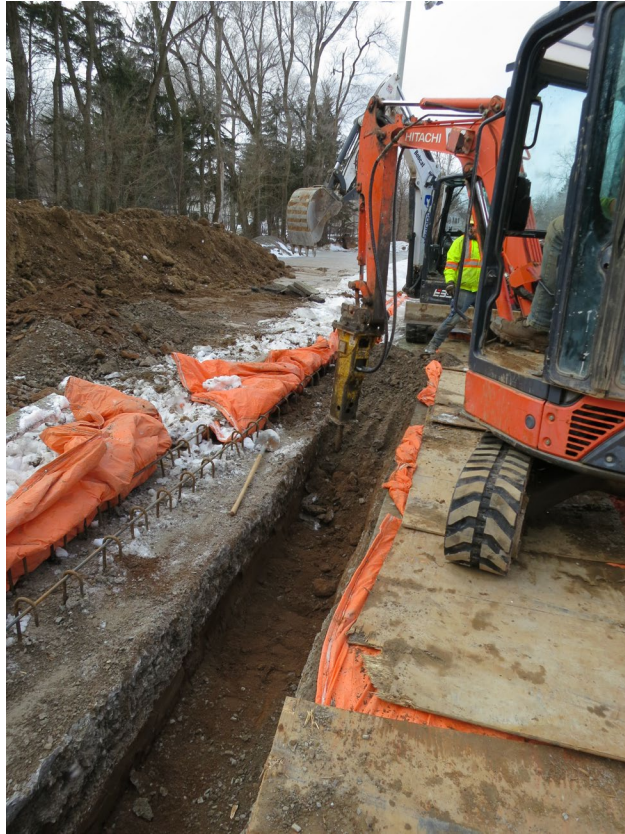
59 - Feb. 23rd. Since the frost is at least 4 feet down, Demik has to use a Hydraulic Breaker/ Jackhammer to loosen the soil. The trench is for the installation of the electrical conduits to be installed on the south side of the courts.
