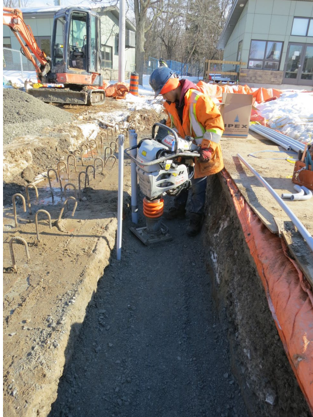
57 - Feb. 9th. Compaction of the granular fill.
