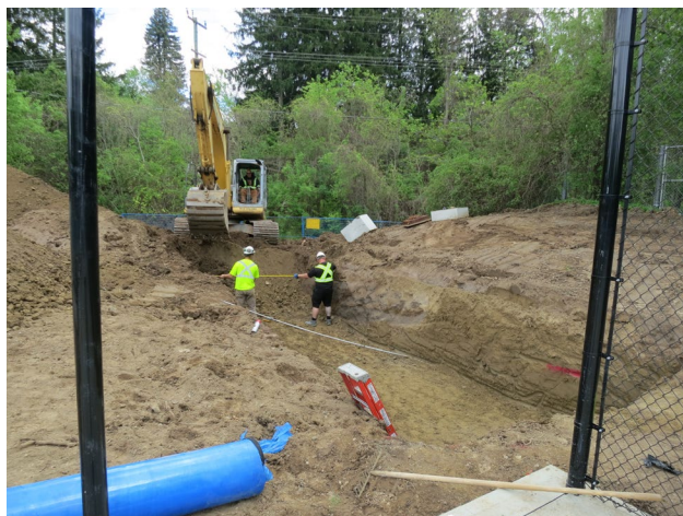
116 - May 17th. Construction of the storm water management infiltration system. This trench will be filled with 2 inch clear stone.
