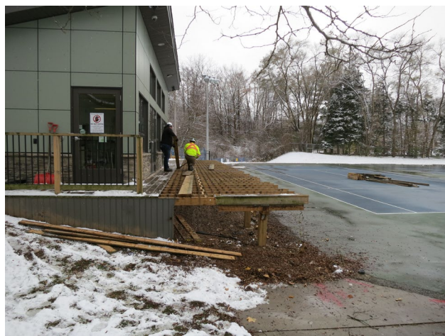
9 - Removal of wooden deck to be replaced by a concrete one ( fire regulation).
