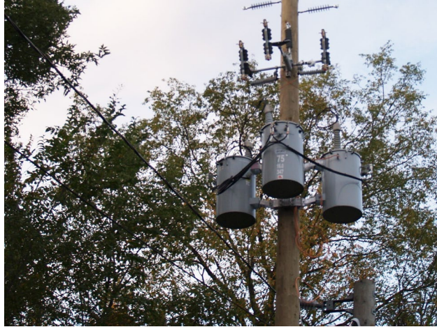
2 - November 30th. Installation of three phase transformer by Alectra utilities for the supply of extra power to the Dome's electrical equipment.
