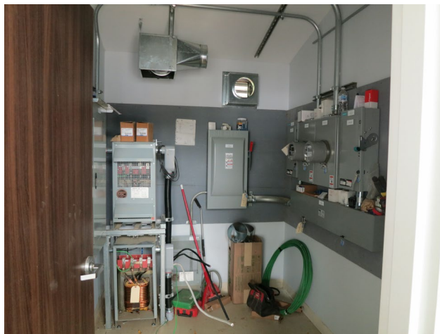
119 - May 19th. The electrical room is full of panels, switches and transformers to operate the Dome.
