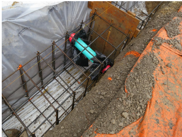
31 - Close up of 6" diam. PVC pipe.
