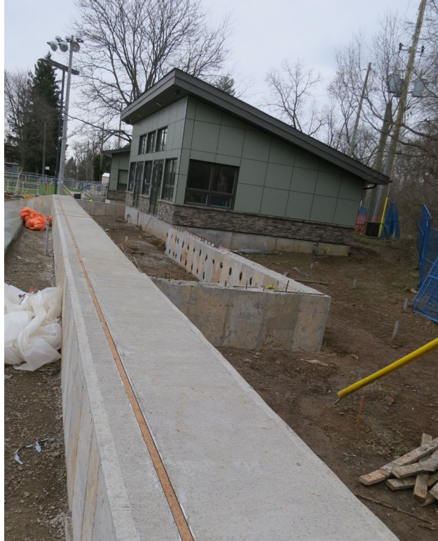
92 - April 14th. When the concrete is poured a 2x4 is inserted in the extrusion channel in which the dome is attached to. The back portion of the deck, beside the clubhouse, will be made out of wood. The posts will sit on the visible tubes (helical piles).
