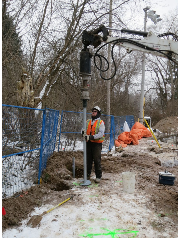
35 - Dec. 22nd. Helical Pile installation. Helical piles are a manufactured steel foundation anchor. The purpose of a helical pile is to provide foundational support for structures. In our case, required for the construction of the concrete deck and the wood deck, immediately south of the clubhouse..
