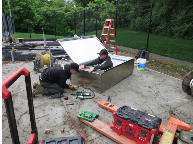
126 - June 9th. Electricians drilling holes for the installation of the electrical cabinet. I trust the fellow in the cabinet is wearing his safety boots.
