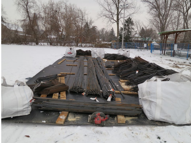
21 - Delivery of reinforcing steel.
