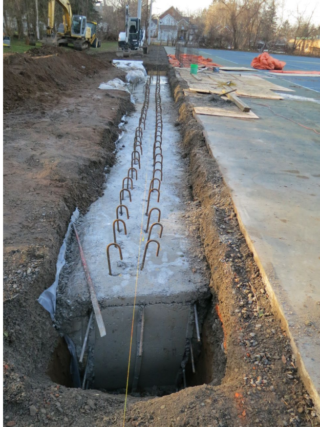
29 - Phase I of the grade beam completed. Phase II will be the concrete cap on top of Phase I, and this cap will house the aluminum rail holding the Dome fabric in place.
