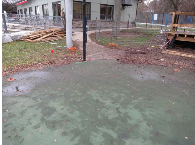
10 - Orange markers indicating building envelope. Location where the Dome fabric meets the grade beam.
