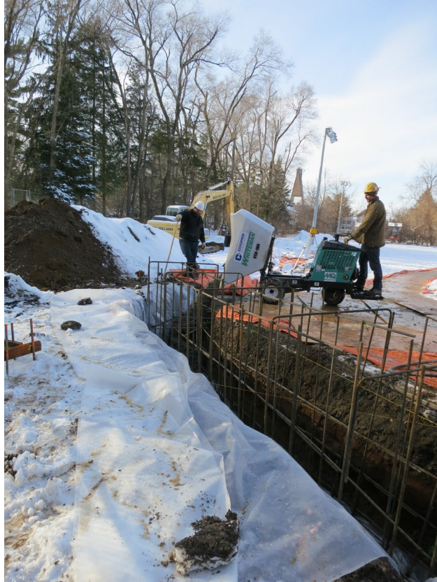
34 - December 20th. Pouring of the concrete at the South/East corner of the courts. The height of this section will gradually change from deck level to ground level.
