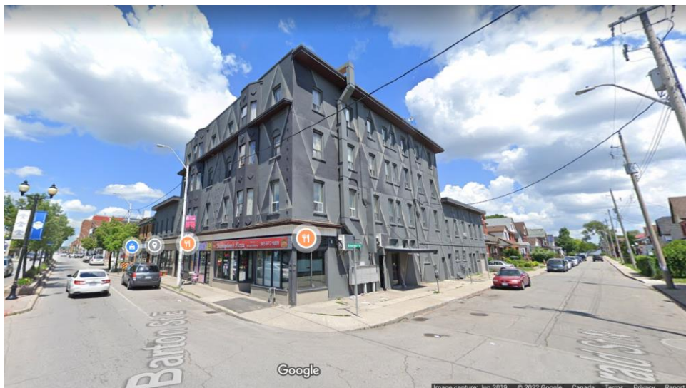
Figure 4 – Mixed Use Building at Northwest Corner of Barton/Emerald
