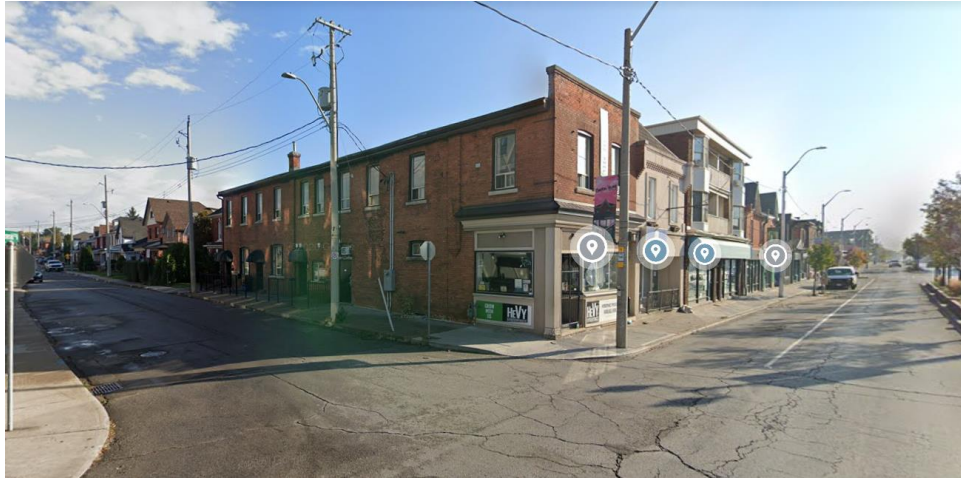
Figure 8 – Mixed Use Building to East of Subject Property
