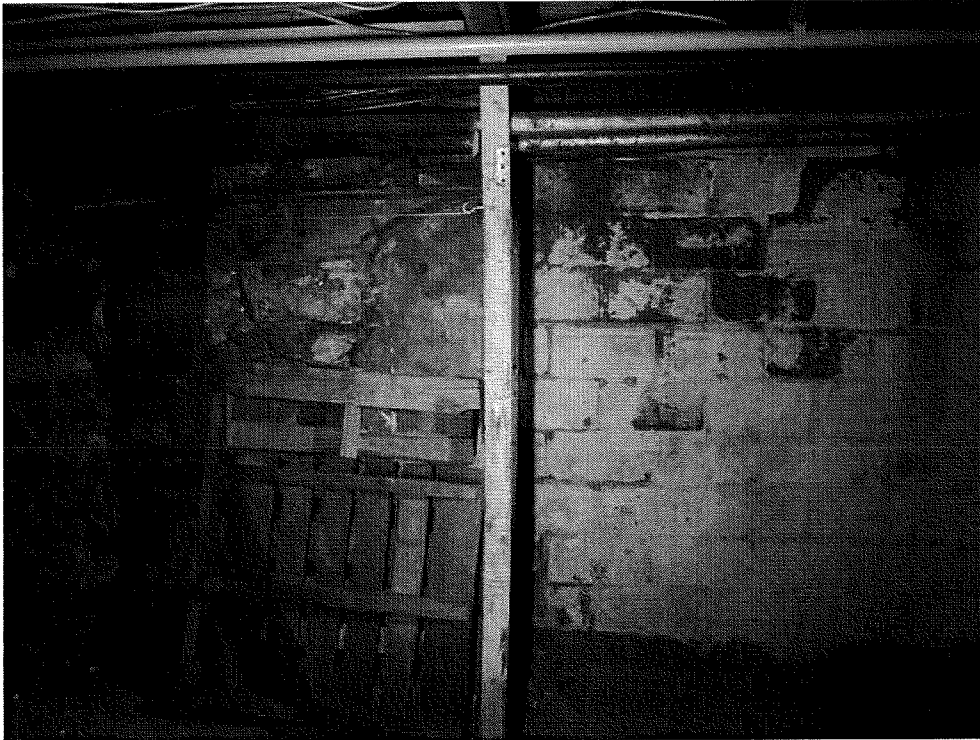
BASEMENT – rubblestone under the historic portion at the front and concrete block under the later additions at the back
