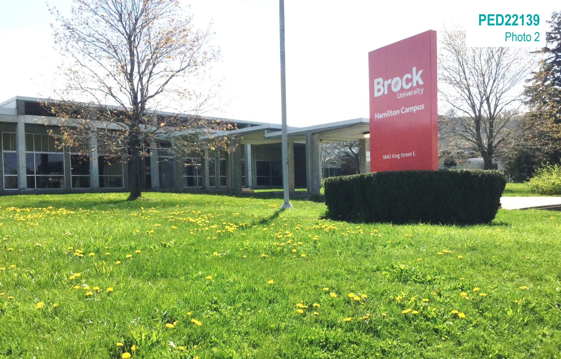
Subject property 1842 King Street East (central portion of the property), as seen from King Street East looking south west
