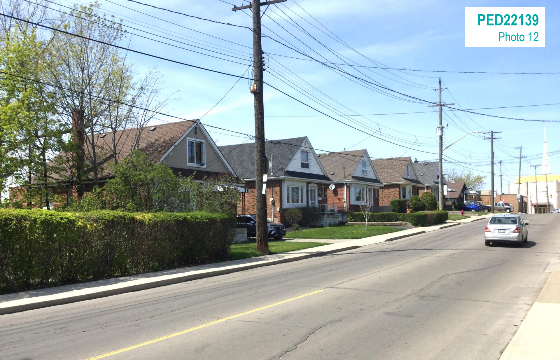
24, 28, 30, 32, 36 and 40 Rosedale Avenue, located to the east of the subject lands, as seen from Rosedale Avenue looking north west
