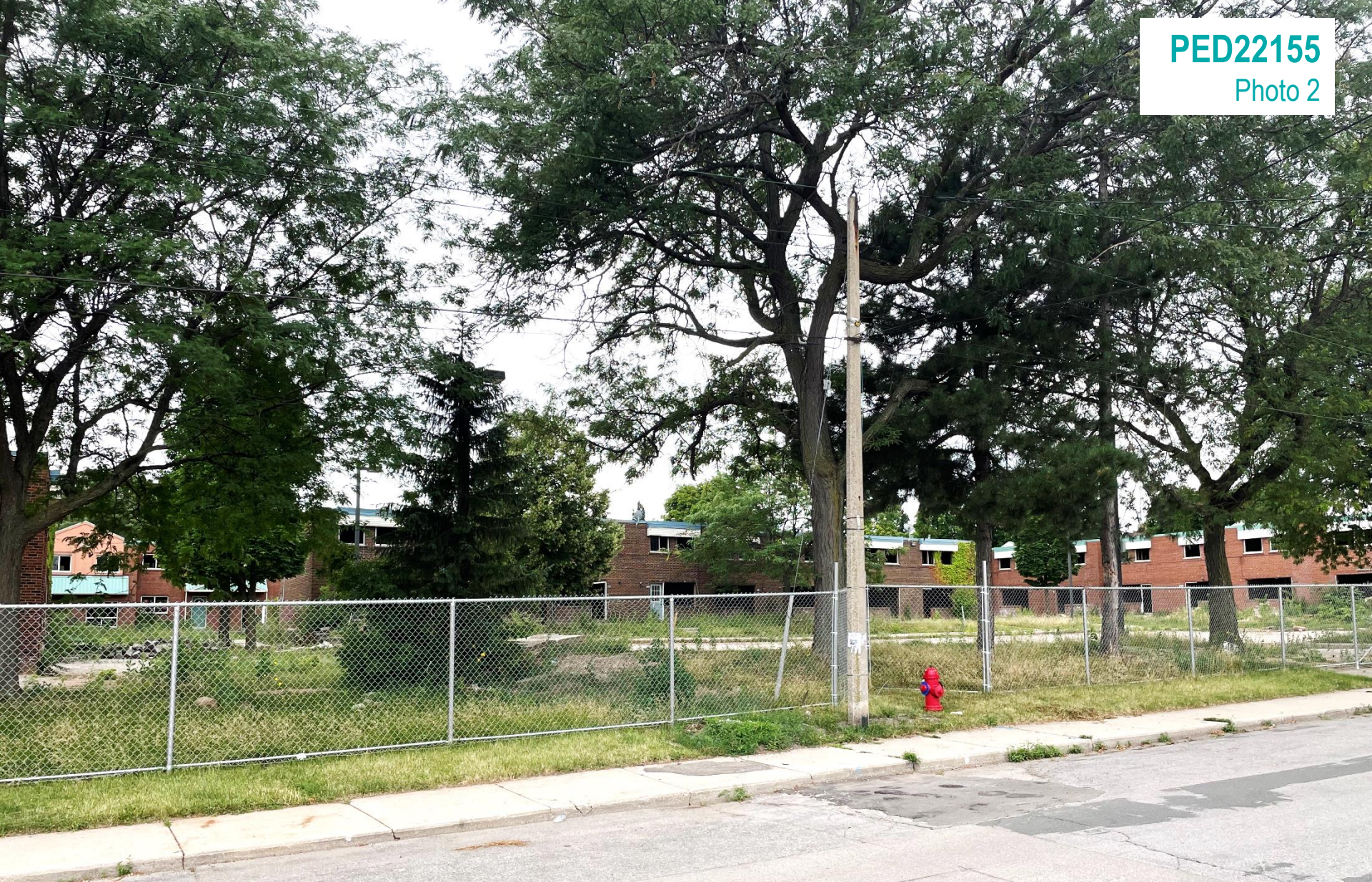
Subject site from Ferrie Street West
