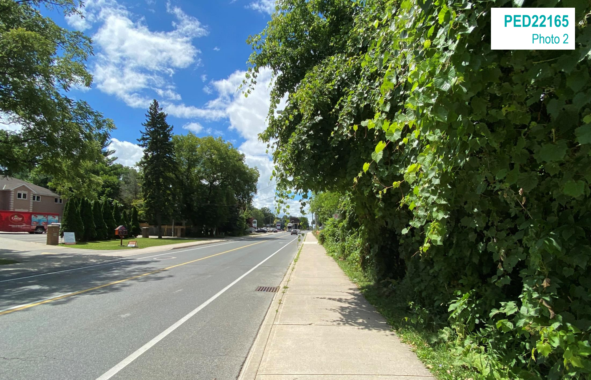
View looking south (Brantford Bound)
