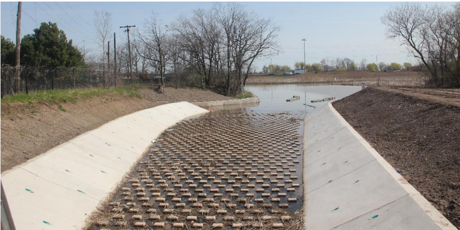
Figure 8: New Outfall & Dissipation Zone Construction
