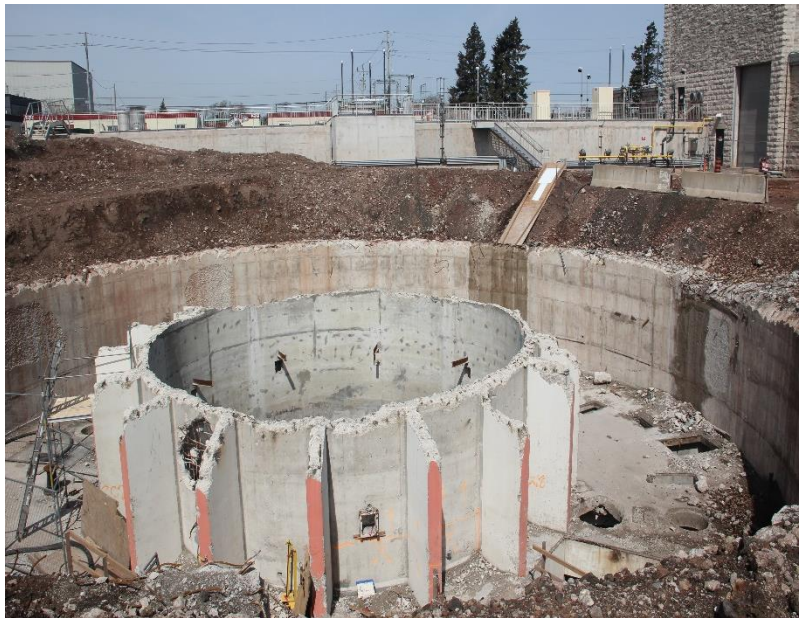
Figure 2: Demolition of old Main Pumping Station - Subgrade
