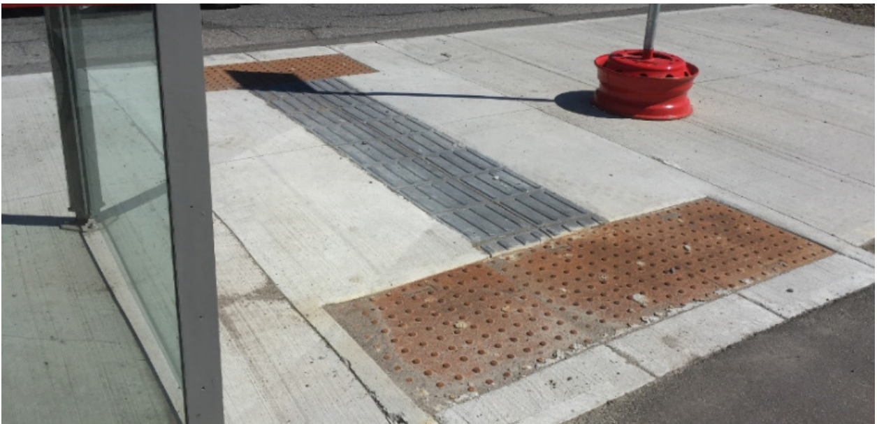
A guidance TWSI in grey used to guide pedestrians between a bus stop (left) and a cycle track crossing (right). Red attention TWSI's are used to identify hazards at each end. Ottawa, ON
