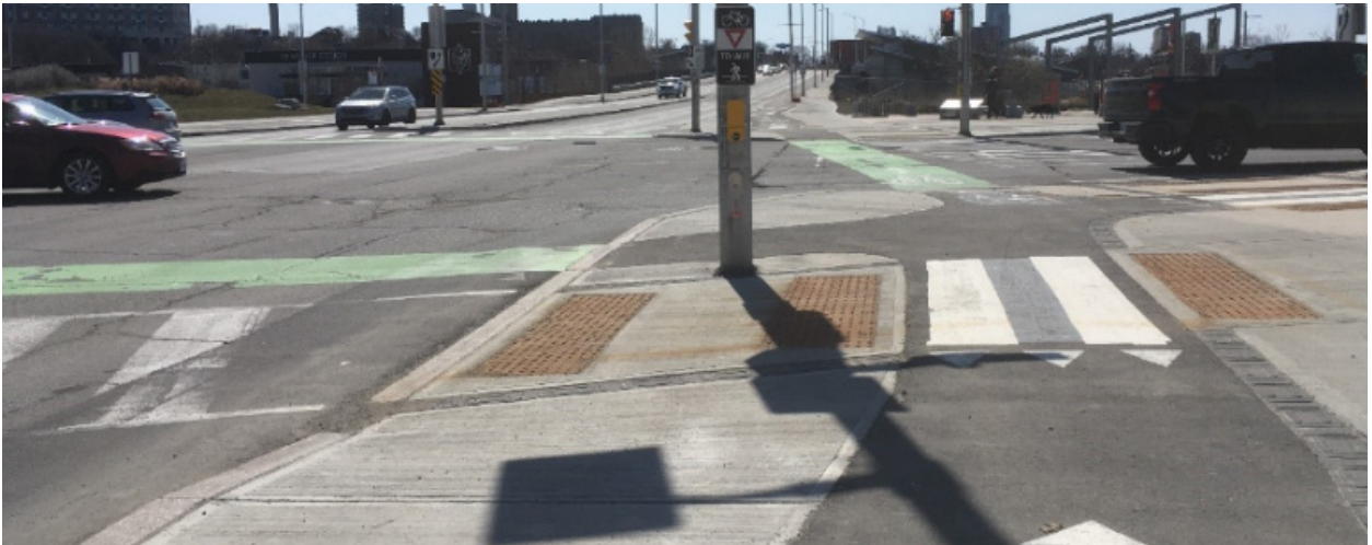
An example of a pedestrian refuge between a cycle track and roadway crossing, denoted by attention TWSI's at each end. Ottawa, ON
