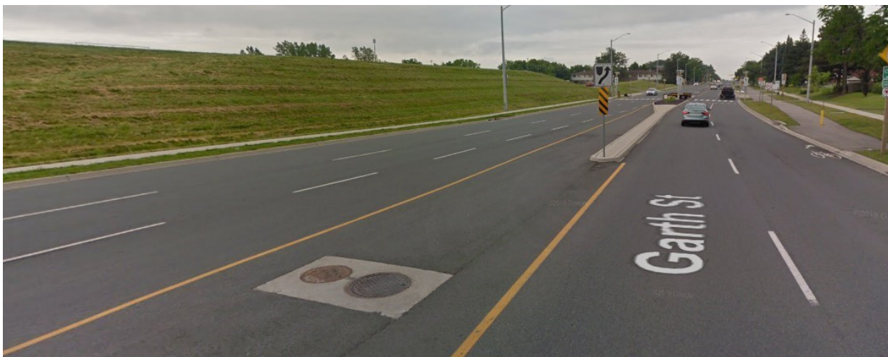
Maintenance holes positioned outside the wheel path of motor vehicles and bicycles on Garth St. in Hamilton. Source: Google Maps
