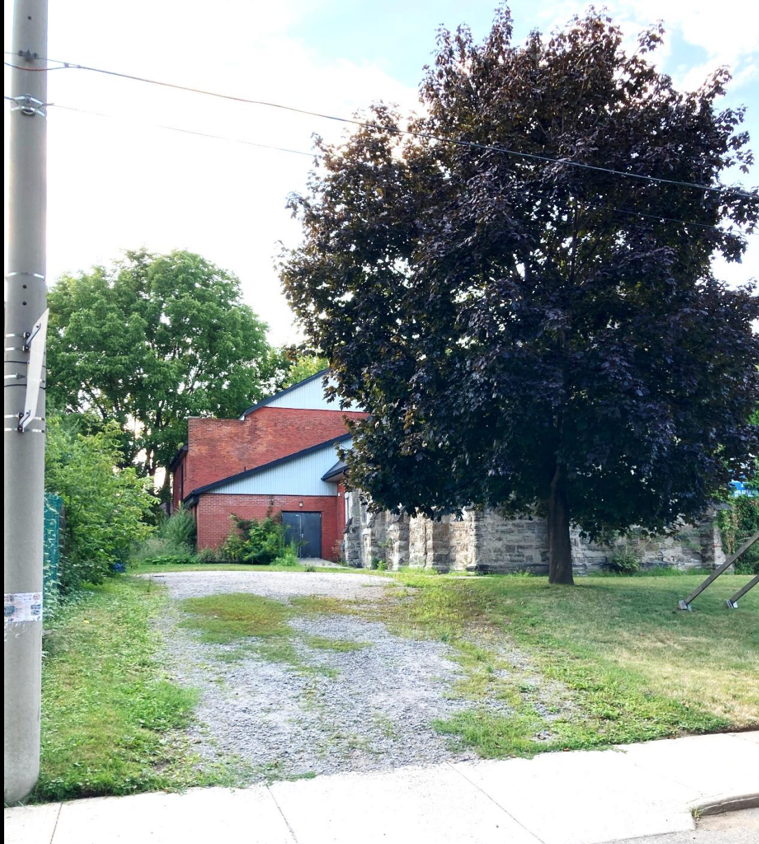
Driveway to be maintained and rear of subject
