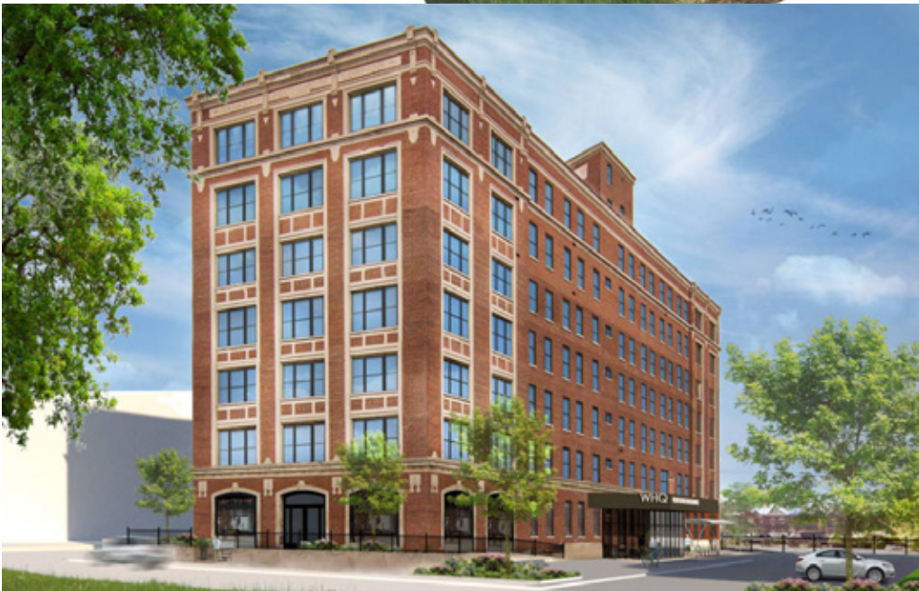
Example of industrial building adaptive reuse in the Westinghouse HQ Building. Credit: mcCallumSather
