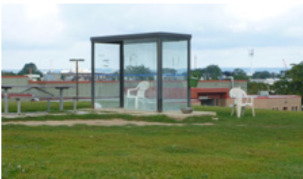
View of existing condition at Birch Street Dog Park, one of the few park spaces in the Bayfront. Credit: Dillon Consulting
