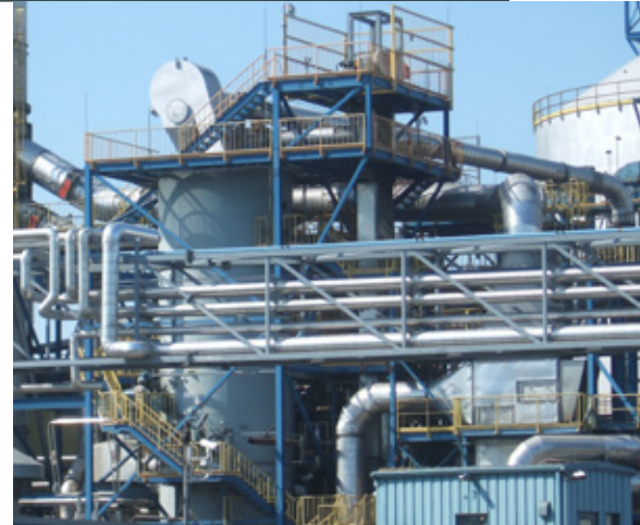
"Dazzling Ducts" by Stephen Ronald Fast - a photo submission to the "Beauty in the Bayfront" photo contest.
