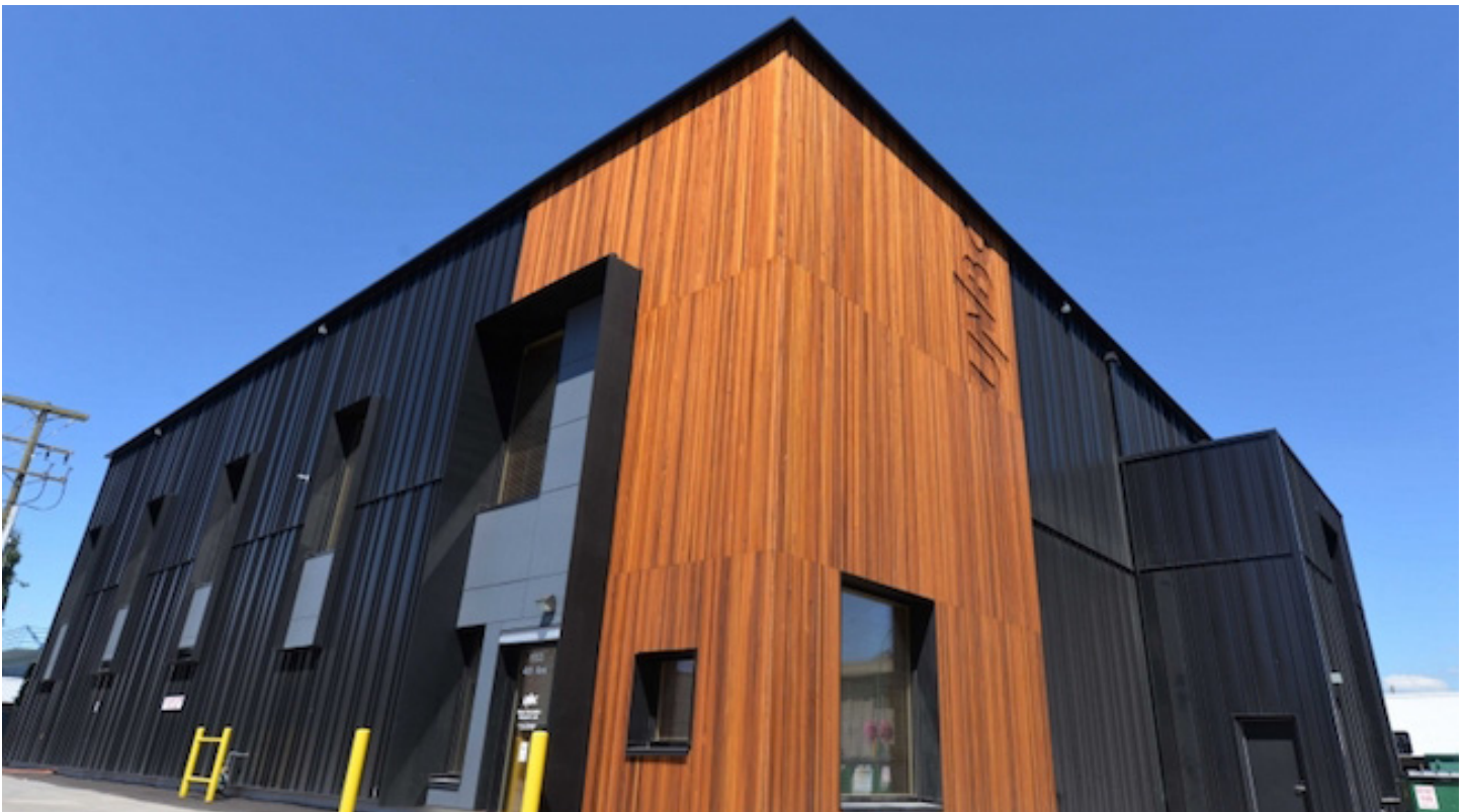
Reducing energy consumption through building design and siting, Industrial Wood Innovation Research Lab at University of Northern British Columbia is Passive House certified, Prince George B.C., Credit: UNBC
