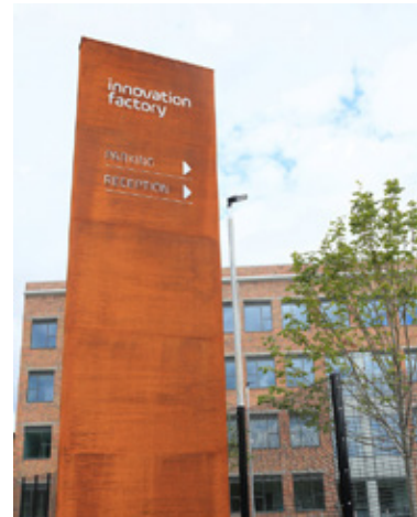
Streetscape entrance signage. Forthriver Innovation Centre, Belfast, Ireland. Credit: Ascot House
