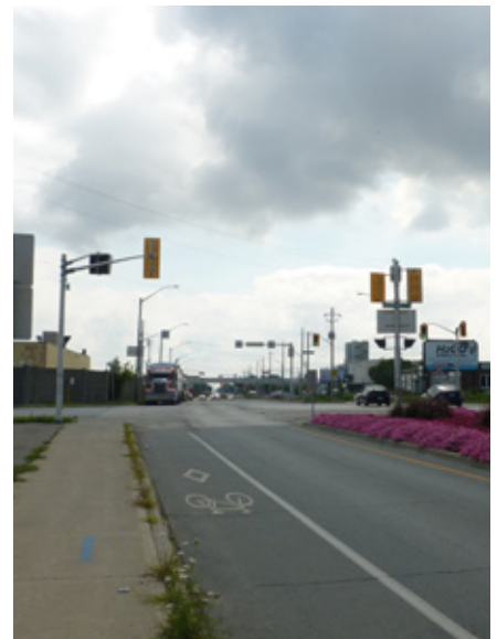
View of existing condition at west Gateway, Burlington Street East at Wellington Street North. Credit: Dillon Consulting
