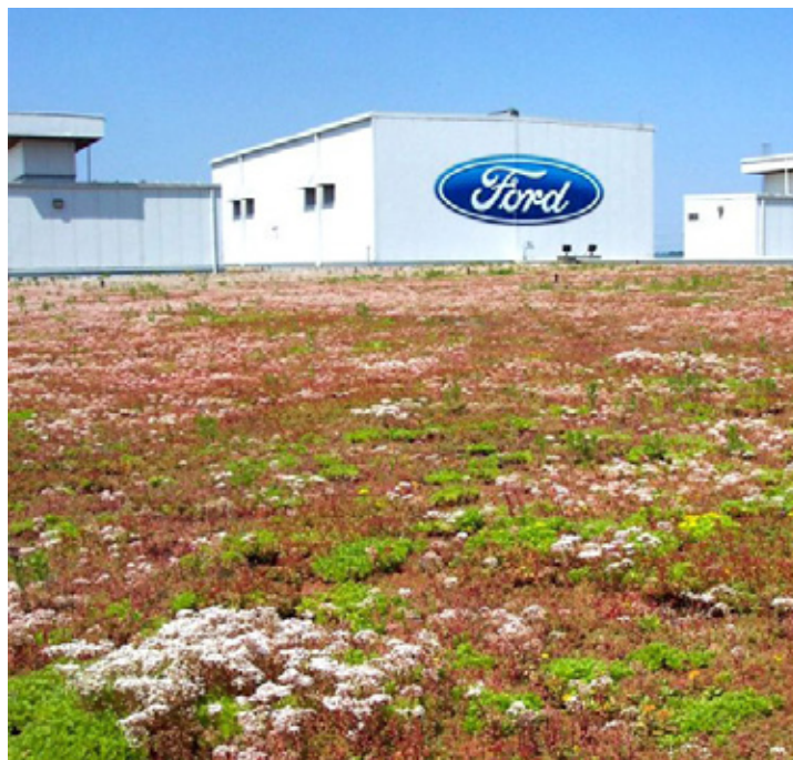
Example of reduction of hardscape to improve site filtration, Ford Motor Company Factory Green Roof, River Rouge, MI Credit: Xero Flor America, LLC
