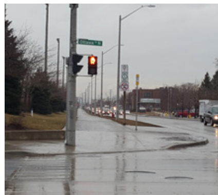
View of incomplete multi-use Trail along Burlington Street East at Ottawa Street North. Credit: Dillon Consulting
