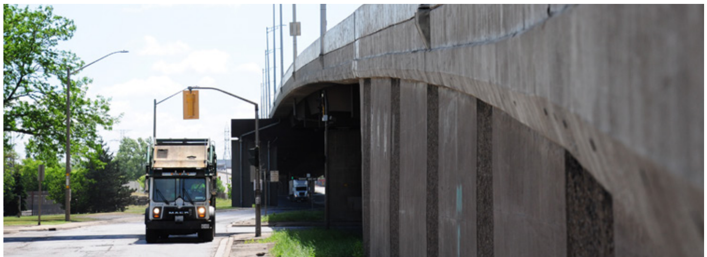
View depicting the many levels of industry functioning in the Bayfront. At-grade roads, elevated roads, and overhead infrastructure intertwine the horizon. Credit: Dillon Consulting
