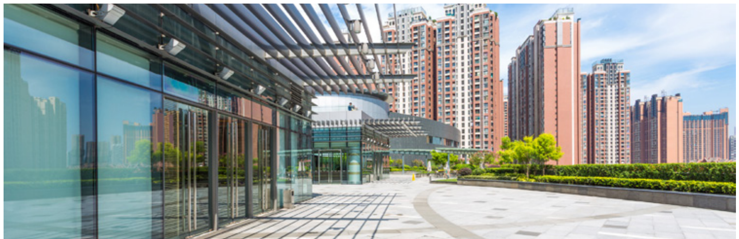
Building with shade structure. Credit: Zhu Difeng
