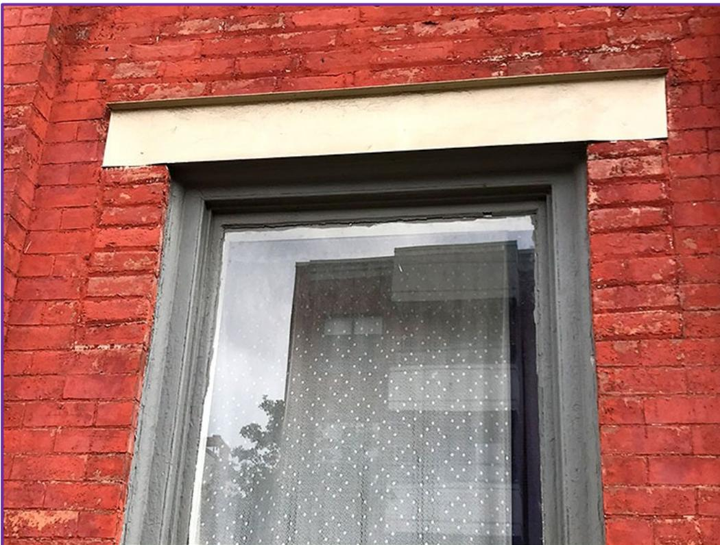
Close-up view of the stacked bricks framing the top of the windows and the aluminum now protecting the brick masonry lintels, once obscured and protected by the galvanized-iron window hoods. AG September 2022
