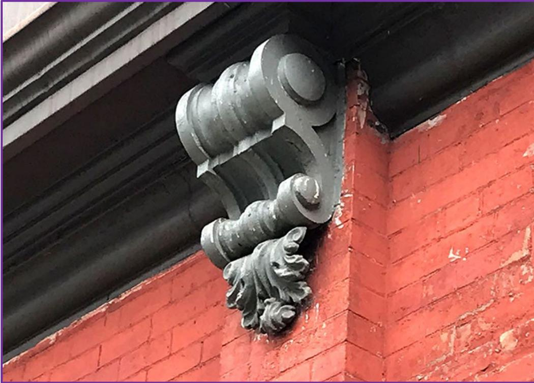
Close-up view of one of the galvanized iron brackets mounted to the brick piers below the cornice defining to the top of the first storey. AG September 2022
