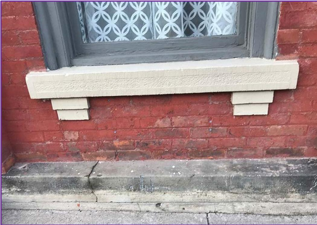
Closeup view of one of the six identical stone sills and the projecting cut stone blocks of the above grade foundation wall. AG August 2022
