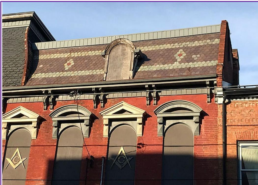
Close-up view of the upper façade showing the galvanized-iron window hoods, paired wood eave brackets, polychromatic roofing slates and one of two badly deteriorated roof dormers. AG August 2022
