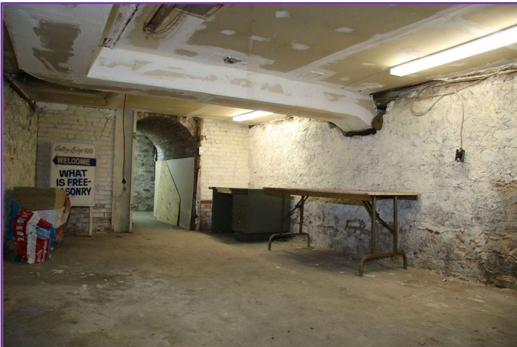
Basement area with rubblestone walls looking towards a barrel-vaulted archway (orientation unknown).
