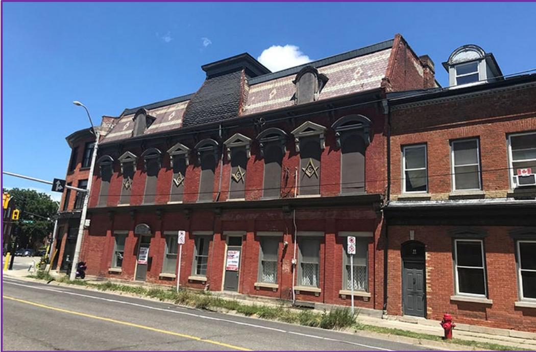
Second storey windows have either been removed and replaced by wood sheets or covered up. The brick masonry was at some point painted but this paint layer has been peeling off for some time. AG August 2022
