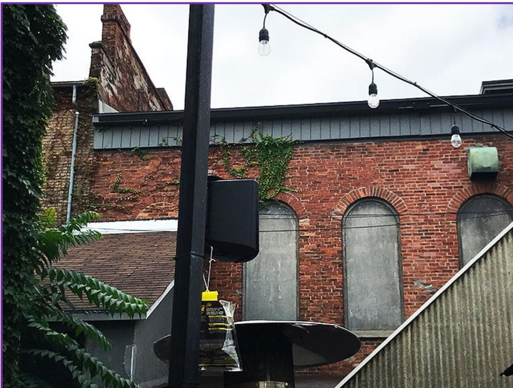
A section of the rear façade viewed from King Street, showing four round-arched window openings, one bricked in and largely obscured by a shed-roofed addition and three filled in with wood panels.
