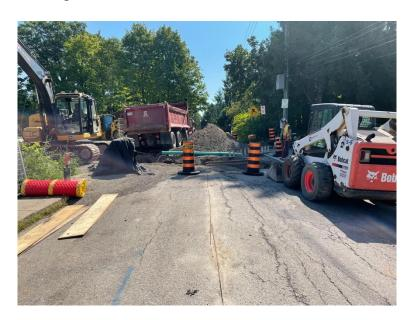
The road is closed as is the single sidewalk. A storm sewer is being installed to accommodate excess runoff from infiltration basins on the 15 Church site.
