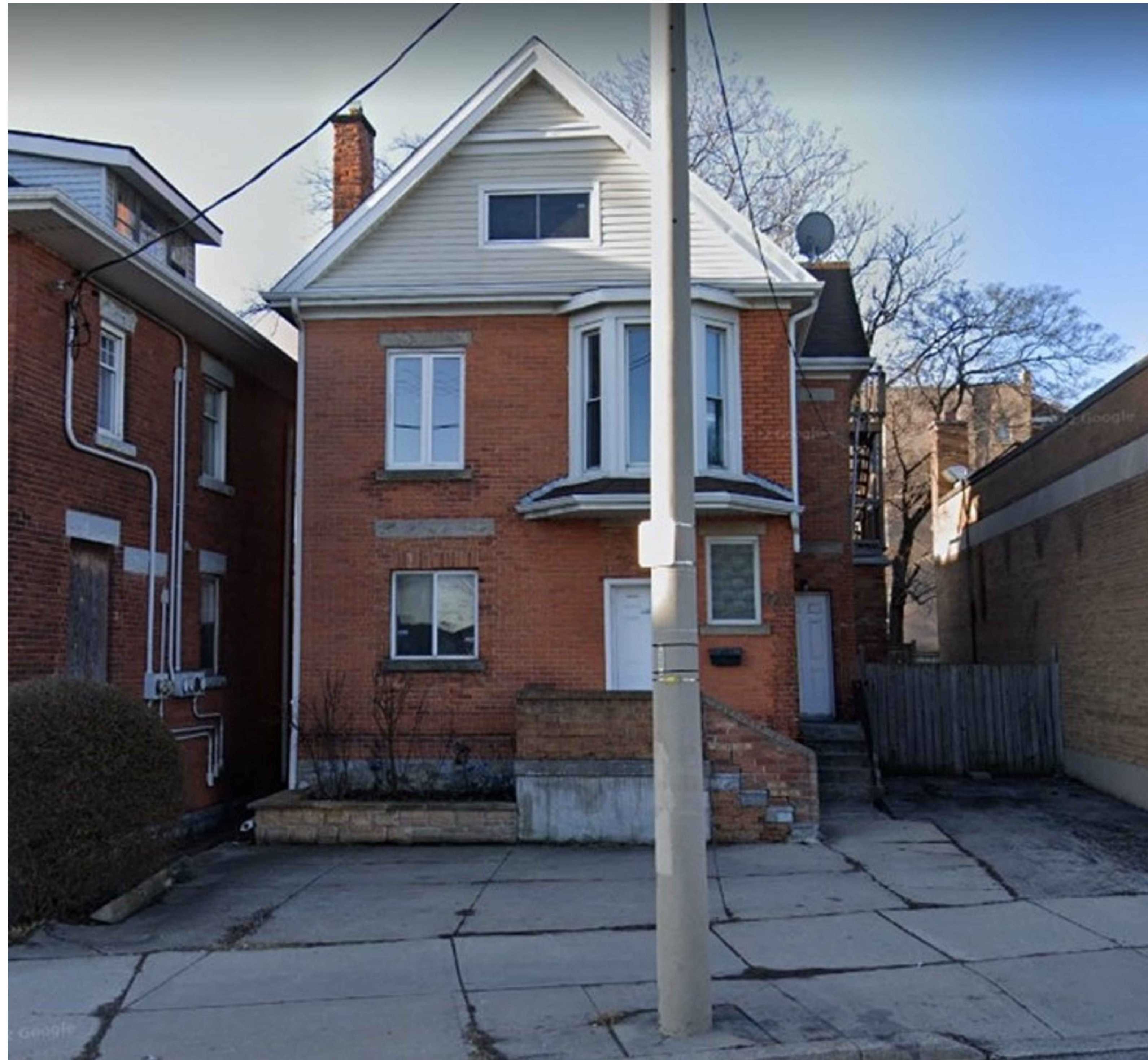
EXISTING BUILDING IMAGE
