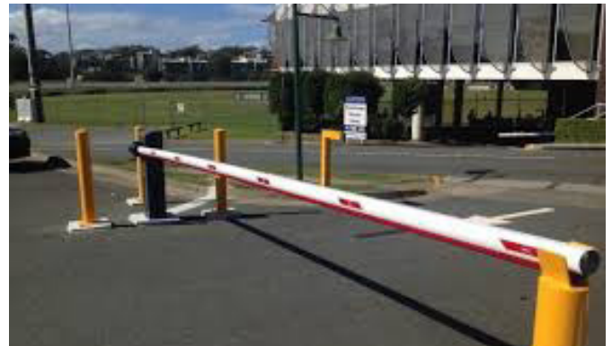
Figure 21: Crash gates and crash bars did not meet criteria for pedestrian movement, heritage or aesthetic considerations
