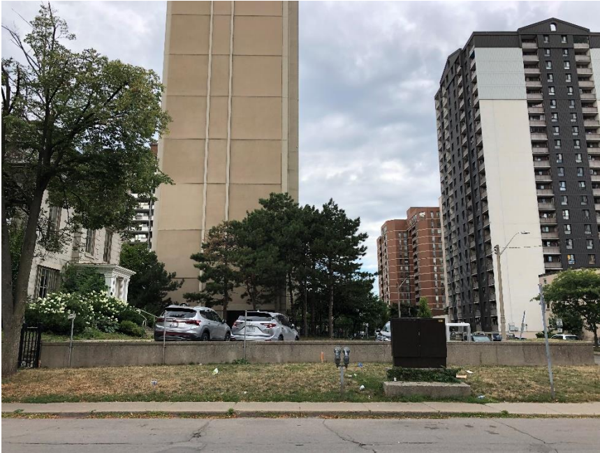
Plate 5: Nineteenth-century former residence on subject property visible at far left with apartment tower in the background (A.S.I. 2022)
