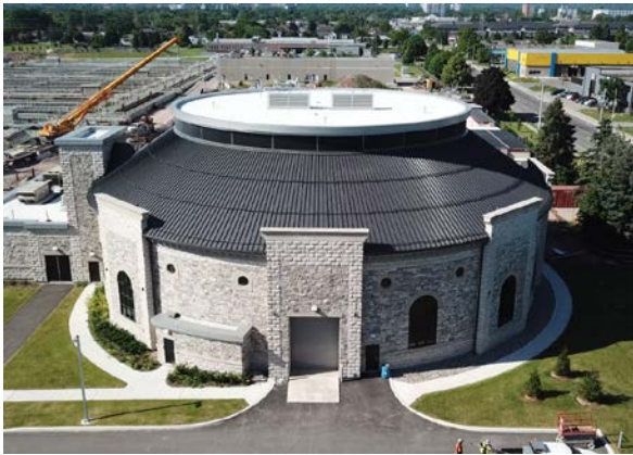
CONTRACT 1 Main Pumping Station
