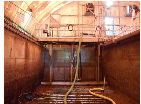
Dundas WWTP repairs
