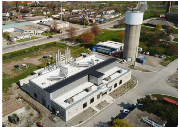
CONTRACT 2 Electrical Power Centre
