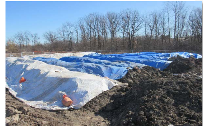
Excess soils, Woodward WWTP
