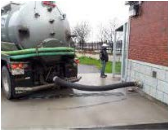
Septage hauling station
