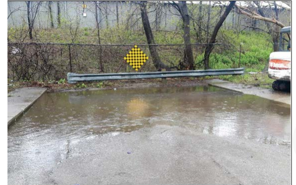
Beach Boulevard Flood Remediation
