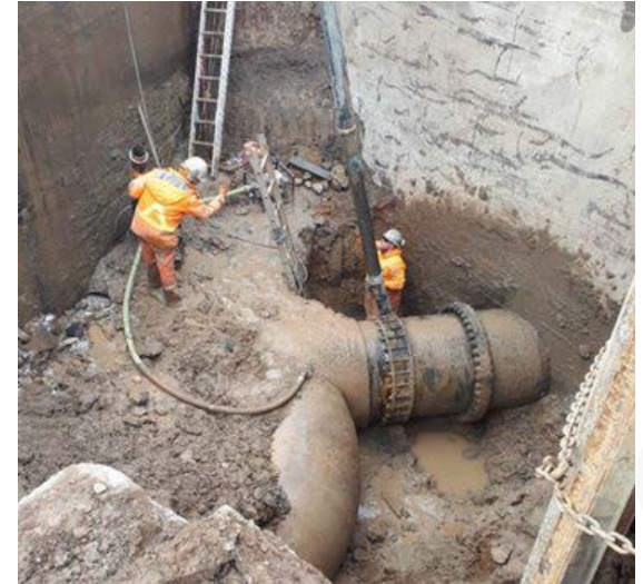
Woodward WTP upgrades
