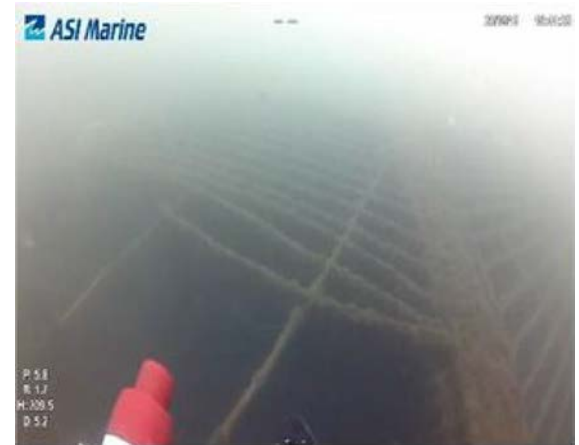
Low lift raw water intake
