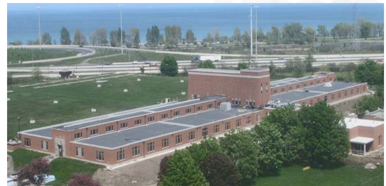
Woodward WTP Pre-treatment and Filter Building
