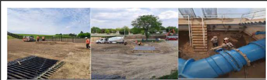
Stone Church & Garth Reservoir Valve chamber and valve house upgrades - $5.8M
