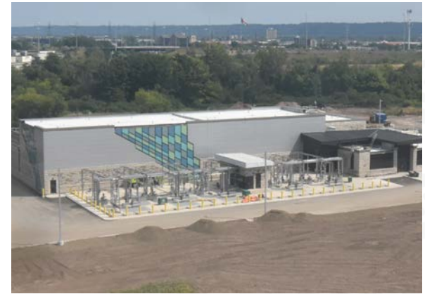
CONTRACT 3 Tertiary Treatment Upgrades
