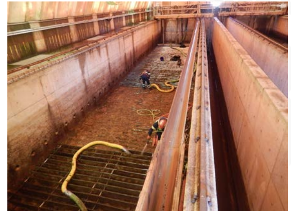
Dundas WWTP upgrades
