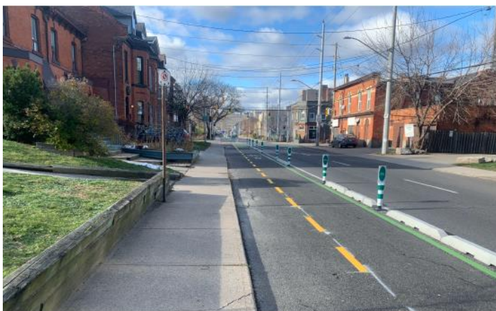
Hunter St, Hamilton Flexposts and precast curbs
