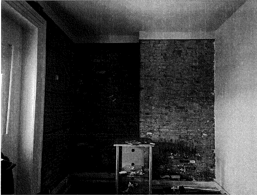
115-117 George Street, Interior Brick Wall City of Hamilton, January 20, 2023
