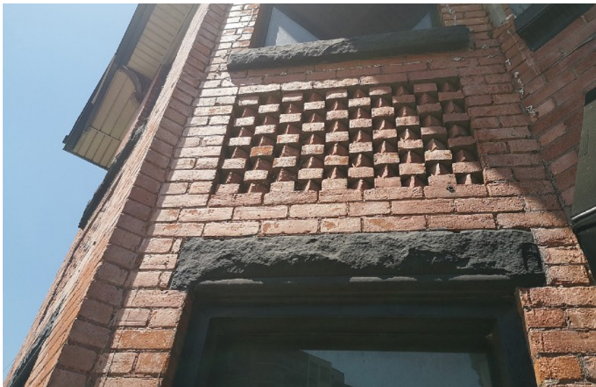
Close-up at exterior wall, showing the checkered brick pattern at the spandrel. The walls appear to have a remnant thin film over the brick surfaces. Note the modern cladding at the soffit above.
