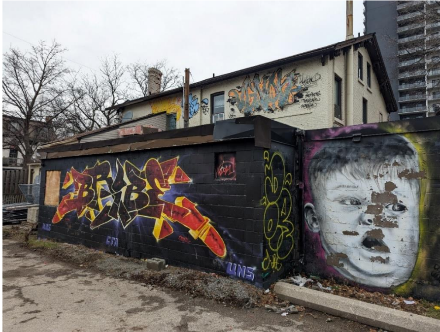
115-117 George Street, East and South (Side and Rear) Elevations City of Hamilton, January 20, 2023
