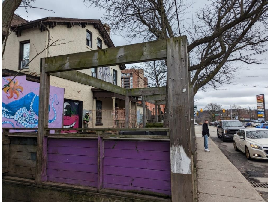
115-117 George Street, North and West (Front and Side) Elevations City of Hamilton, January 20, 2023
