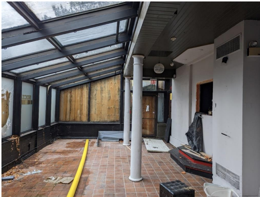
115-117 George Street, Front Sunroom Addition Facing East City of Hamilton, January 20, 2023
