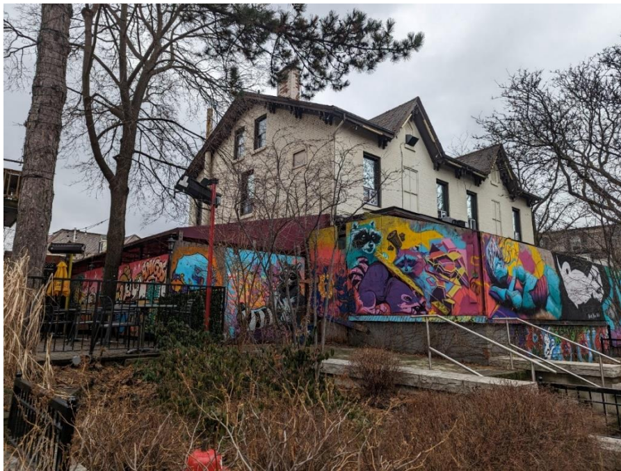
115-117 George Street, North and East (Front and Side) Elevations City of Hamilton, January 20, 2023
