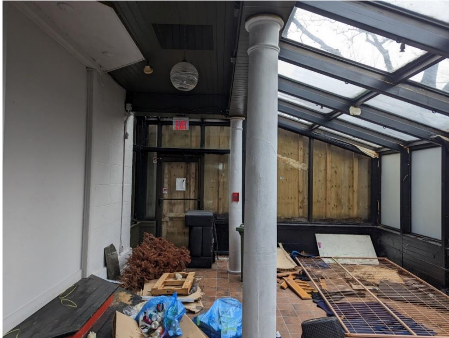
115-117 George Street, Front Sunroom Addition Facing West City of Hamilton, January 20, 2023
