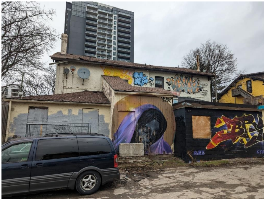
115-117 George Street, South (Rear) Elevation City of Hamilton, January 20, 2023
