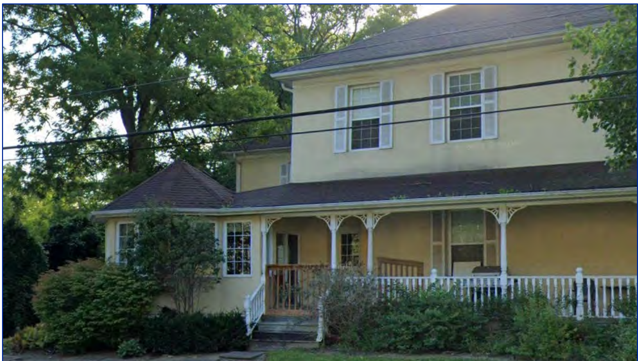
Figure 26: View of the sliding glass door entrance into the sunroom
