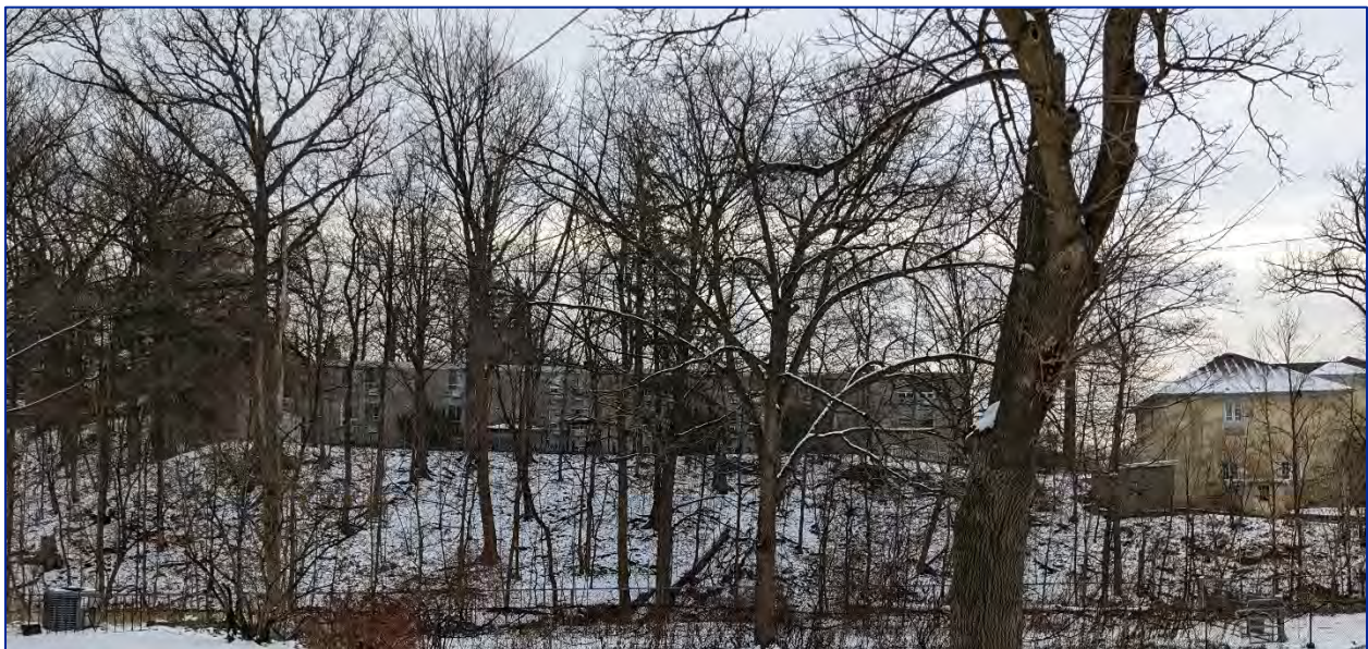
Figure 32: View of the north elevation of the continuing care centre
