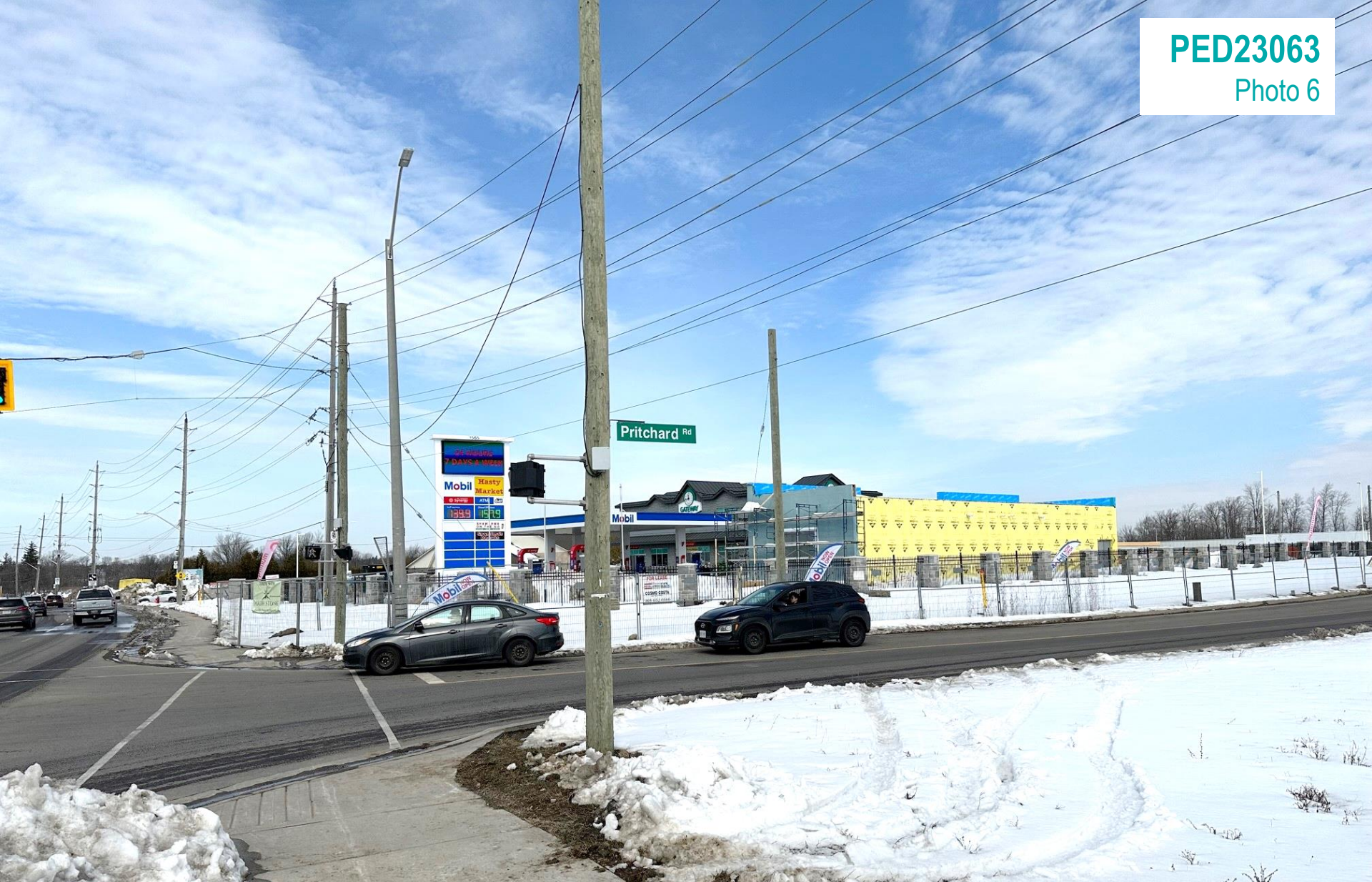
1557 and 1565 Rymal Road East and 694 Pritchard Road, Hamilton - Facing Northwest
