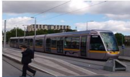
Overhead Catenary System (OCS)
