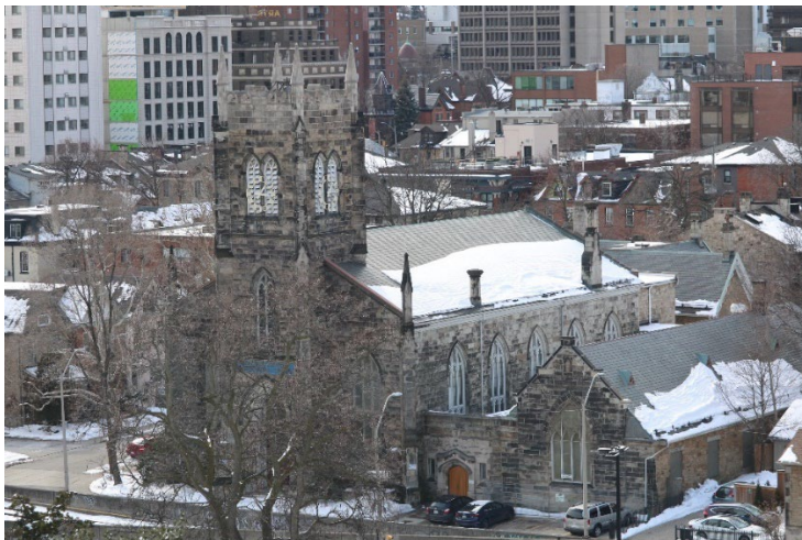
114-116 MacNab Avenue South, Hamilton (Source: CDSB Staff)
