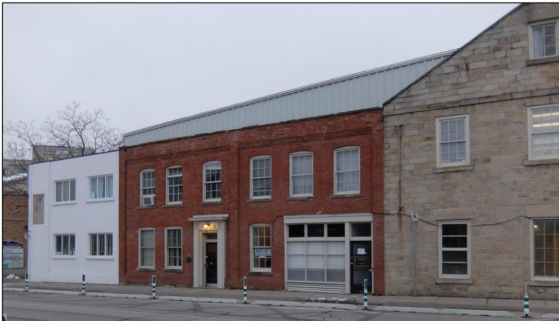
Image 4: Northern elevation (from left to right), Building Nos. 11, 7, & 1 (December 2022)
