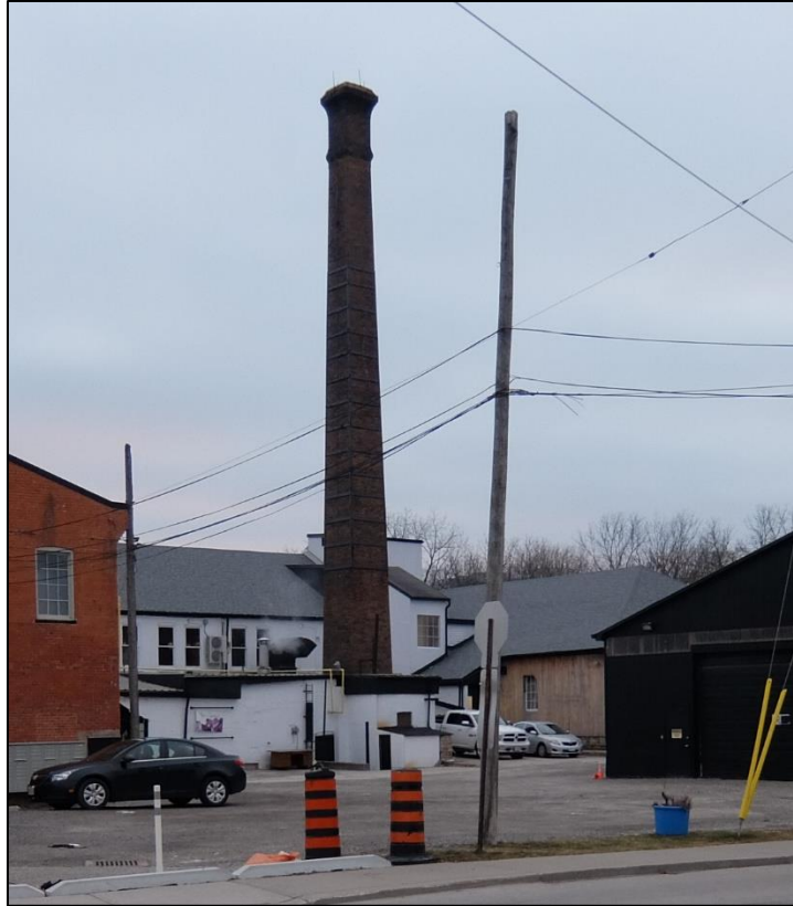
Image 13: Closeup of chimney (January 2023)
