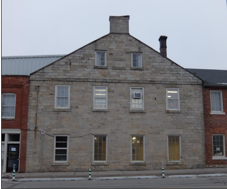
Image 3: Northern elevation, Building No. 1 (December 2022)
