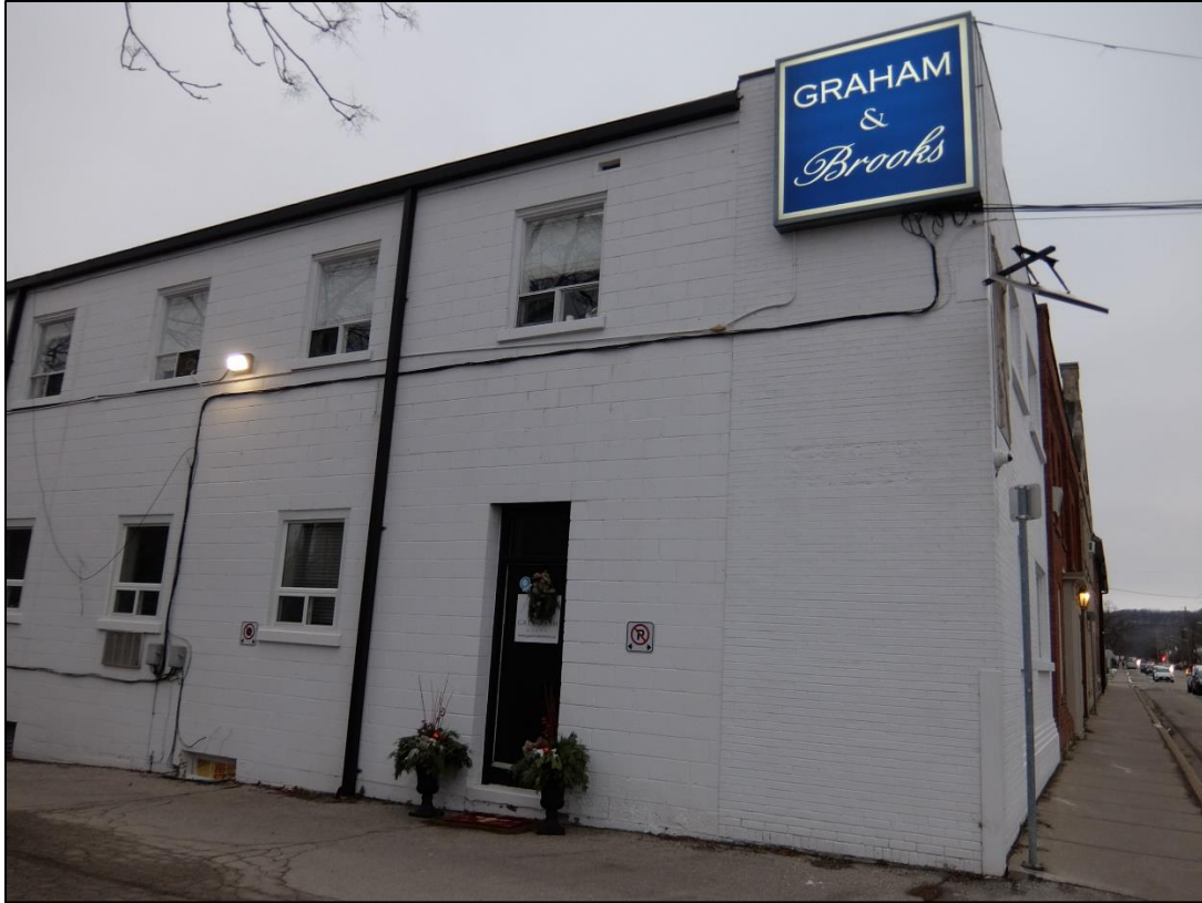
Image 9: Eastern elevation, east wall of Building No. 11 (December 2022)
