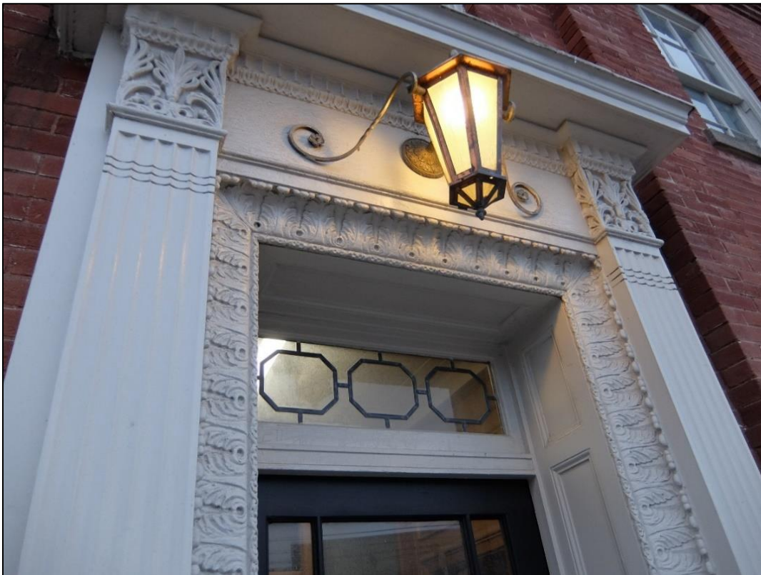
Figure 16: Details on door of Building No. 7 (December 2022)
