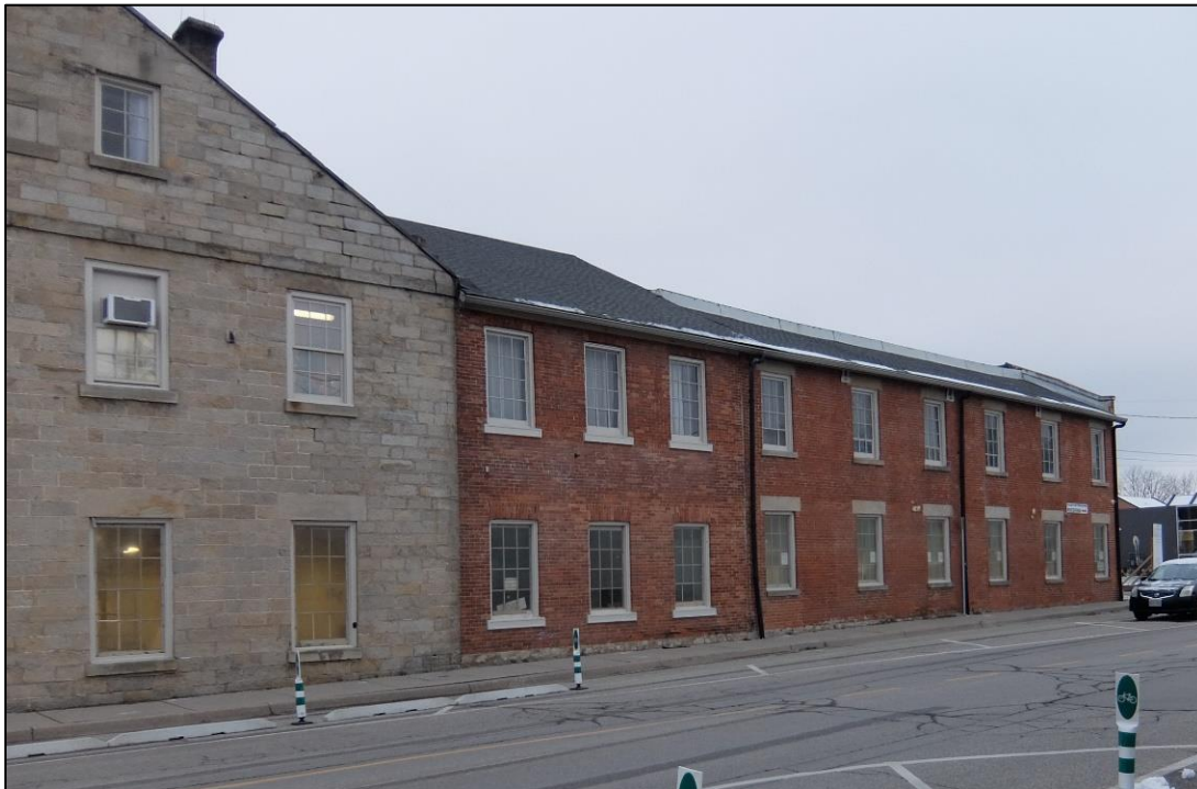
Image 10: Northern elevation (from left to right), Building Nos. 1, 4, and 2 (December 2022)
