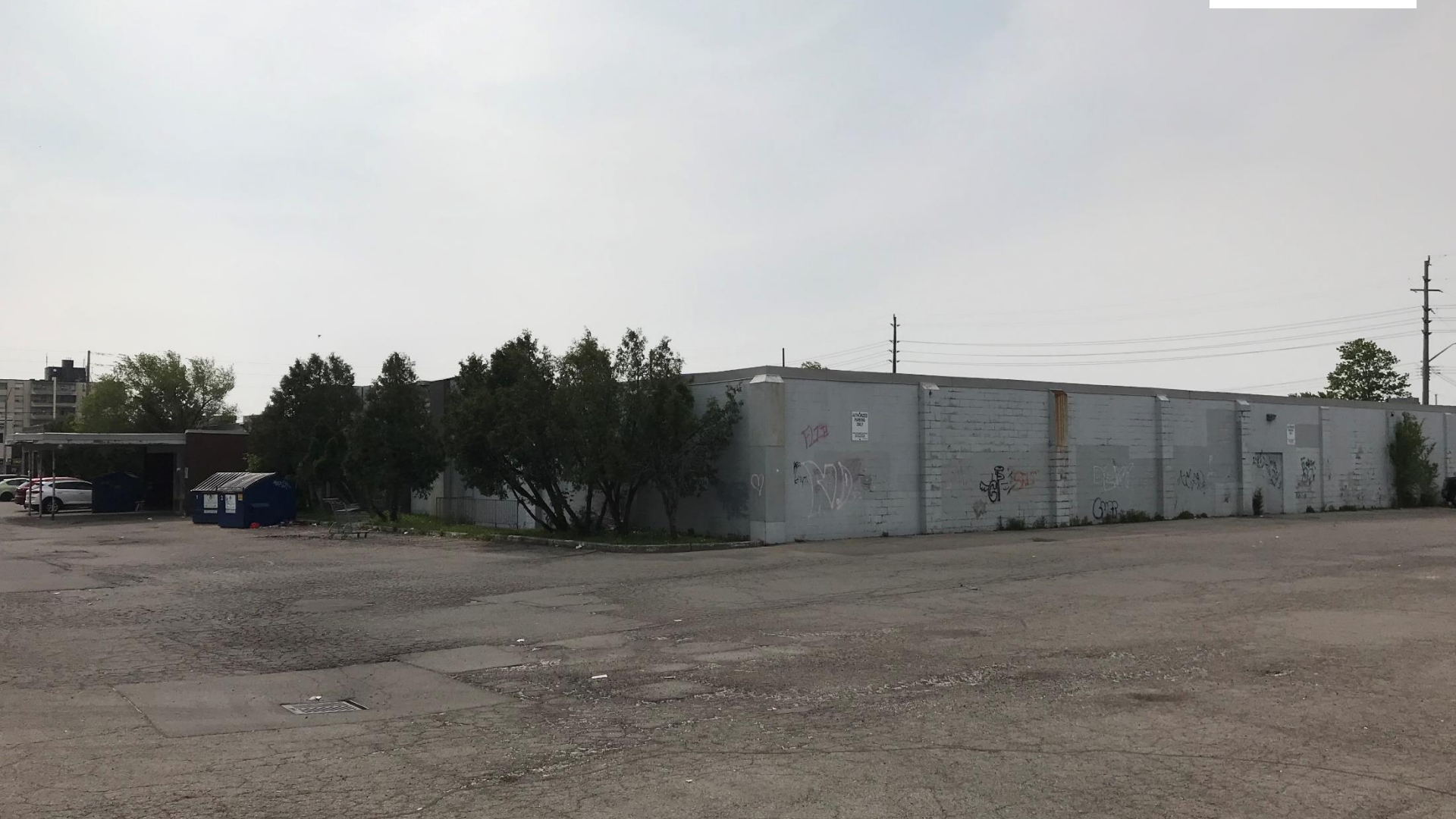
Subject Lands – View from northeast corner
