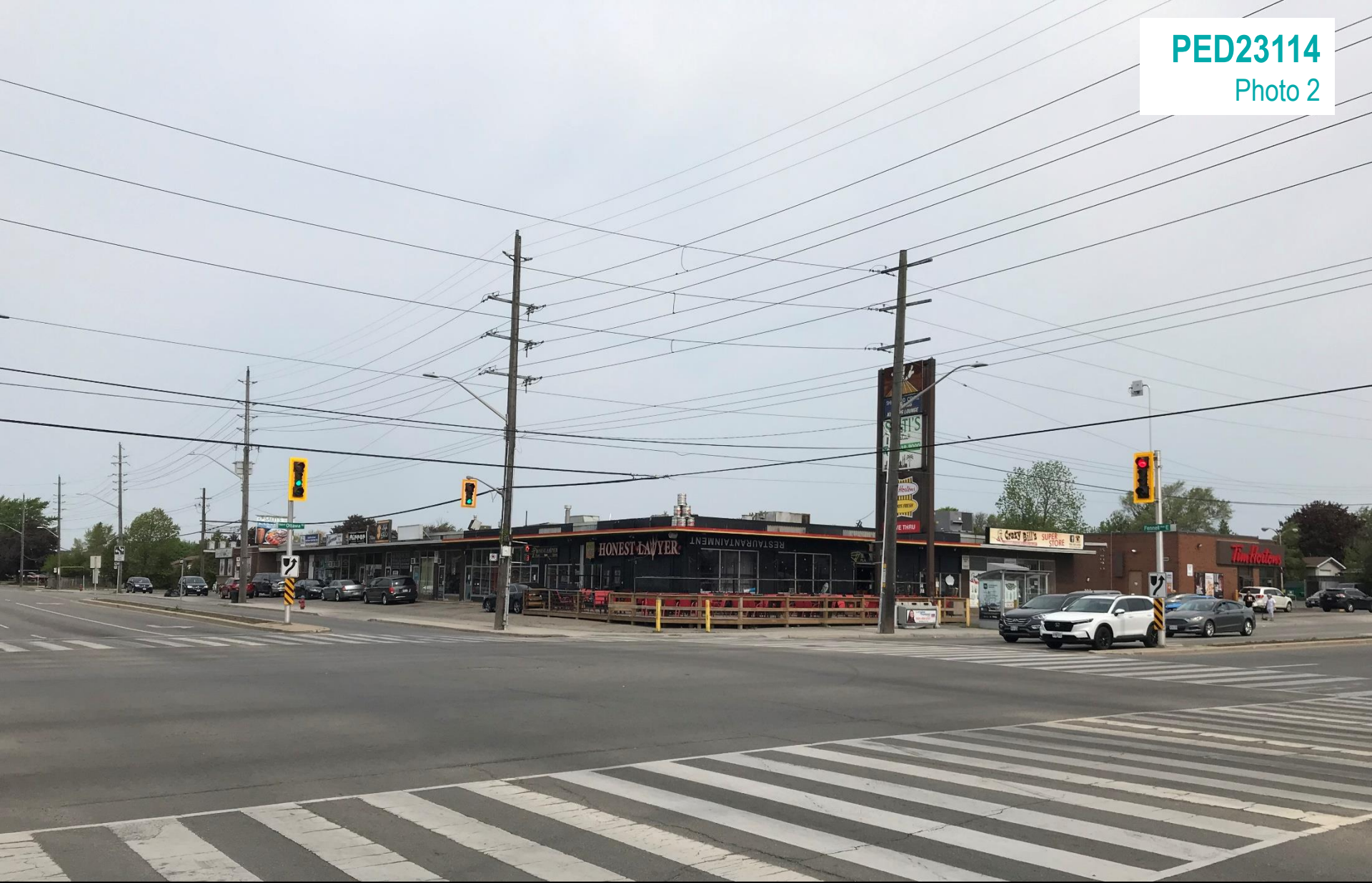
Subject Lands – View from southeast corner
