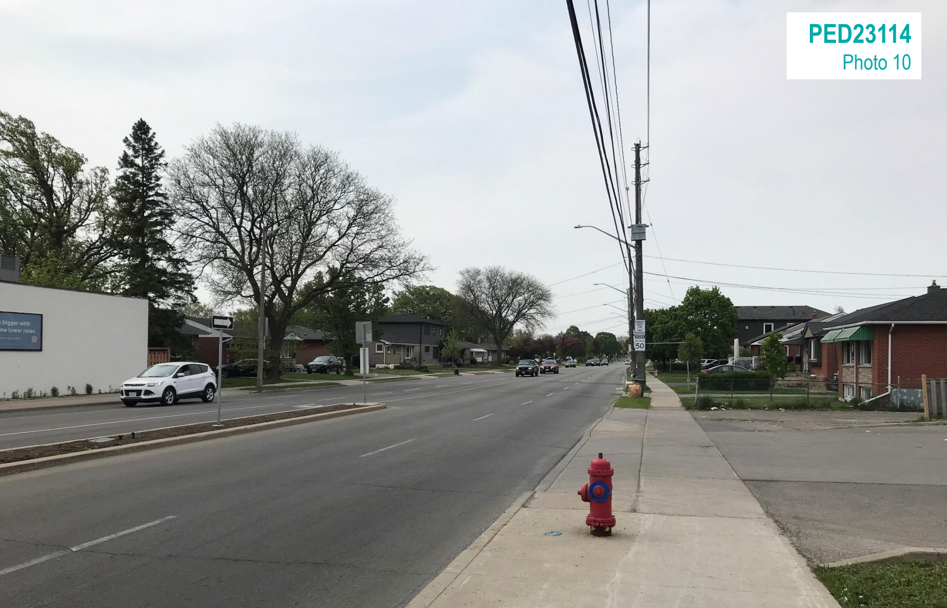
Upper Ottawa Street – Looking south
