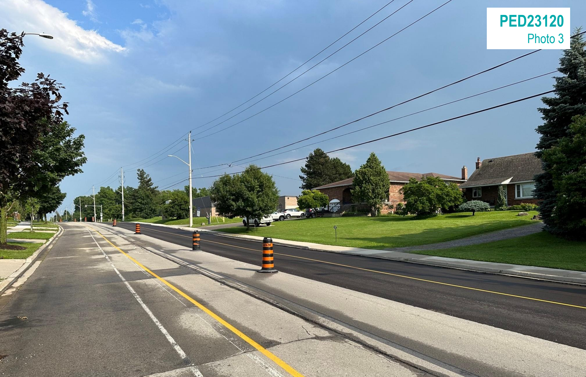
View looking southeast from Highland Road West
