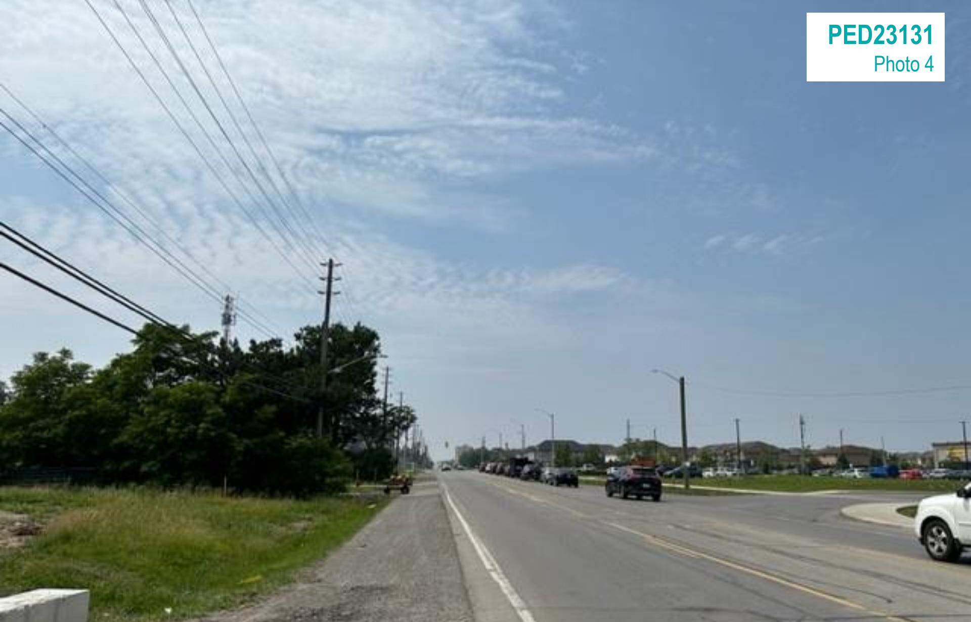
705 and 713 Rymal Road East - Facing west
