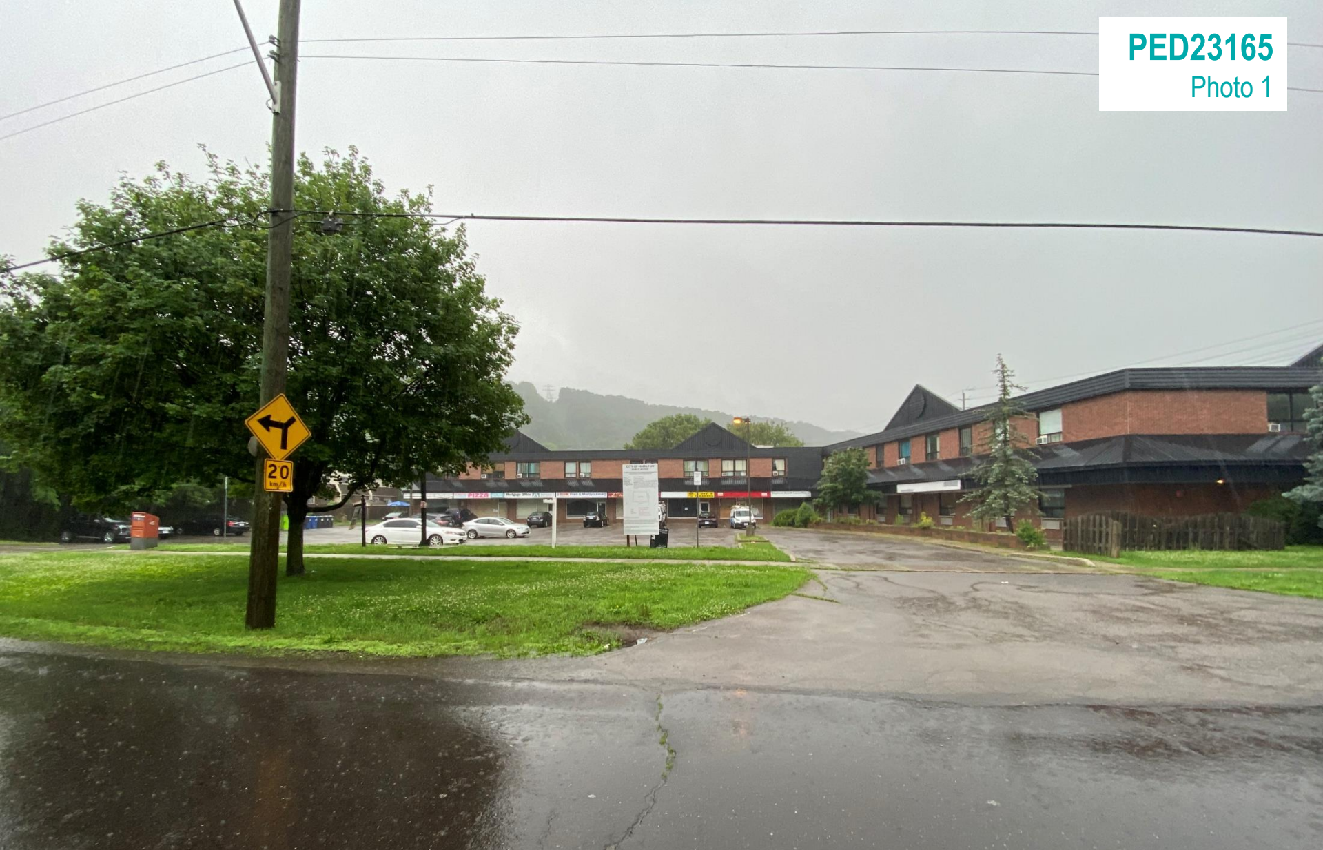
View of Subject Lands from York Road
