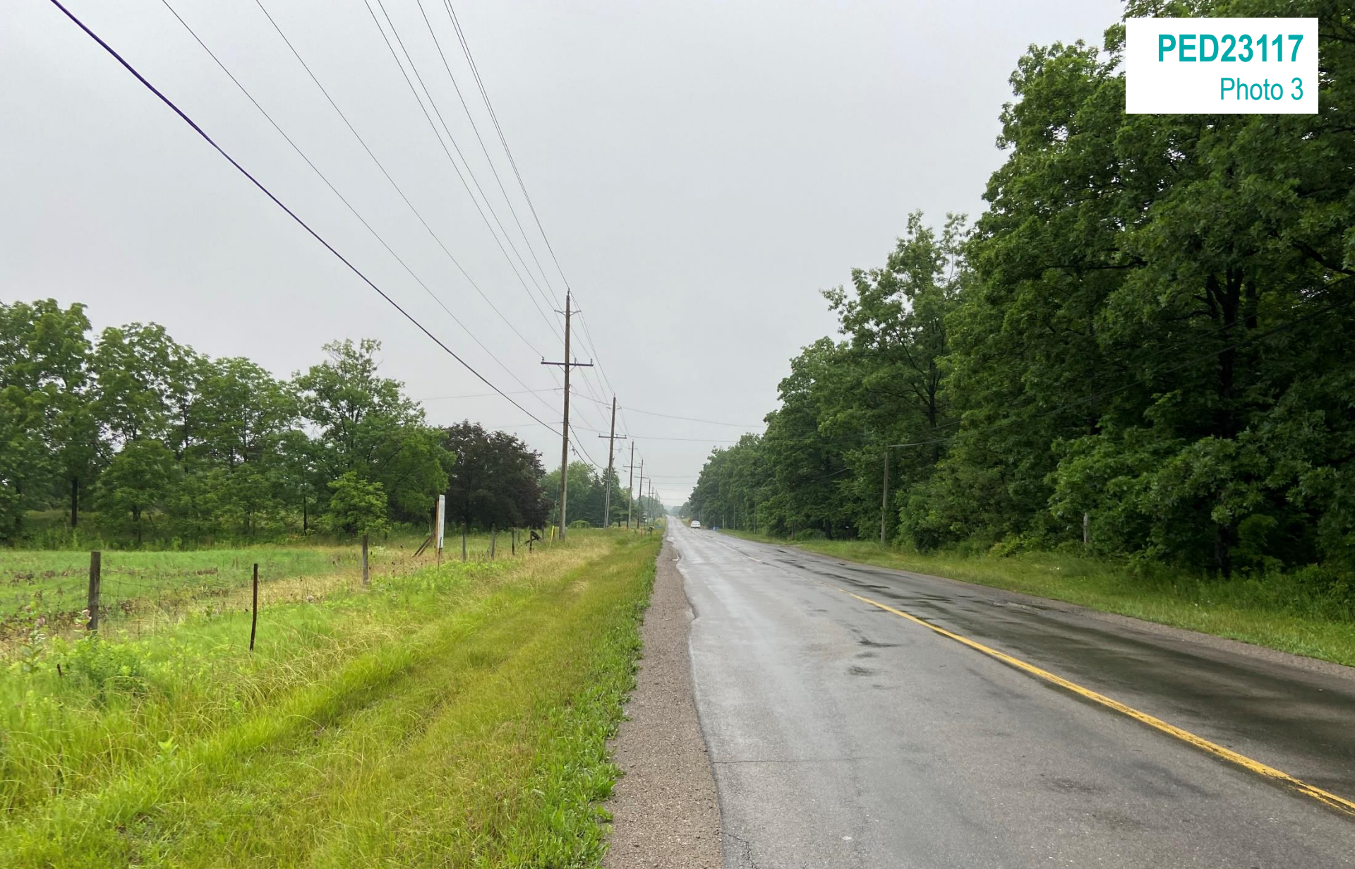
View looking West on Binbrook Road
