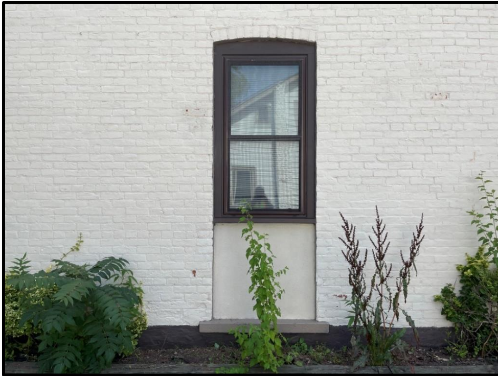
Image 19: Former Door Opening on West Elevation on 215 King Street West (Photo taken on August 6, 2021; Facing East)
