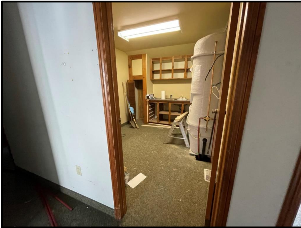
Image 57: Room in Rear Addition (Photo taken on August 6, 2021)
