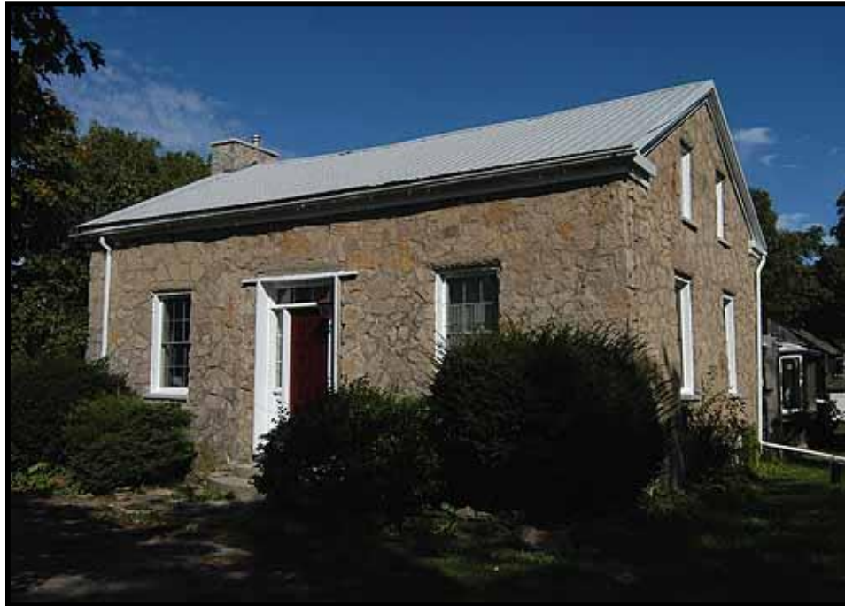
Figure 2: Cummins House, Example of a Georgian Cottage (Kyles 2016)
