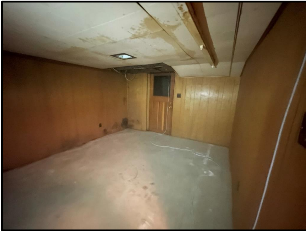
Image 75: Basement Room with Door to Closed Staircase (Photo taken on August 6, 2021)
