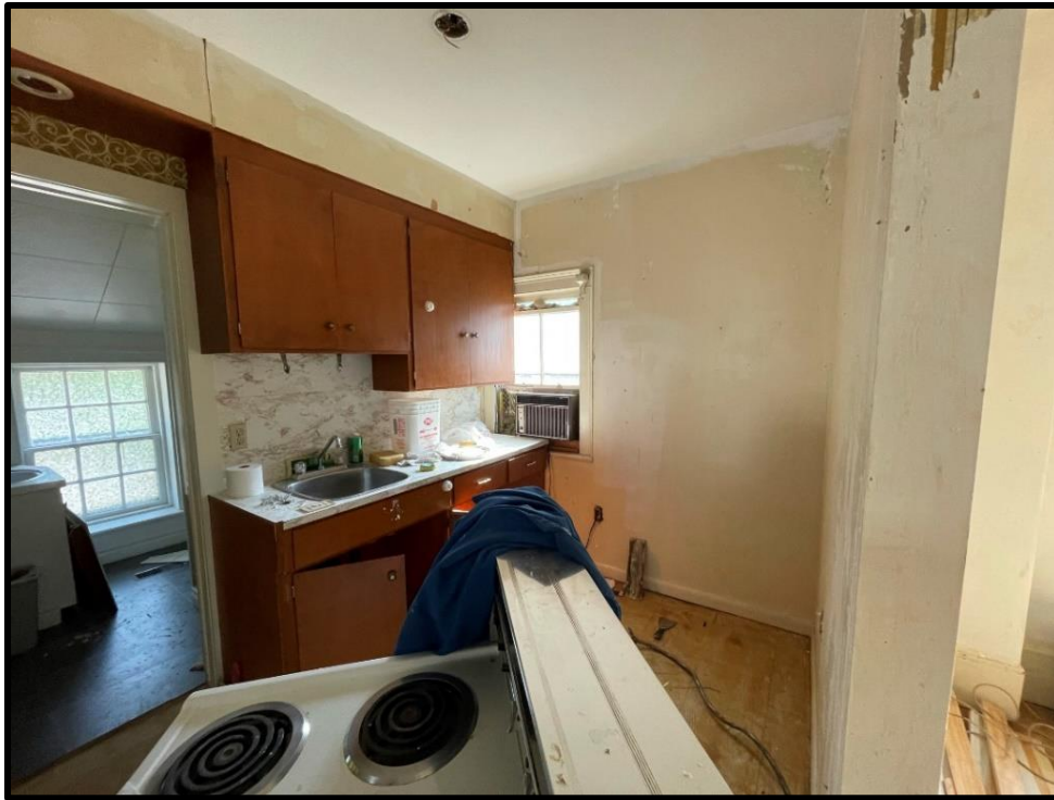
Image 63: Second Floor Kitchen Area (Photo taken on August 6, 2021)
