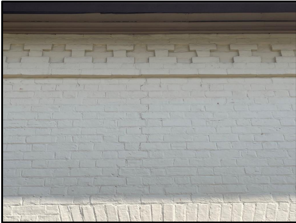
Image 5: Decorative Brickwork and Flemish Bond on 215 King Street West (Photo taken on August 6, 2021; Facing North)
