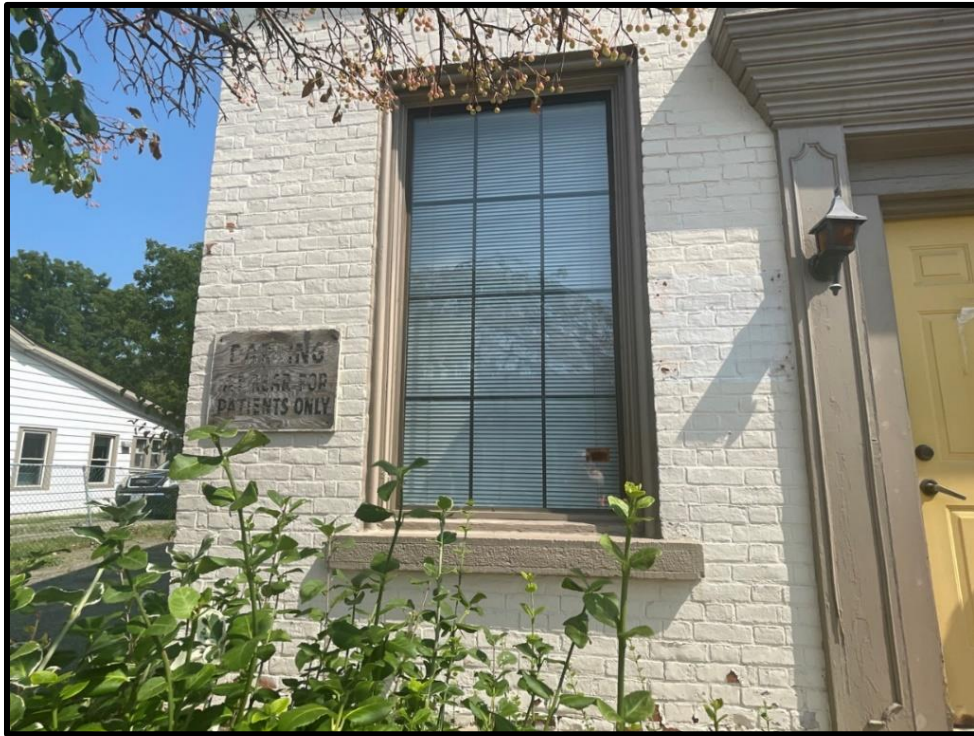
Image 9: Façade Window Opening (Photo taken on August 6, 2021; Facing North)
