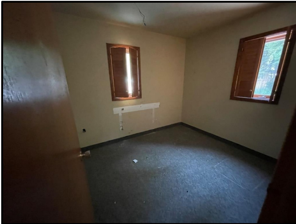
Image 58: Room in Rear Addition (Photo taken on August 6, 2021)
