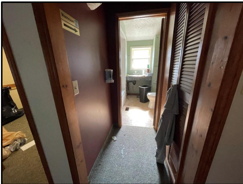
Image 60: Rear Addition Hallway (Photo taken on August 6, 2021)
