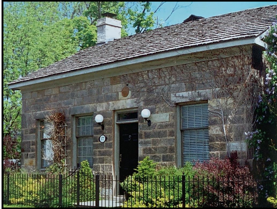
Figure 1: Hatt Street House, Example of an Asymmetrical Georgian Façade (Mikel 2004:16)
