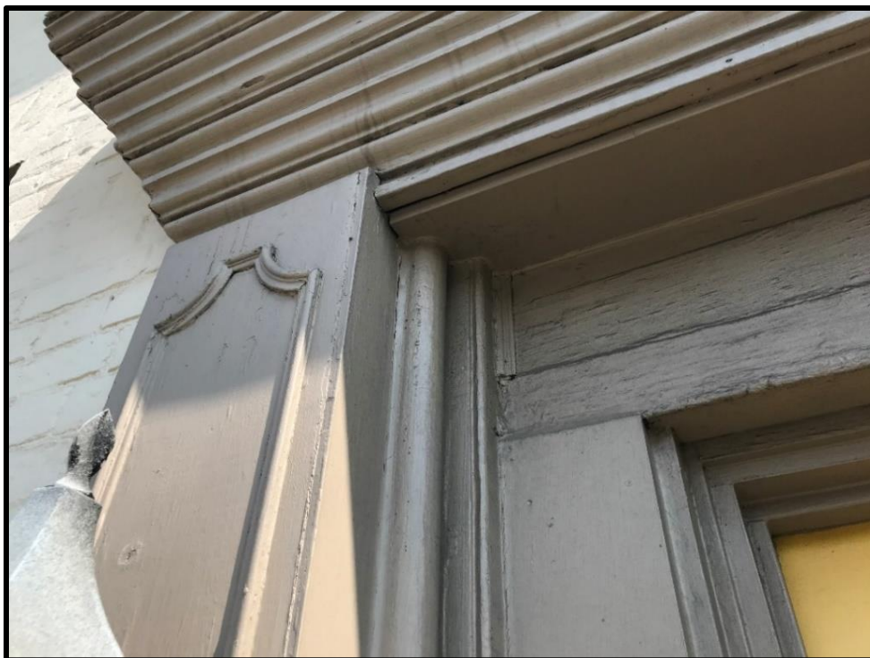
Image 8: Detail of Façade Entry Door Surround (Photo taken on August 6, 2021; Facing West)
