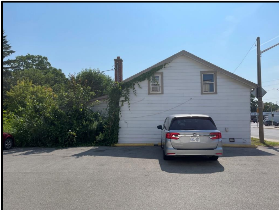
Image 28: West Elevation of 219 King Street West (Photo taken on August 6, 2021; Facing East)
