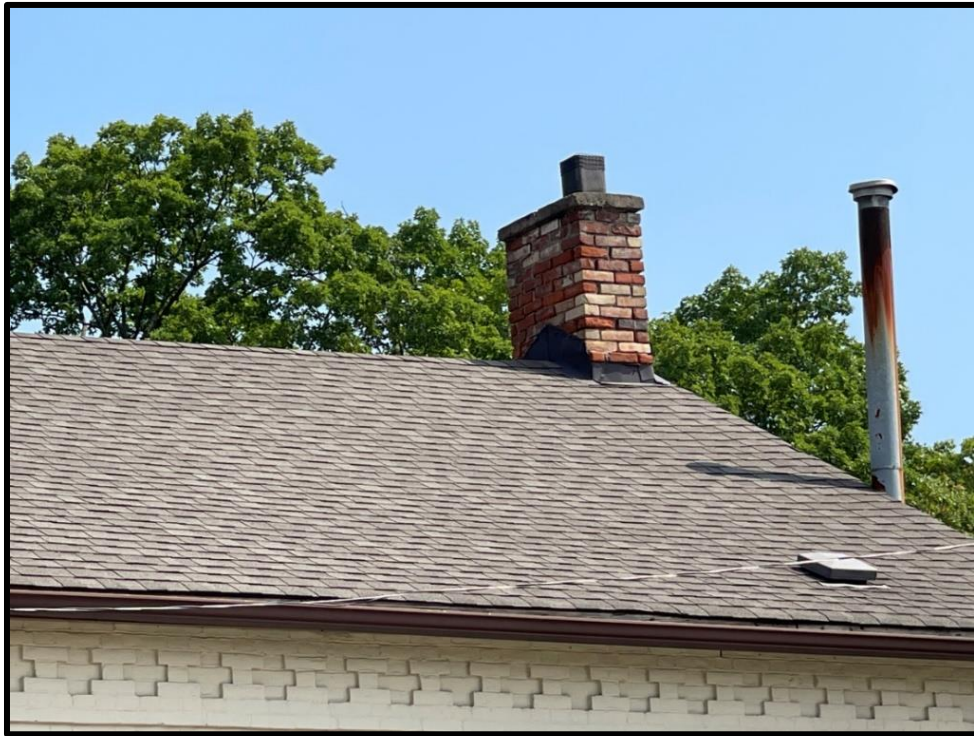
Image 3: Brick Chimney on 215 King Street West (Photo taken on August 6, 2021; Facing Northeast)
