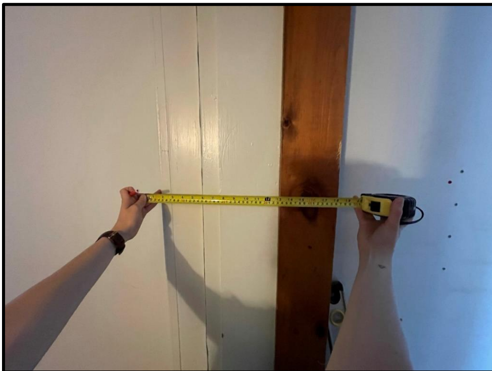
Image 54: Interior – Wall Thickness Between Brick Building and Rear Addition (Photo taken on August 6, 2021)
