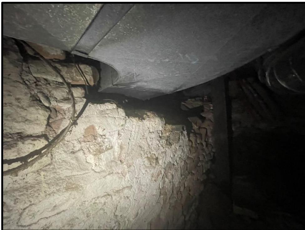
Image 74: Basement Showing Crawlspace Under Rear Addition (Photo taken on August 6, 2021)
