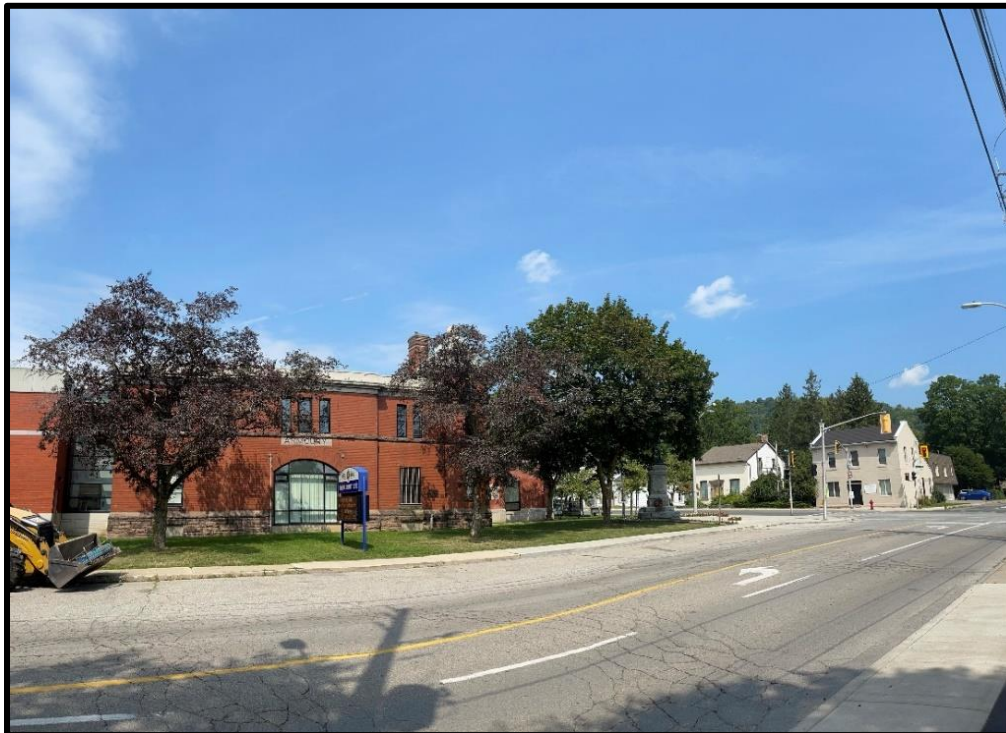
Image 40: 10 Market Street South (The Dundas Armoury) – Study Area Visible (Photo taken on August 6, 2021; Facing West)
