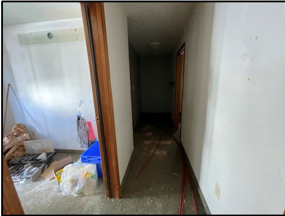
Image 55: First Floor, Rear Addition Hallway (Photo taken on August 6, 2021)
