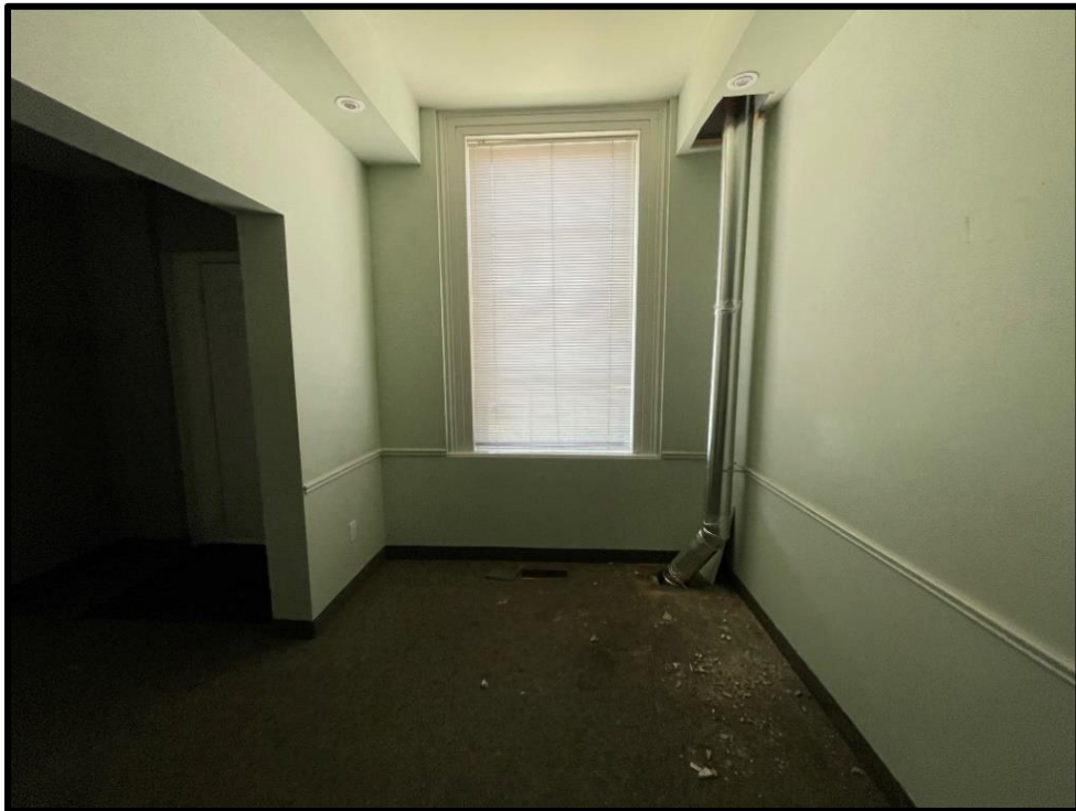
Image 48: West Window Opening on Façade (Photo taken on August 6, 2021)
