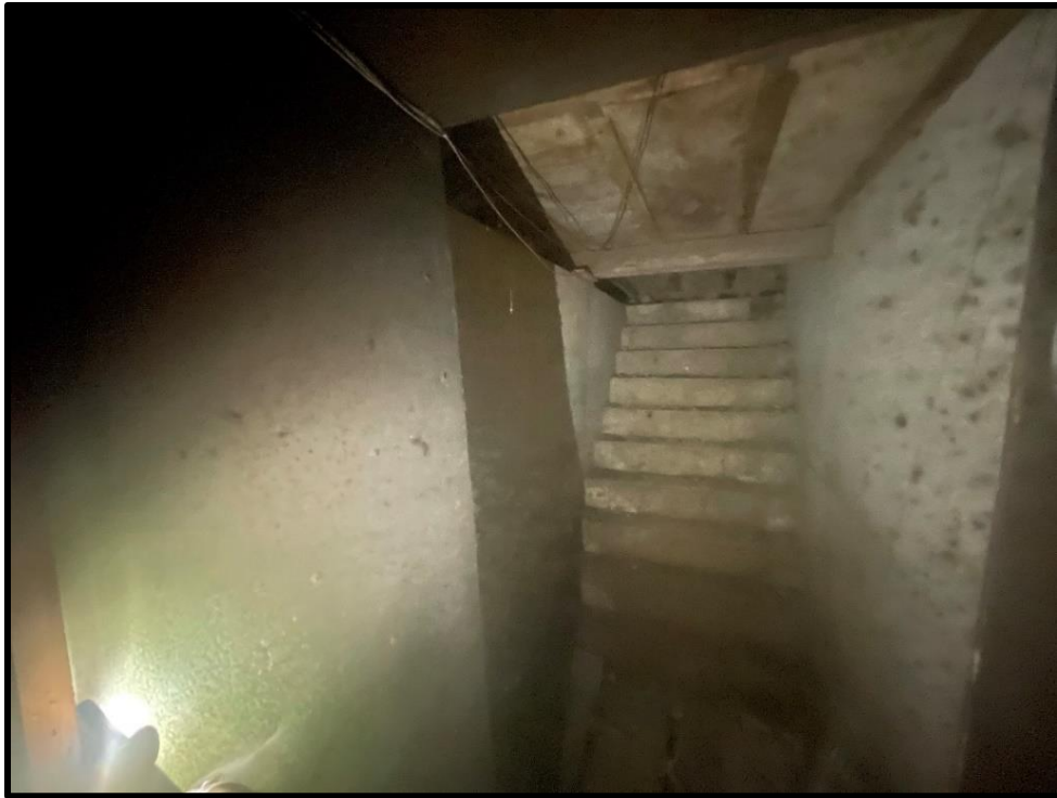
Image 77: Closed Stairwell in Basement (Photo taken on August 6, 2021)
