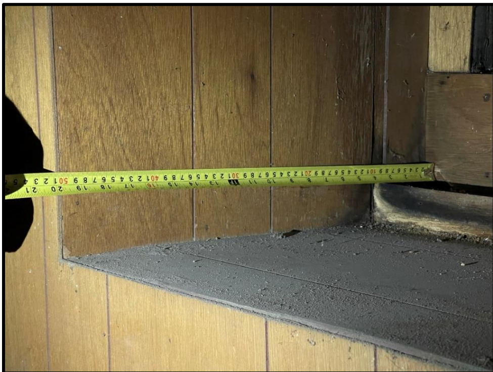
Image 80: Depth of Basement Window Well (Photo taken on August 6, 2021)
