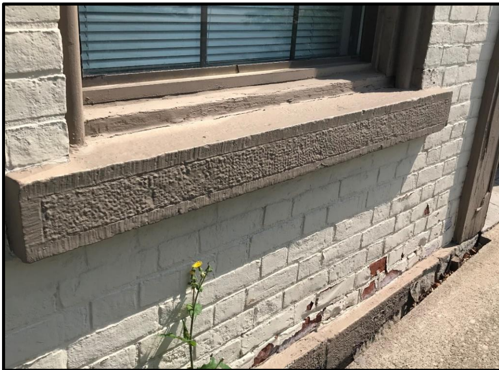
Image 10: Rusticated Sill on 215 King Street West Façade (Photo taken on August 6, 2021; Facing North)
