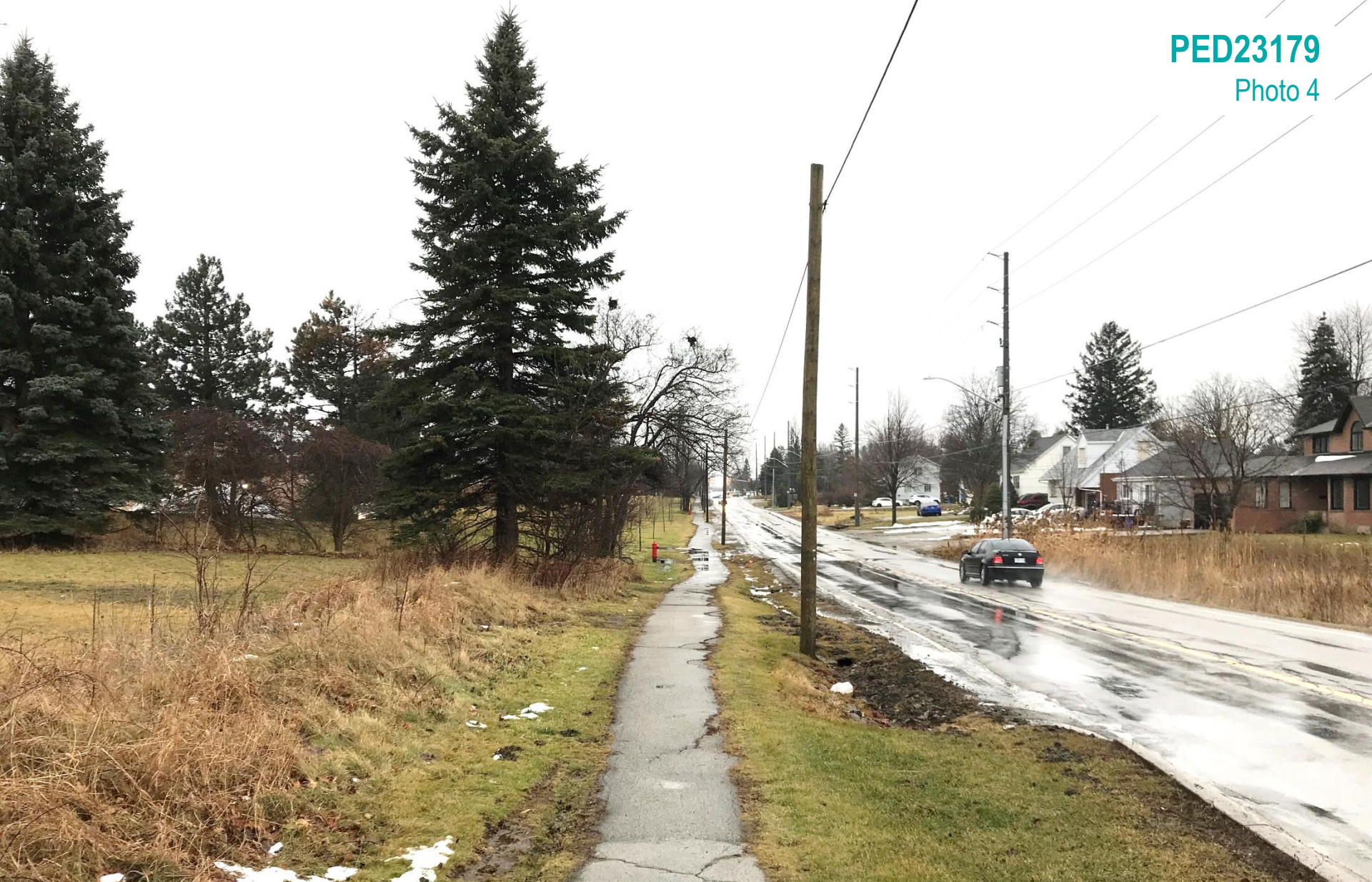
West 5th Street – Looking South
