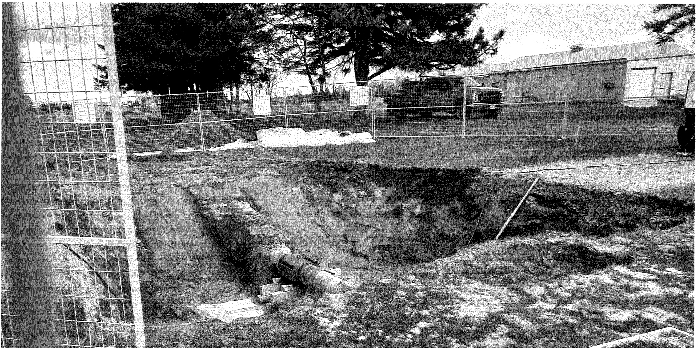
Imperial Oil Line Repair Sleeve on borderline of 1142/1164 Properties, April 17, 2022. Several hundred feet of pipeline were eventually replaced in this area. (taken by Ron Sealey on phone)
