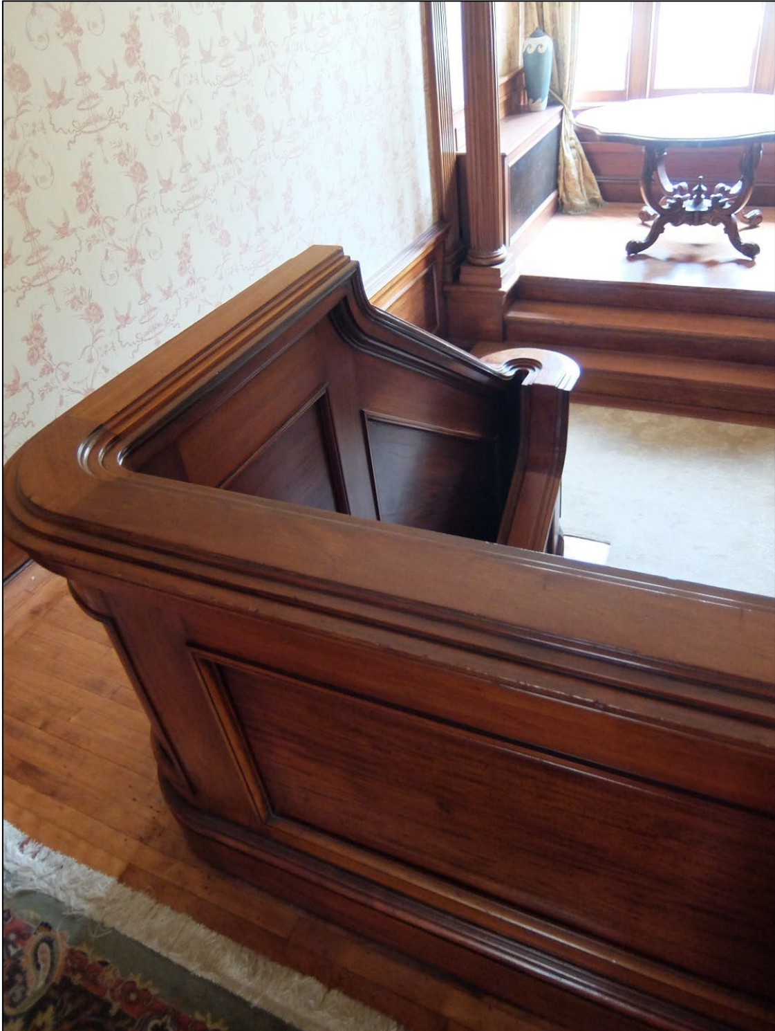
Closeup of carved wood handrail and paneling in second-storey of main stairway
