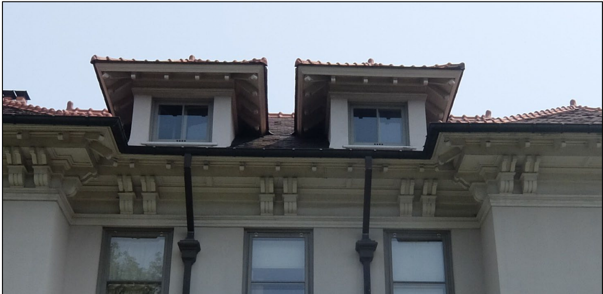
Closeup of hipped roof dormers with red clay tiles
