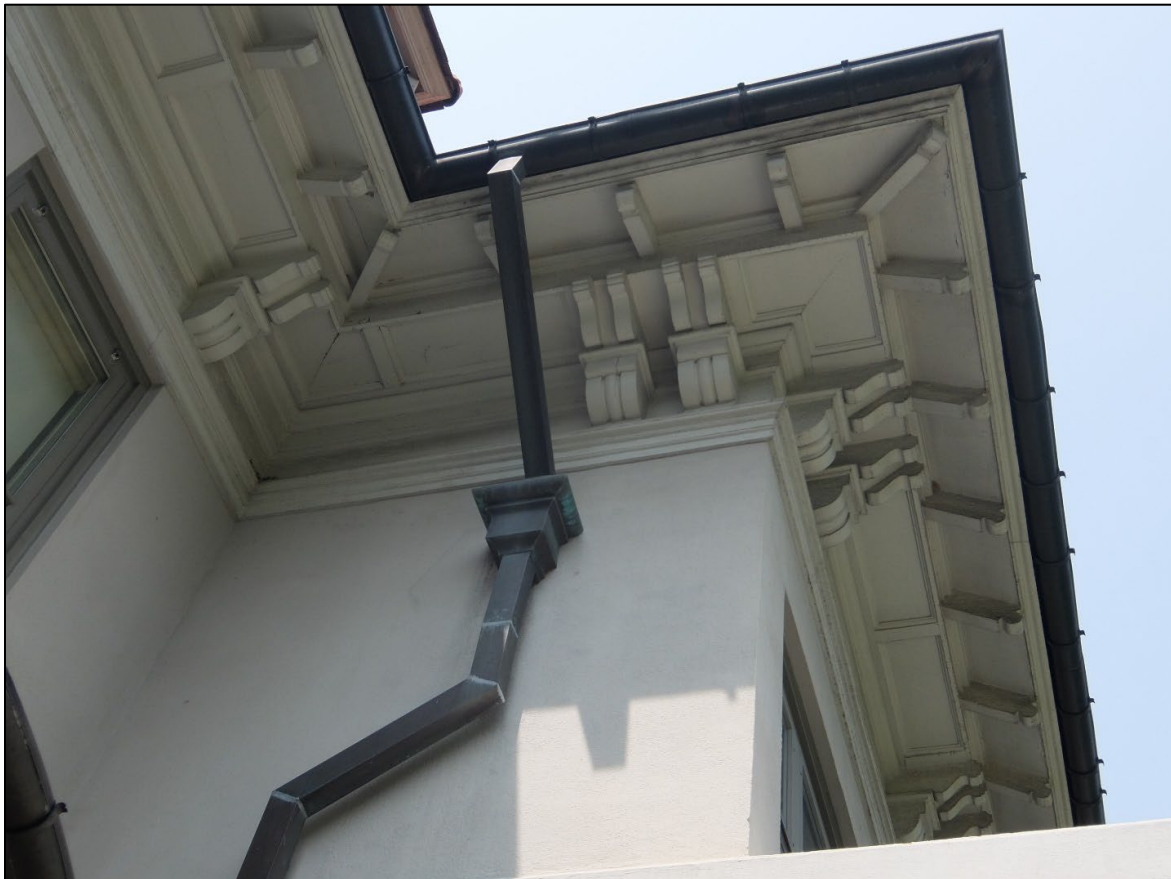
Closeup of paired bracketed eaves, moulded frieze, and copper downspout
