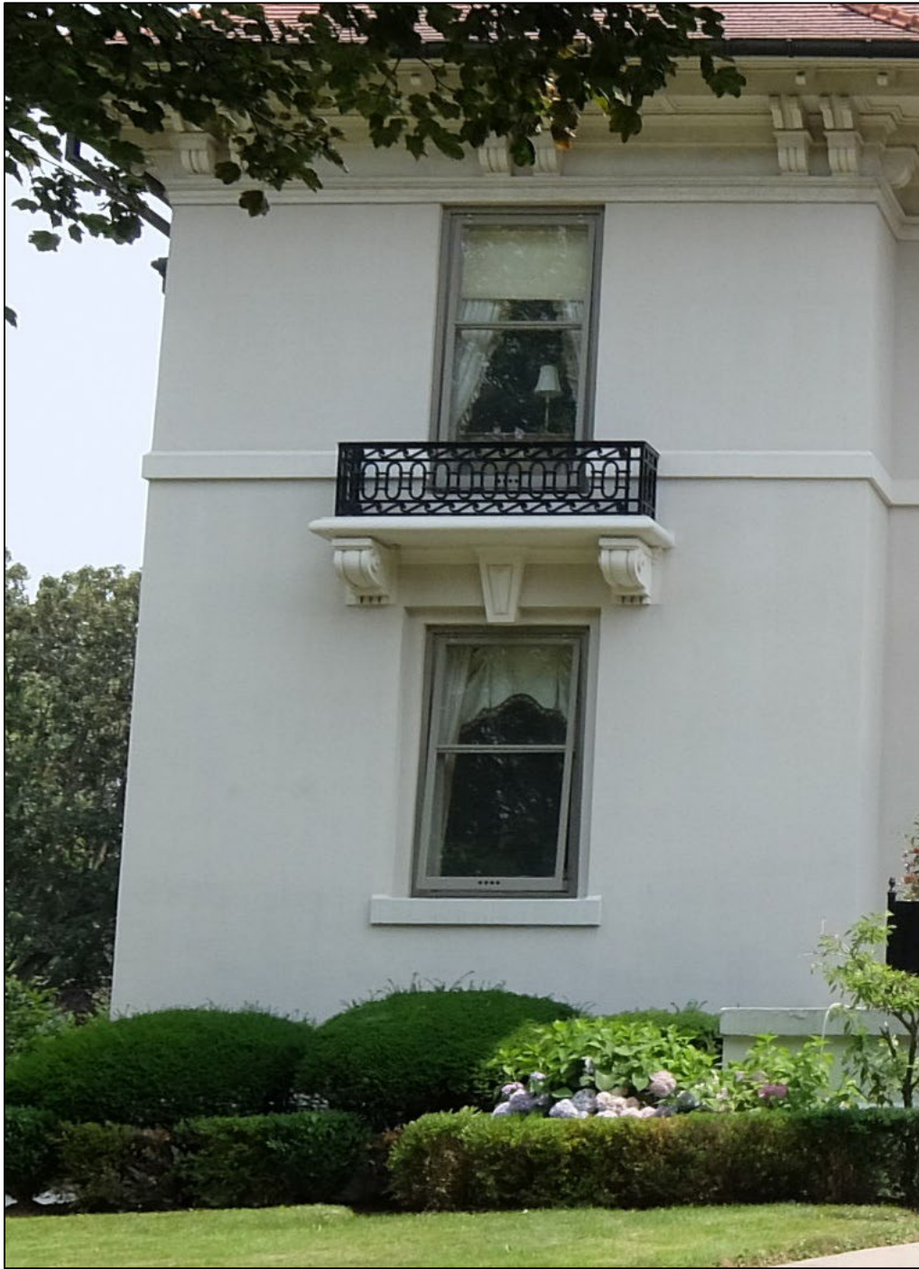
Closeup of balconet with wrought-iron railings, corbels, and decorative keystones
