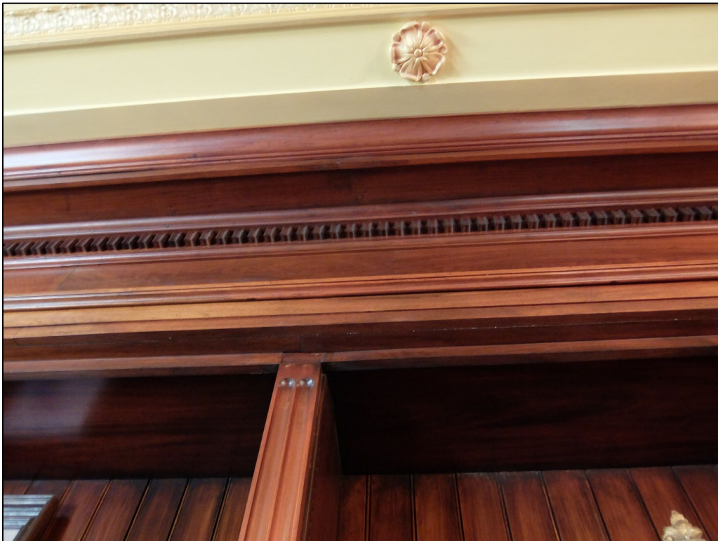
Closeup of library wood carved crown moulding with dentils and plaster ceiling rosette
