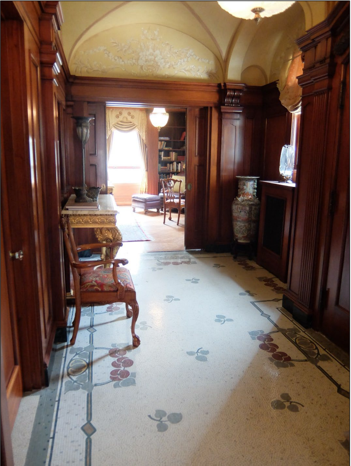
Wood paneled front foyer with cross vaulted ceiling, carved wood pilasters, and double brackets
