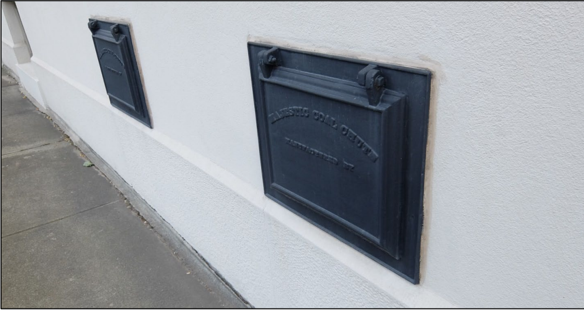
Closeup of coal chutes
