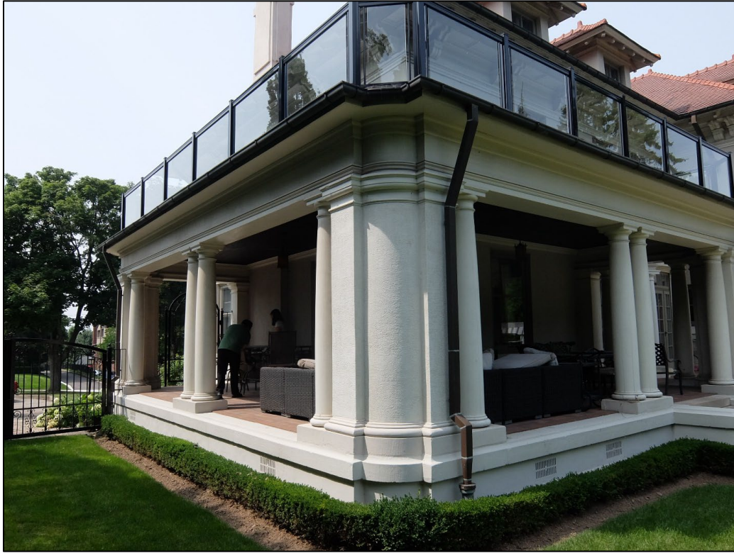
Southeast elevation showing the covered south side porch
