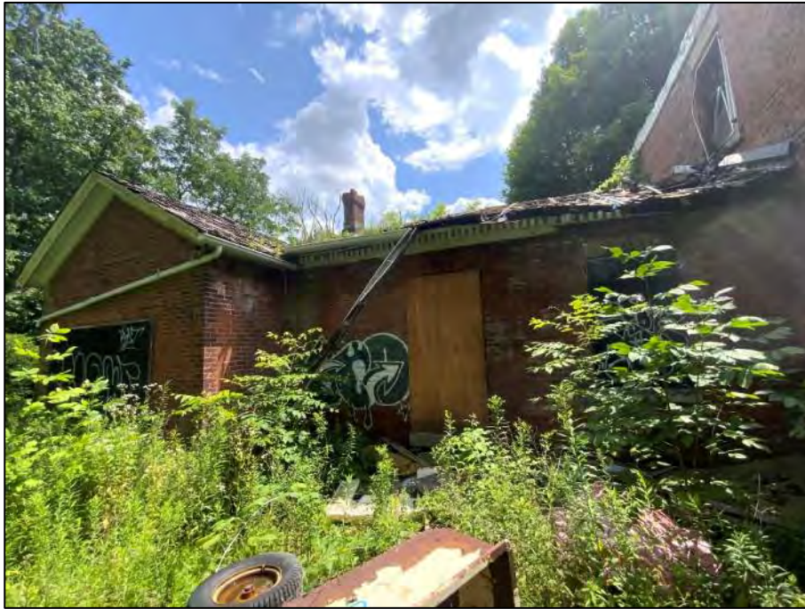
Photograph 1: Rear Link Roof
