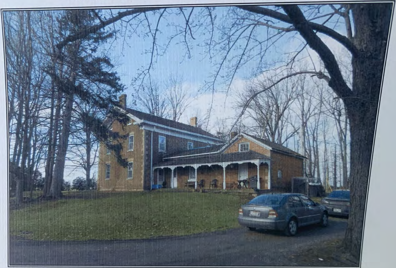
South and East Walls of Home
