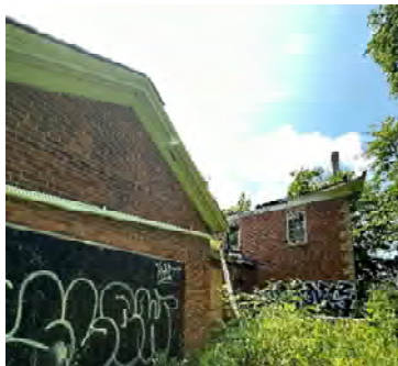
Figure 20 View of the existing chimney at the front of the building.
