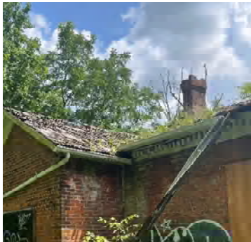
Figure 19 View of the existing chimney at the rear of the building.
