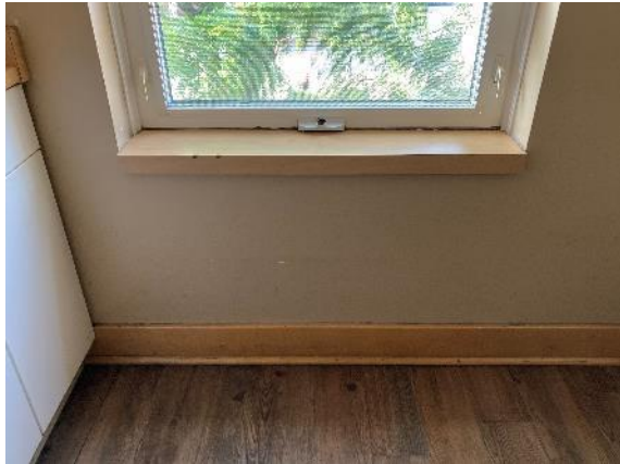
Image 69: Detail of flooring, baseboard and window casing in second floor kitchenette
