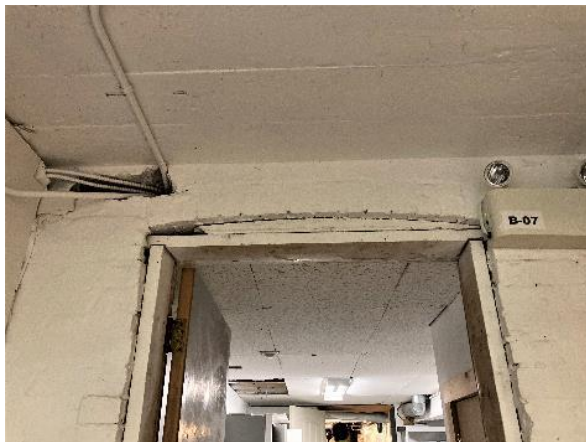
Image 89: Detail of brick segmentally arched door opening in brick wall in basement
