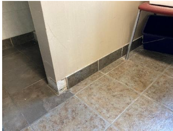
Image 66: Detail of tile flooring in second floor bathroom
