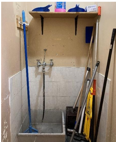
Image 67: Detail of janitors closet on second floor
