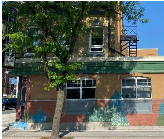
Image 35: Detail of east elevation, note addition and contemporary cladding
