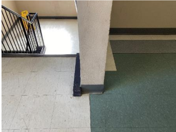
Image 53: Detail of contemporary construction material in stairwell
