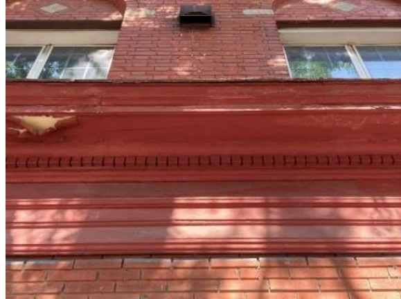
Image 105: Projecting moulded, dentilated cornice on east elevation
