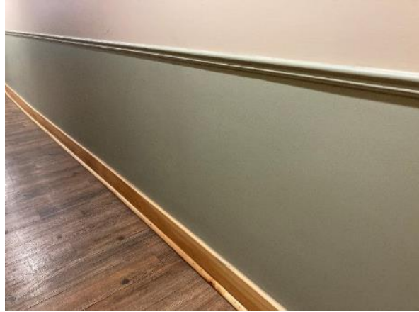
Image 58: Chair rail and baseboards in second floor hallway
