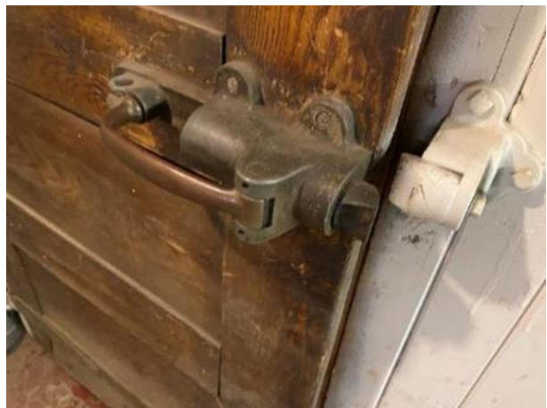
Image 98: Detailed view of cold storage door hardware
