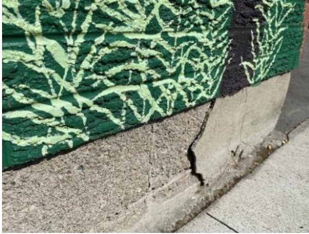
Image 38: Detail of CMU foundation of north addition
