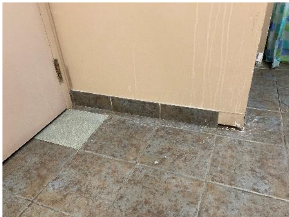
Image 79: Detail of tile flooring in third floor bathroom
