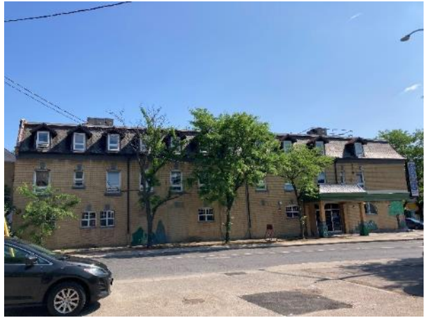
Image 4: South elevation of subject property
