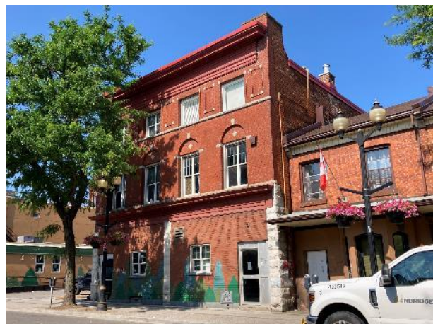
Image 121: Northeast corner of 325 James Street North
