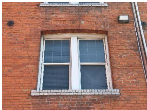
Image 115: Detail of segmentally arched window in south elevation with brick lintel and sill
