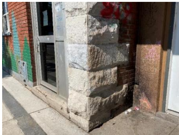
Image 103: Cut stone quoins on corner of east elevation
