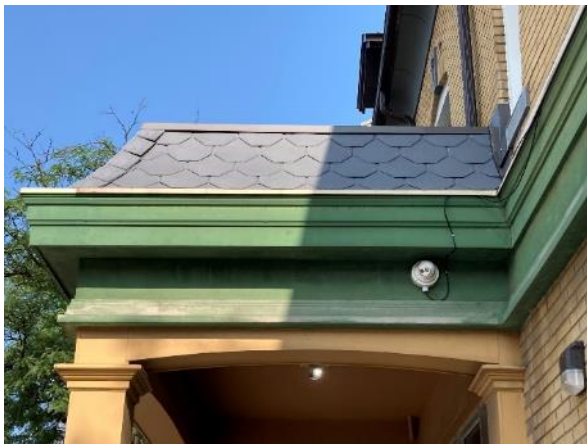
Image 19: Slate tile mansard roof of portico on south elevation looking west
