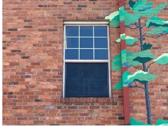
Image 111: Nine-over-one window in south elevation of addition
