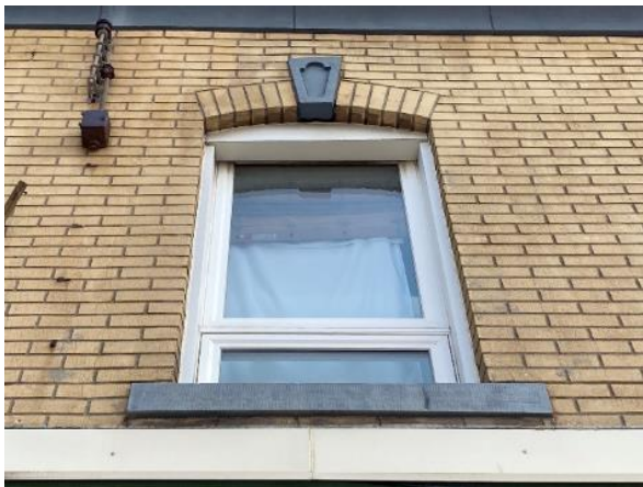
Image 17: Detail of tooled stone window sill and keystone on upper level of south elevation
