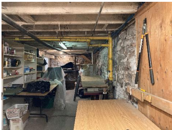
Image 91: View of unfinished basement room with exposed stone foundation and trusses
