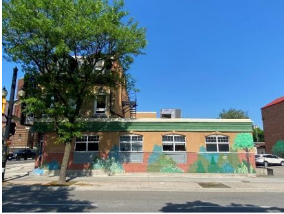
Image 32: East elevation of subject property
