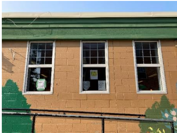
Image 29: Detail of vinyl windows in north elevation of addition
