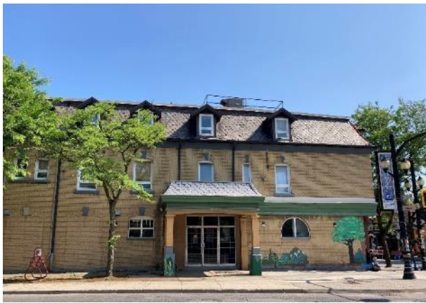
Image 11: Detail of fenestration on east side of south elevation
