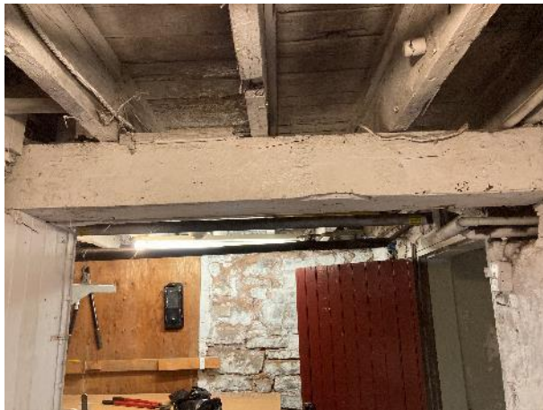
Image 95: View of dimensional timber floor joists and wood plank subflooring
