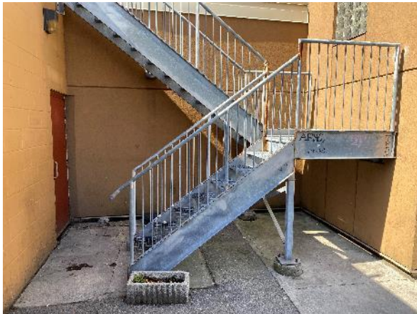
Image 28: Detail of fire escape on north elevation
