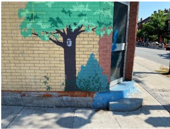
Image 5: Foundation at east side of south elevation
