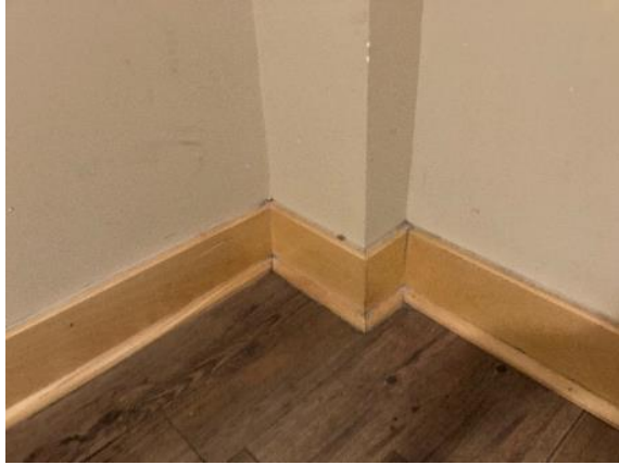
Image 63: Representative baseboard and quarter round in second floor bedroom
