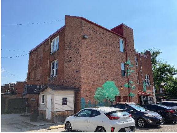
Image 116: Southwest corner of 325 James Street North
