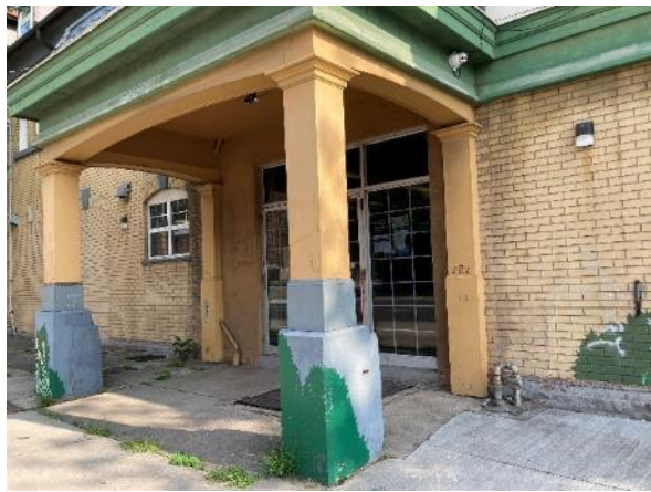
Image 20: Detail of portico pillars and concrete support base
