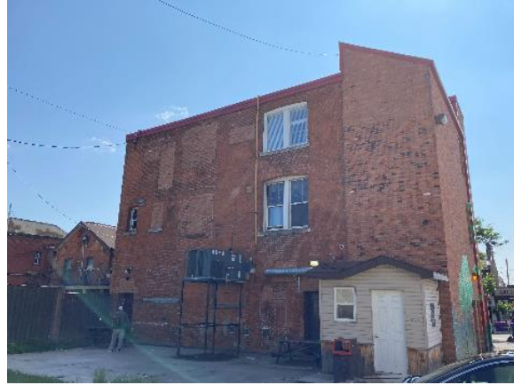
Image 117: West elevation of 325 James Street North
