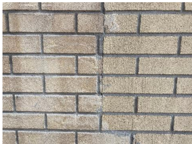
Image 2: Brick veneer on south elevation, to left note replacement material over enclosed window opening
