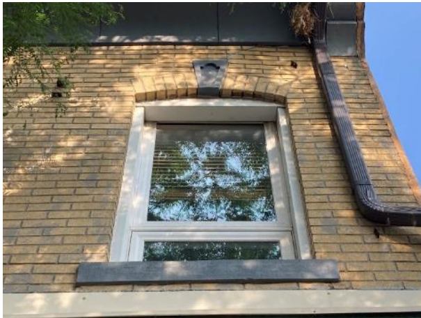
Image 34: Detail of upper storey window on east elevation
