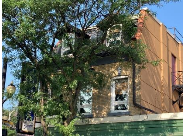
Image 33: Detail of upper storey fenestration of east elevation
