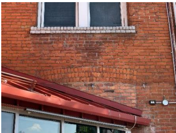
Image 114: Detail of enclosed window behind entrance addition on south elevation
