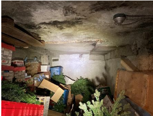
Image 99: View of concrete cold storage room
