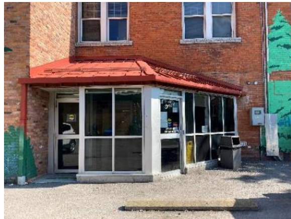
Image 113: Projecting entranceway in south elevation
