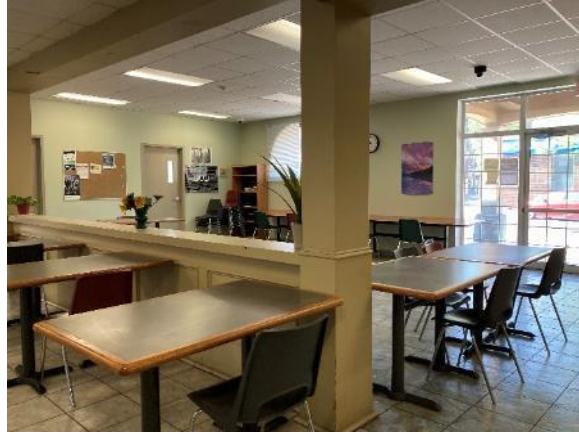
Image 40: View across the communal dining area, note beams marking division between original block and addition
