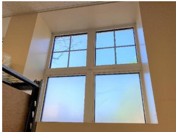
Image 48: Recessed window opening in south wall of kitchen
