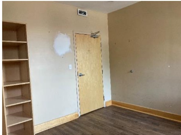
Image 60: Representative view of a second floor bedroom looking northeast
