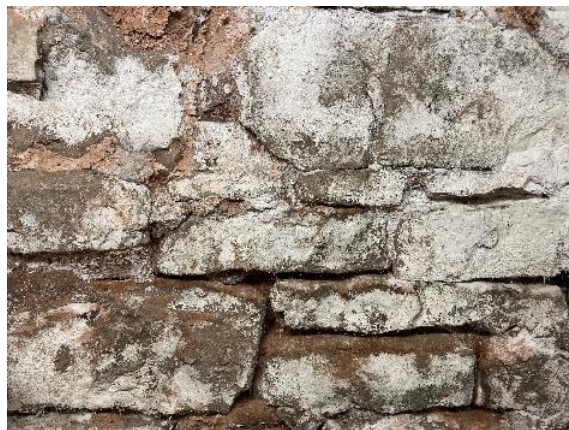
Image 92: Detail of limestone and fieldstone foundation
