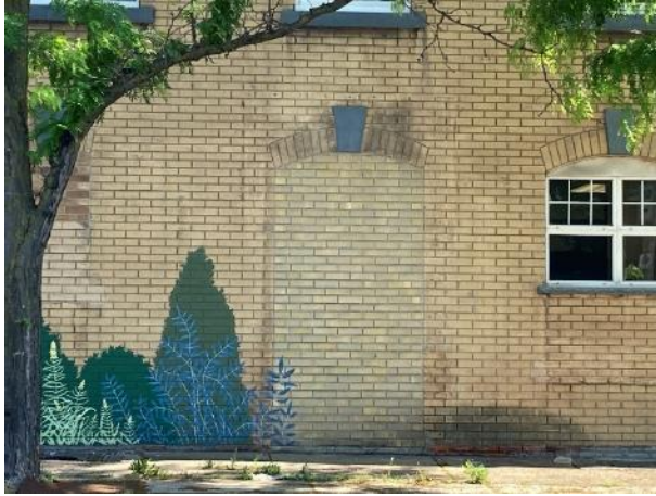
Image 15: Detail of brick-enclosed window opening on ground level of south elevation
