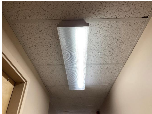
Image 56: Detail of drop ceiling in upper floor hallway
