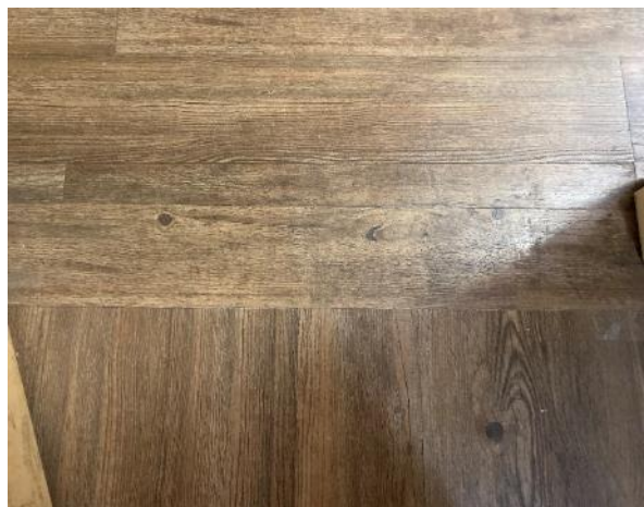
Image 62: Vinyl flooring in second floor bedroom
