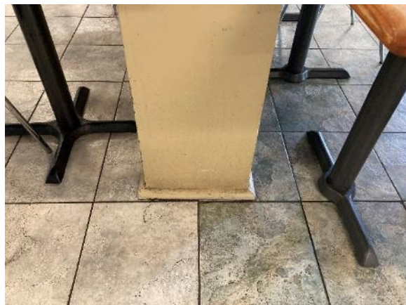
Image 44: Representative example of flooring and baseboards on main level
