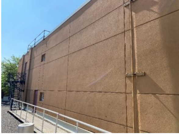
Image 26: Detail of stucco cladding on north elevation of original block
