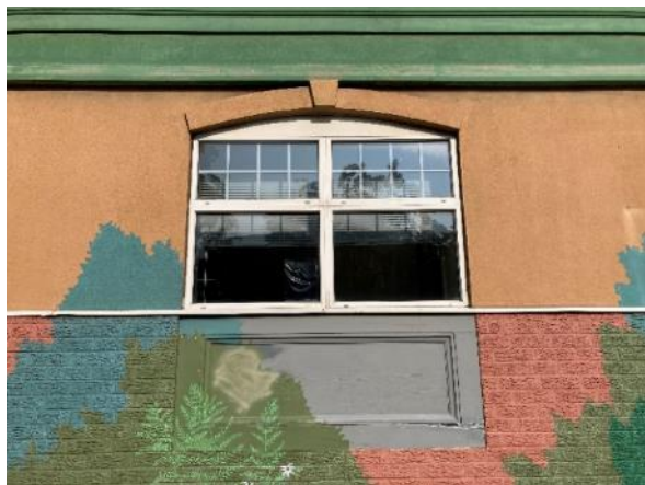
Image 37: Detail of cornice and contemporary window detailing on east elevation
