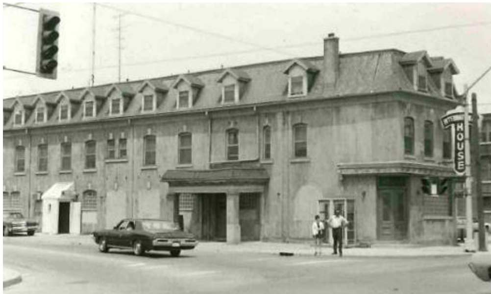
Plate 2: International Hotel, ca. pre-1970s (City of Hamilton, n.d.b)
