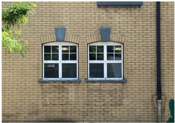
Image 12: Detail of segmentally arched window openings on ground level of south elevation
