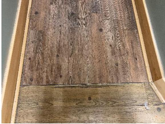
Image 57: Detail of vinyl flooring and simple baseboards in upper floor hallway
