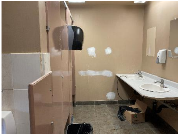
Image 77: Third floor bathroom looking west
