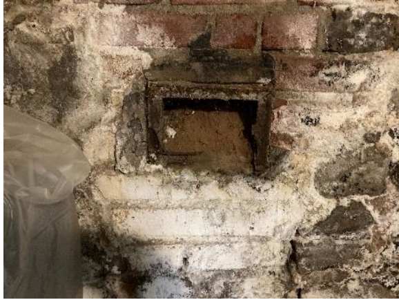
Image 93: Coal chute in bricked portion of foundation
