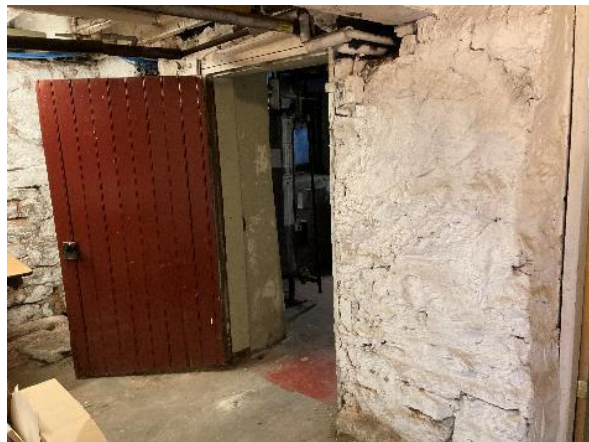
Image 90: View of exposed stone foundation in basement
