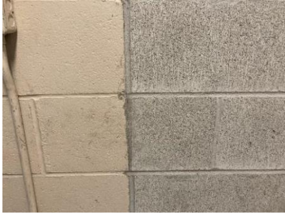
Image 51: Detail of CMU construction of stairwell
