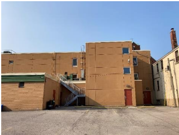
Image 24: West side of north elevation of subject property
