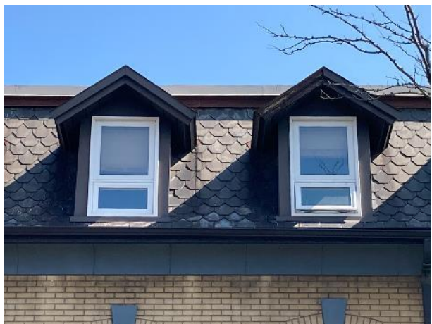
Image 8: Detail of mansard roof with dormer windows
