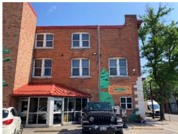
Image 109: East side of south elevation of 325 James Street North
