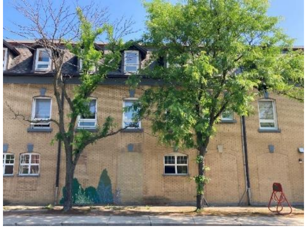
Image 10: Detail of fenestration on centre of south elevation
