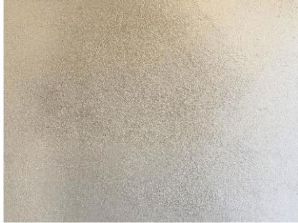
Image 52: Detail of plaster cladding of stairwell walls
