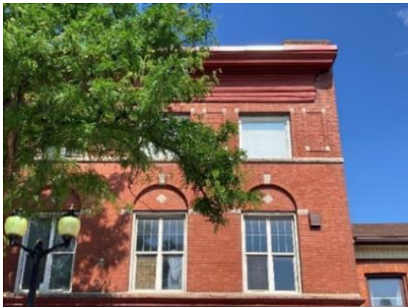
Image 106: Detail of upper storey of east elevation
