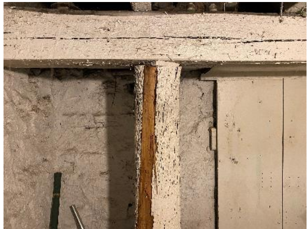
Image 96: Detail of timber support beam
