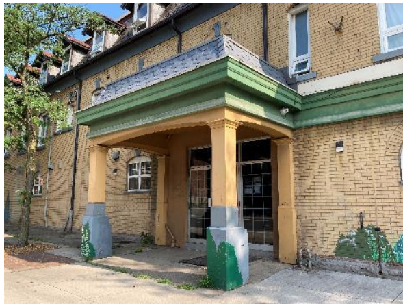
Image 18: Detail of portico on south elevation
