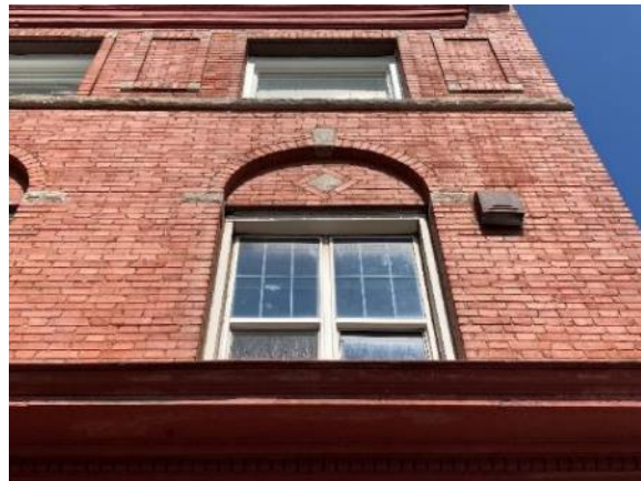
Image 107: Detail of upper storey fenestration of east elevation
