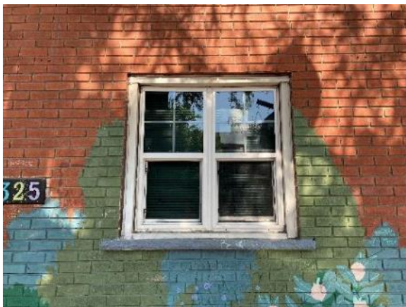
Image 102: Detail of ground level replacement window on east elevation
