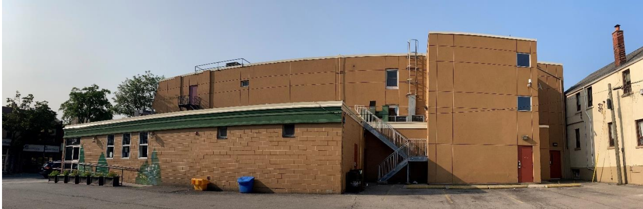
Image 23: North elevation of subject property
