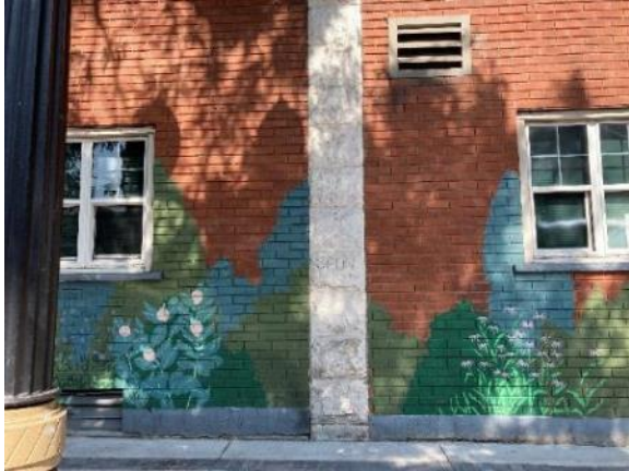
Image 104: Cut stone decorative column on east elevation
