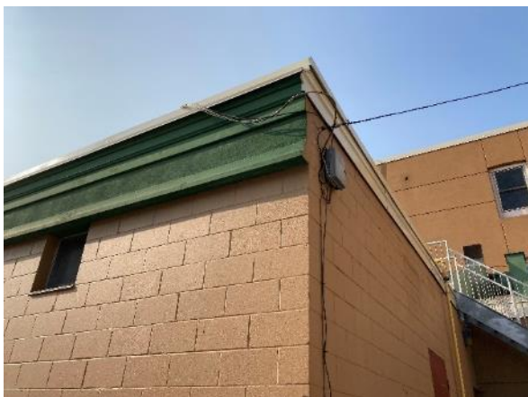
Image 30: Detail of CMU construction and cornice of north addition
