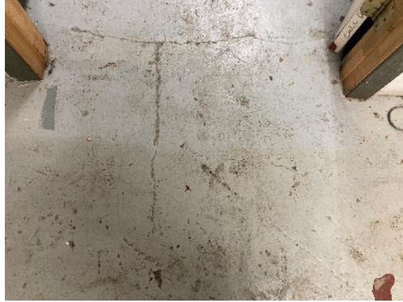
Image 94: Detailed view of concrete floor in basement
