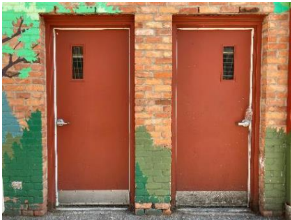
Image 112: Two steel doors in south elevation of addition
