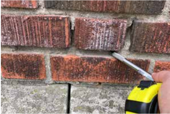
Fig. 10. Recessed mortar joints.
