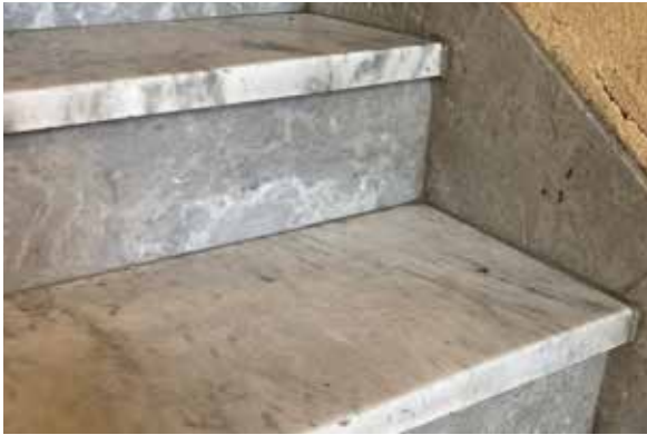
Fig. 107. Original marble stairs in good condition.
