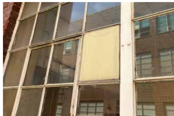
Fig. 55. Infilled window lite.
