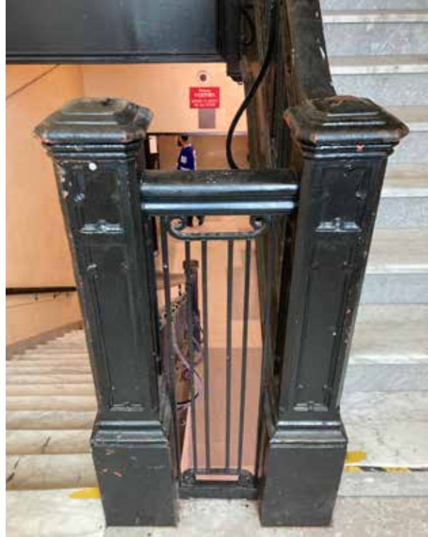
Stairway landing newel posts.
