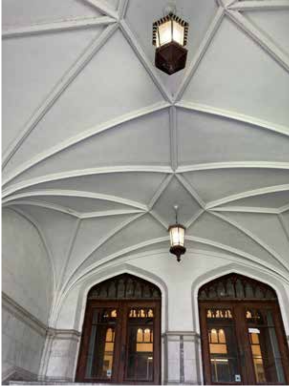
Front entrance and doorways.
