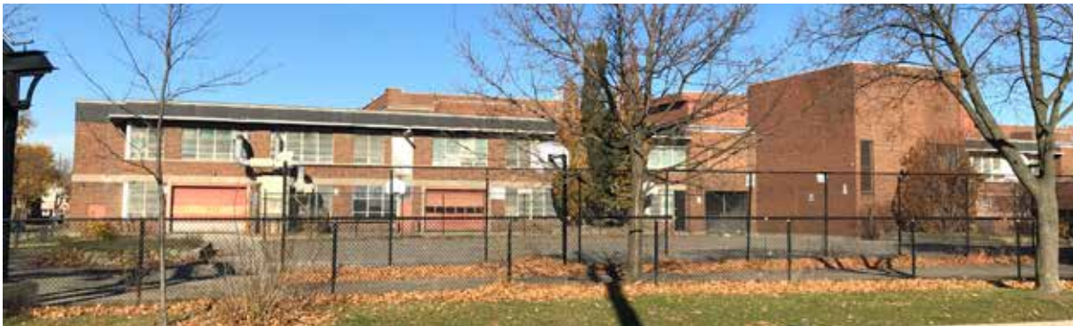
South elevation - 1948-50 South Wing and 1970 addition (near right).
