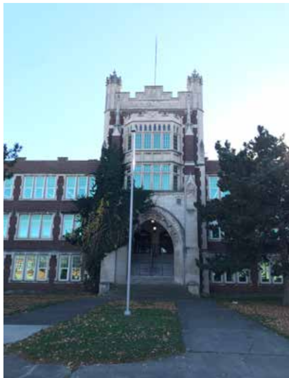
1924 School Building, north elevation tower.
