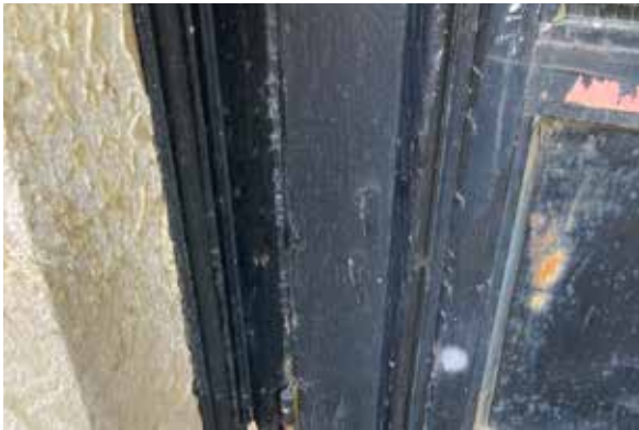
Fig. 90. Paint deterioration.
