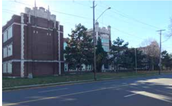
1924 School Building, north elevation.
