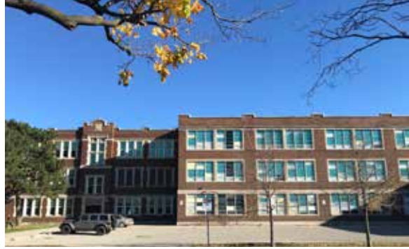
West elevation - 1924 School Building (left) and 1948-50 Southwest Wing (right).
