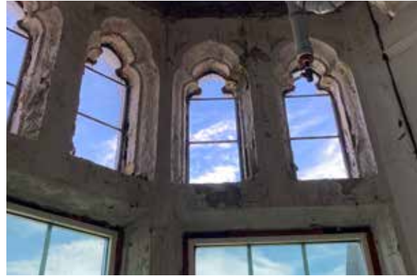
Fig. 42. Trefoil arched openings with original glazing.
