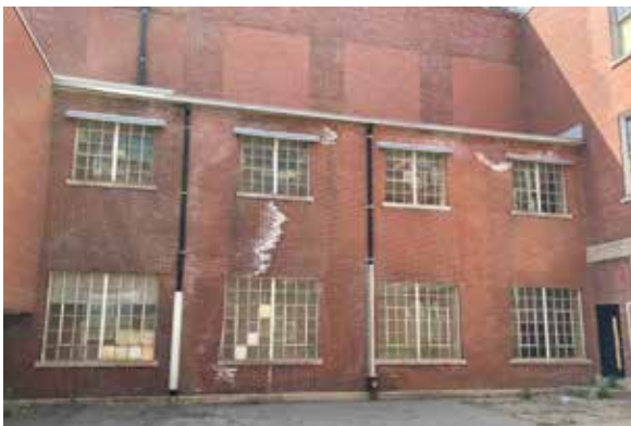
Fig. 46. Brick infill of pre-existing clerestory.
