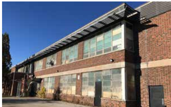
South elevation - 1948-50 South Wing.
