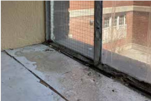
Fig. 57. Overpainting of steel frames.
