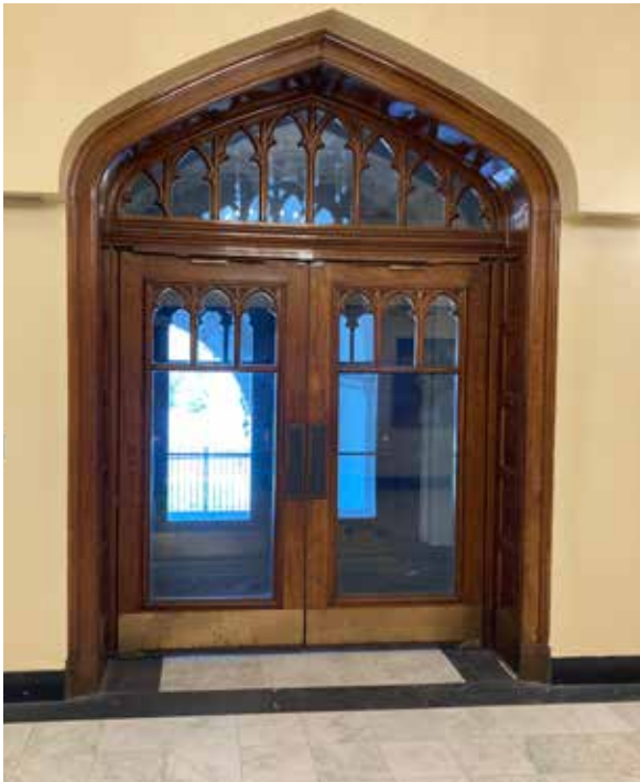
Interior front entrance vestibule doorway.
