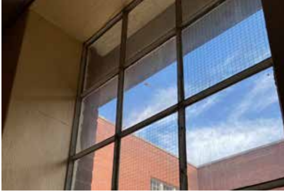
Fig. 56. Replaced window lites.
