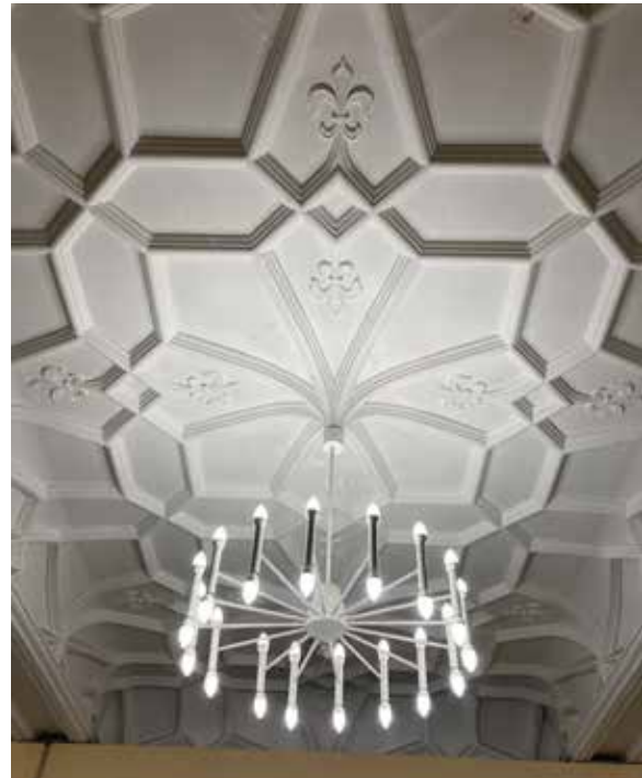
Front entrance lobby plaster ceiling.
