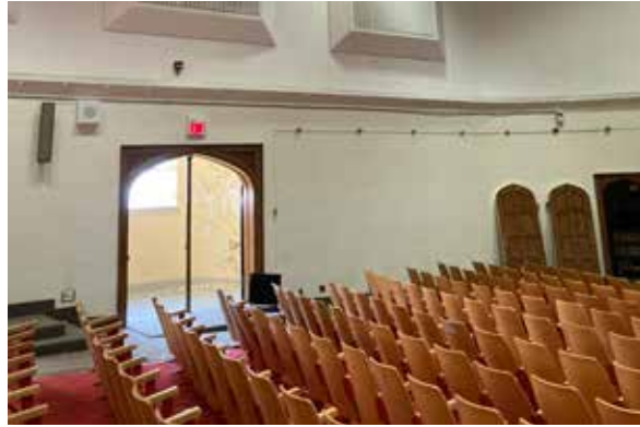
Fig. 99. Auditorium interior with original door surrounds.
