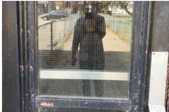
Fig. 87. Wired safety glass panel infill.
