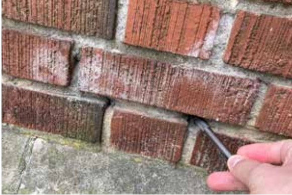
Fig. 9. Recessed mortar joints.
