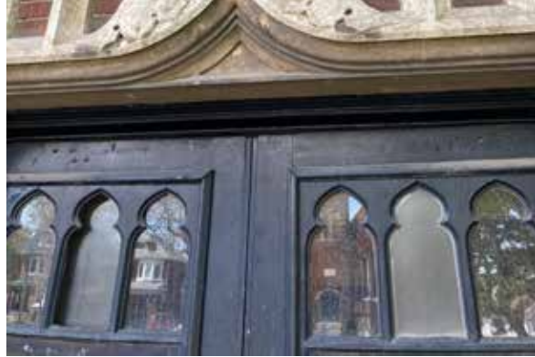
Fig. 85. Replaced transom lites.
