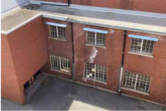
Fig. 51. Added flashings and PVC downspout.
