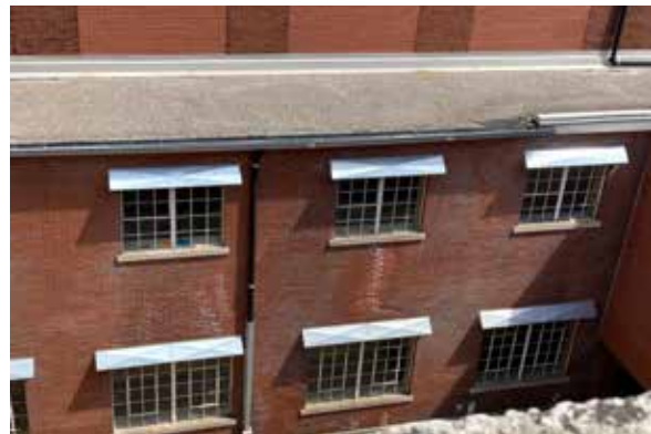
Fig. 50. Added flashings over first floor windows.
