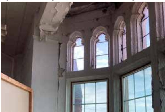
Fig. 41. Trefoil arched openings with original glazing.
