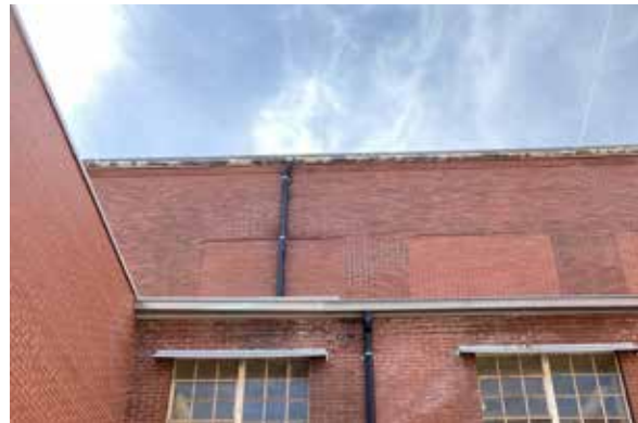
Fig. 49. Added flashings over first floor windows.
