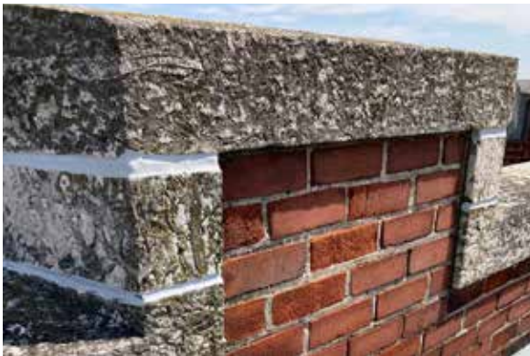
Fig. 64. Replaced mortar joint.
