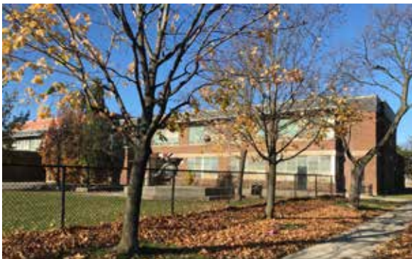
South elevation - 1948-50 South Wing.
