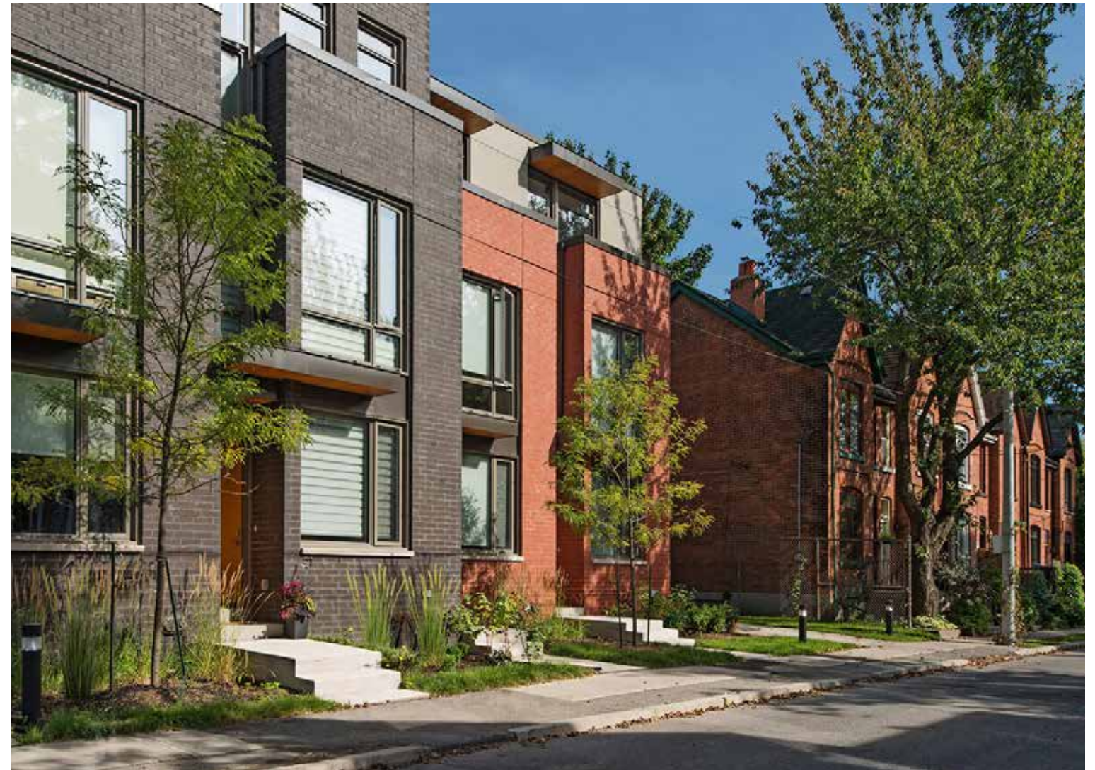
Precedent - Contemporary townhouses reference varied masonry material palette (TACT Architecture, Riverdale Towns, Toronto)
