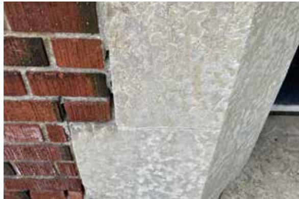
Fig. 8. Recessed mortar joints between stone and brick.
