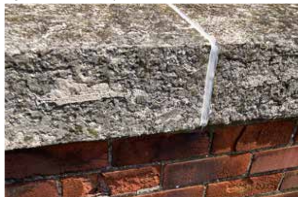
Fig. 62. Replaced mortar joint.
