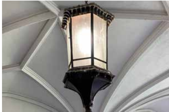
Fig. 39. Minimal soiling on outer surface of pendant light.
