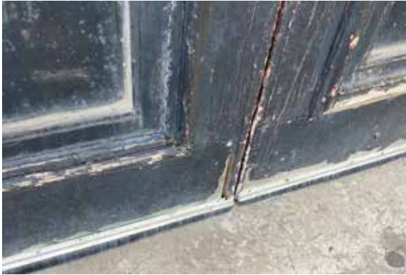
Fig. 89. Paint deterioration.
