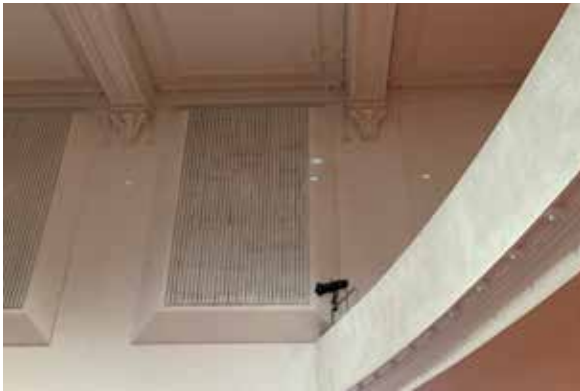
Fig. 102. Infilled windows.
