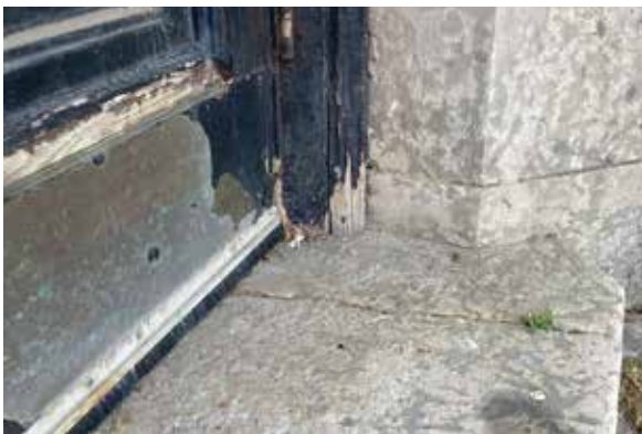
Fig. 91. Paint deterioration.
