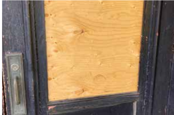
Fig. 86. Plywood pane infill.
