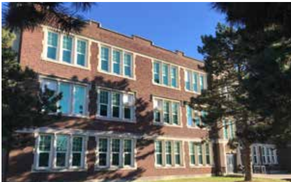
1924 School Building, west elevation.
