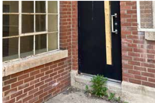
Fig. 43. Cast in place concrete base wall.
