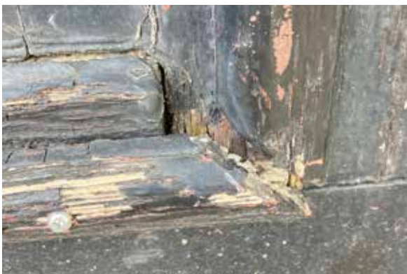
Fig. 92. Separated moulding attached via screw.
