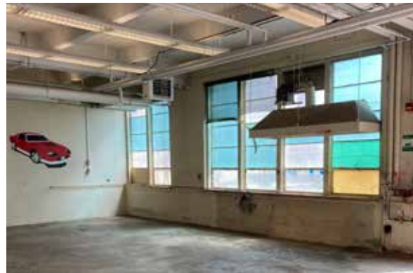
Fig. 115. Infilled window panes.
