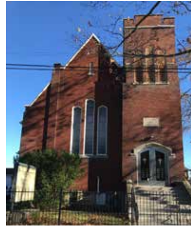
West elevation - 15 Wexford Avenue (ERA, 2022).
