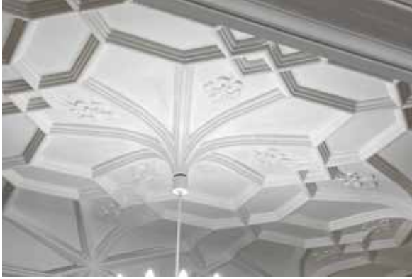
Fig. 94. Main lobby plaster ceiling.
