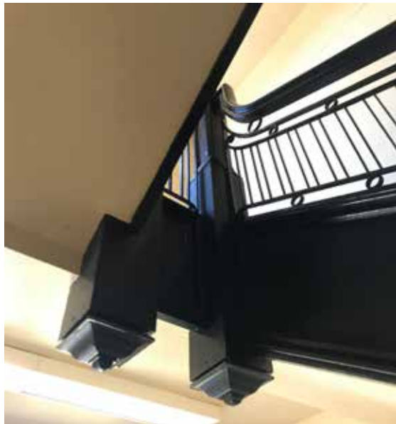
Stairway landing newel posts from below.
