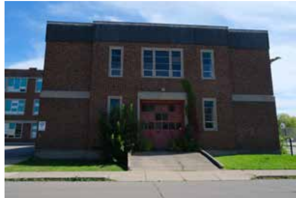
Fig. 114. South Back Wing facade.
