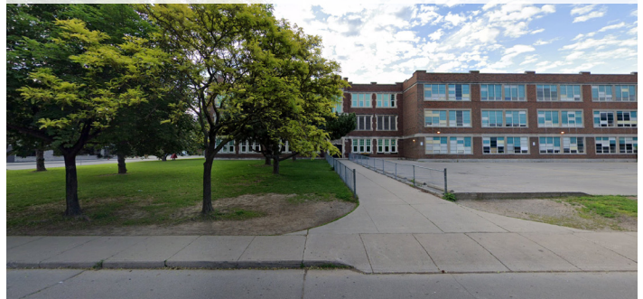
Concrete Walk from Graham Avenue S. to Entrance
