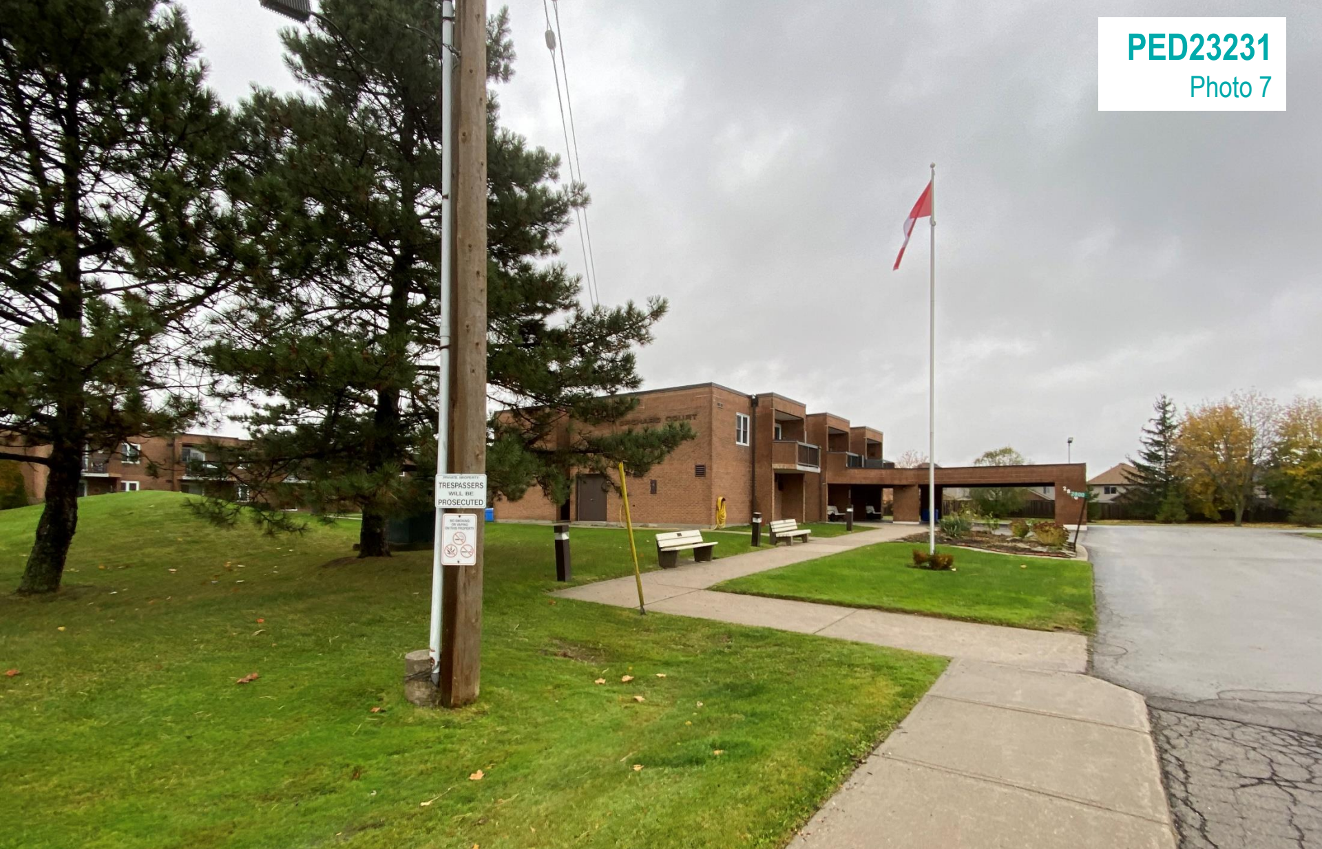
View of existing orchard court seniors residence
