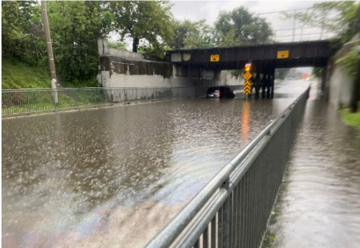
August 2023 storm – flooding on Birch Avenue
