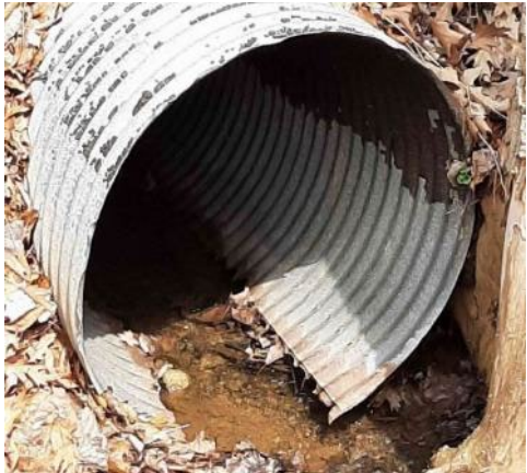
Damaged outfall
