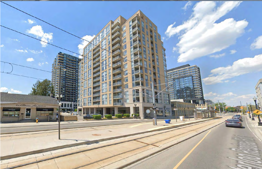
Figure 26: Precedent: 191 King St S, Waterloo ON
