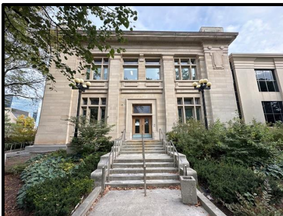
Image 3: Detailed View of West Elevation (October 18, 2023; Facing East)
