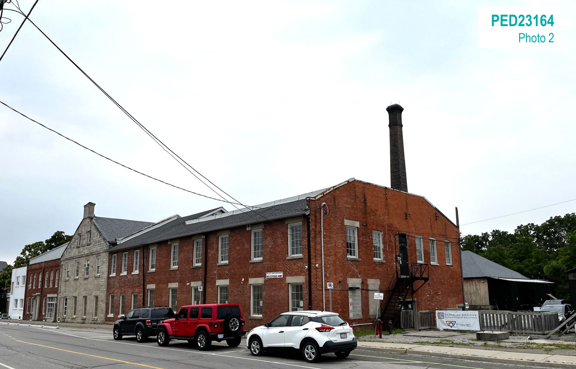
Looking south east at the subject property, from Hatt St
