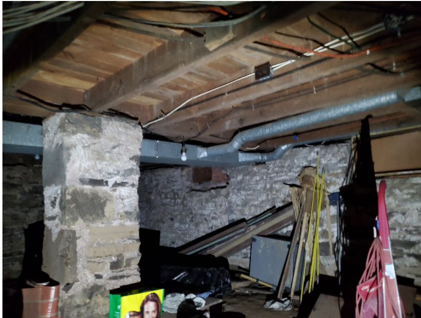
Photo No 03: Main Floor Framing (Original House)
