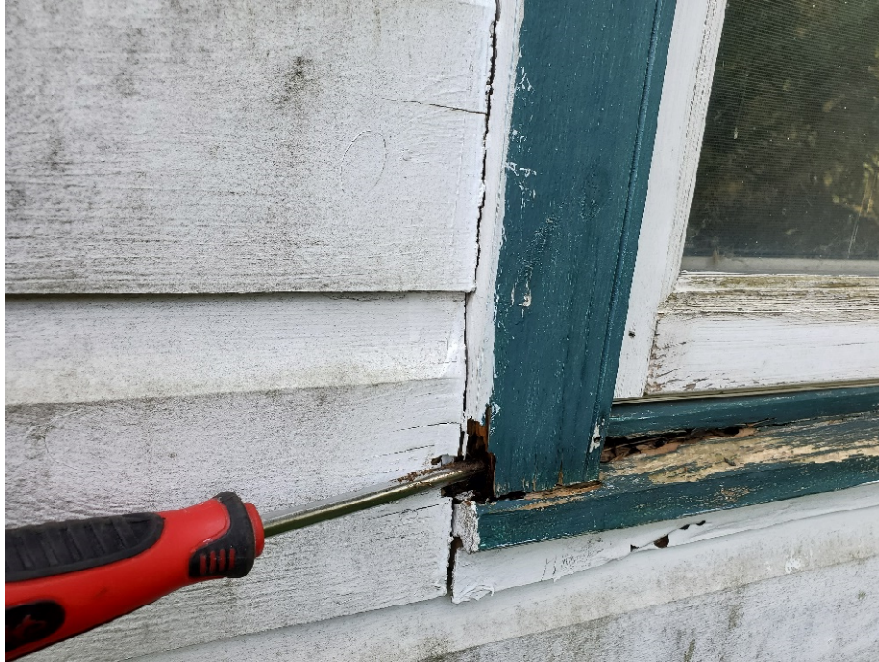
Photo No 07: Rotted Sill
