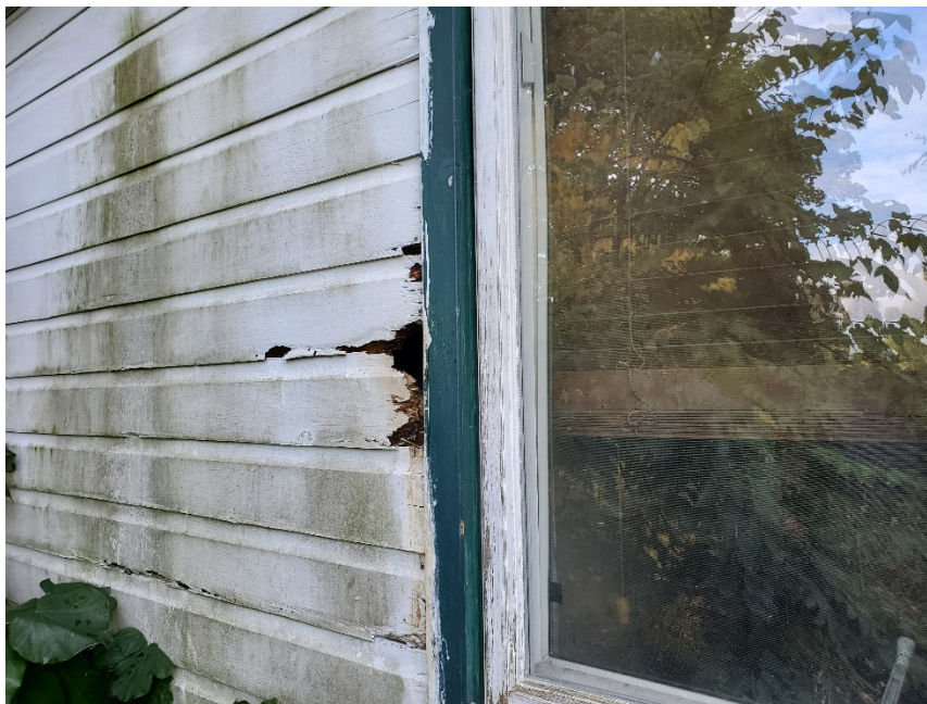
Photo No 06: Rotted Siding
