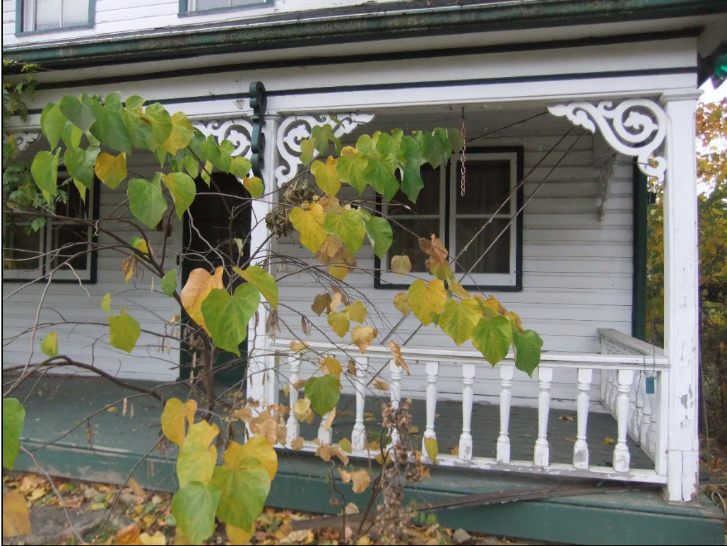
Figure 19: View of front porch with posts, scroll work and railings
