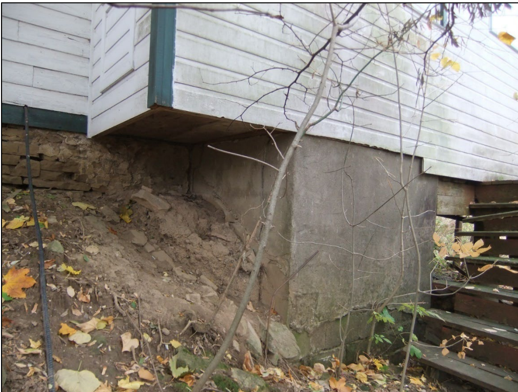
Figure 12: View of contemporary side addition and foundation
