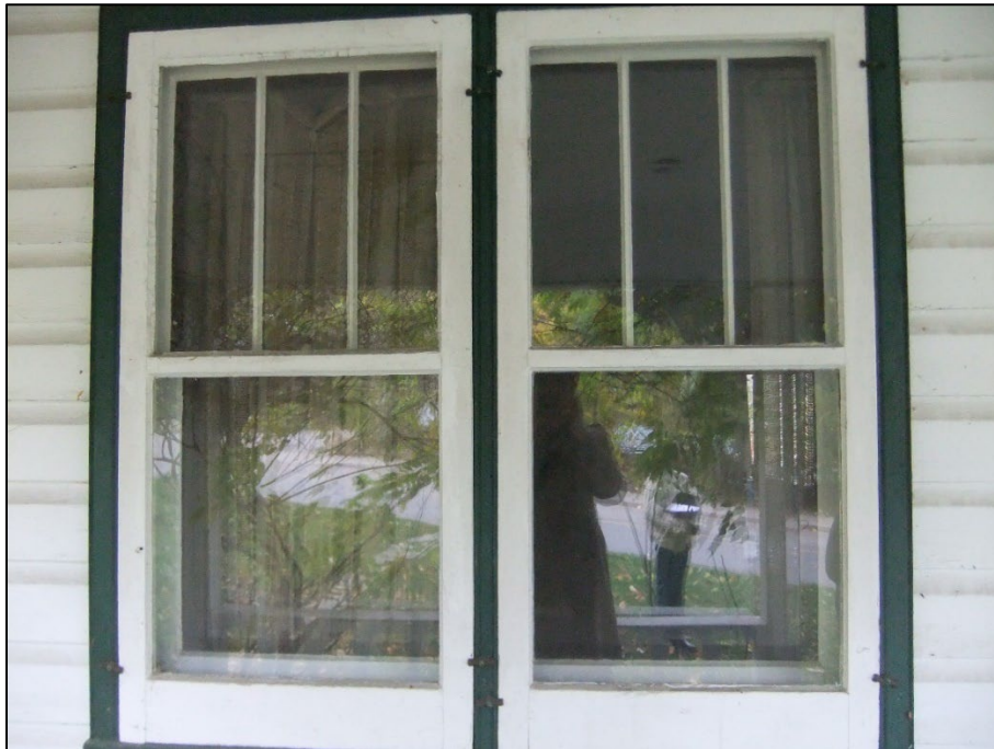
Figure 18: Early twentieth-century windows on front exterior
