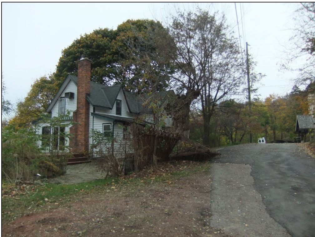
Figure 2: View of South Elevation along Ontario Road
