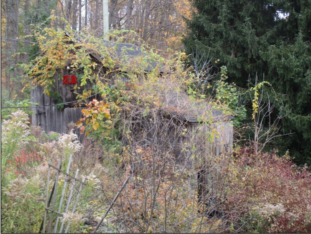
Figure 3: View of Two Level Shed in rear yard
