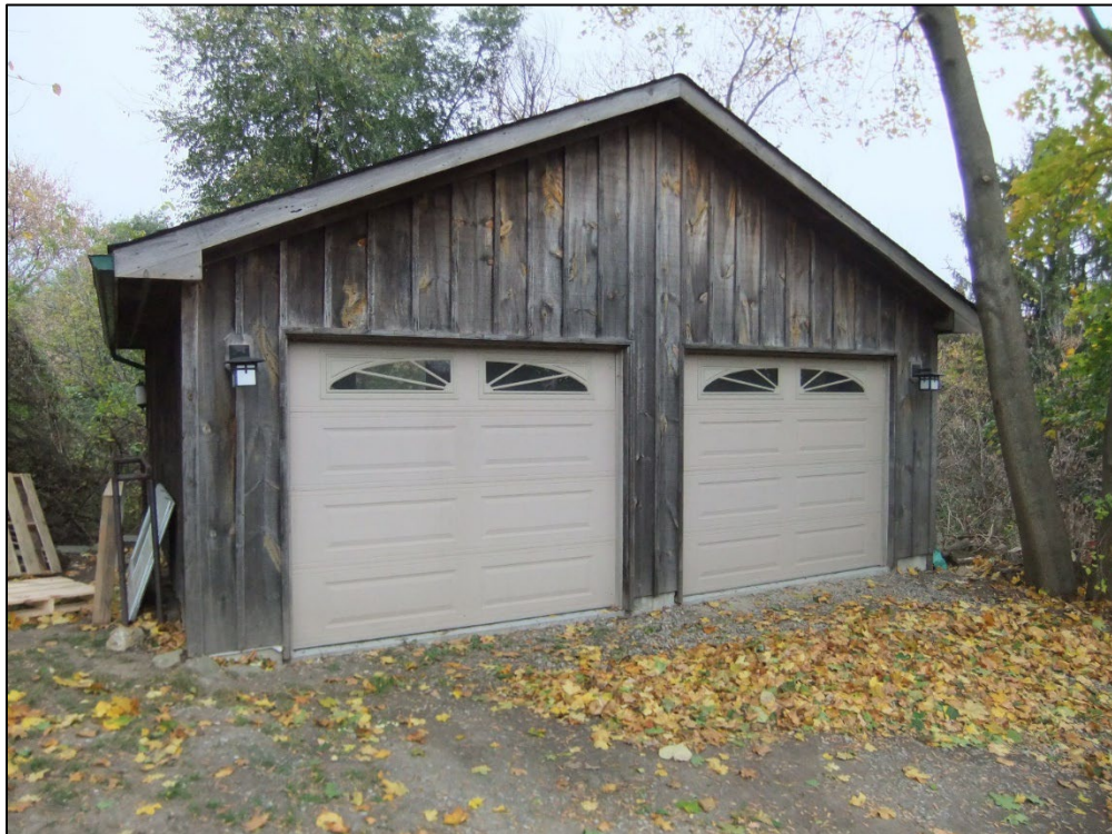
Figure 4: View of existing contemporary side garage
